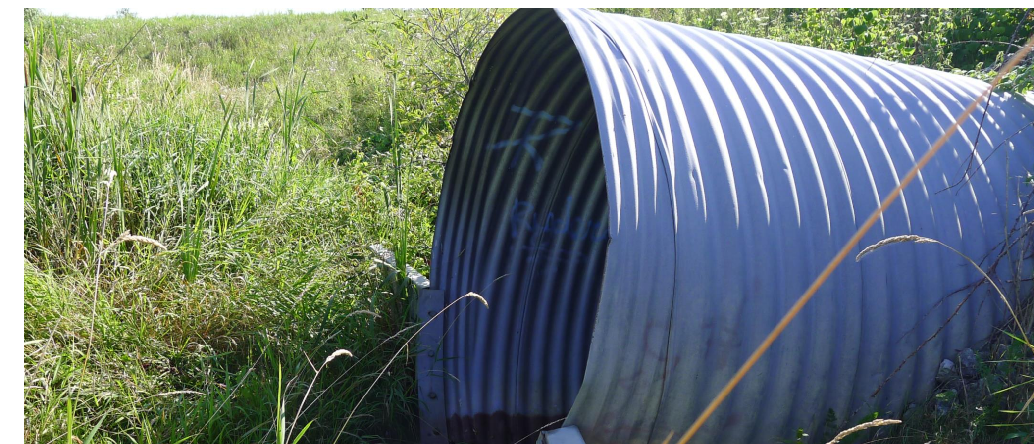
2-meter diameter CSP culvert
