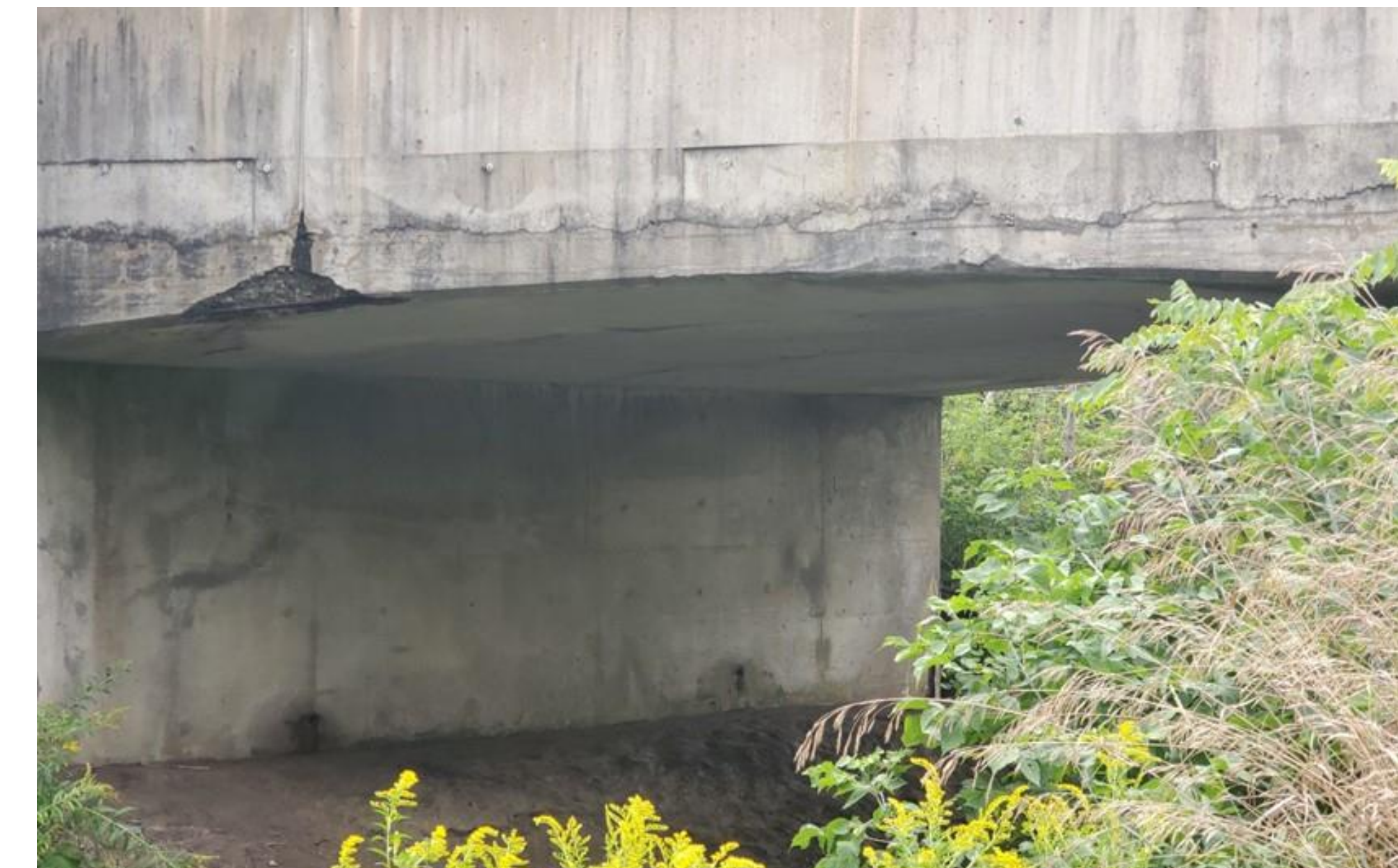
Soffit of bridge looking north to be repaired
