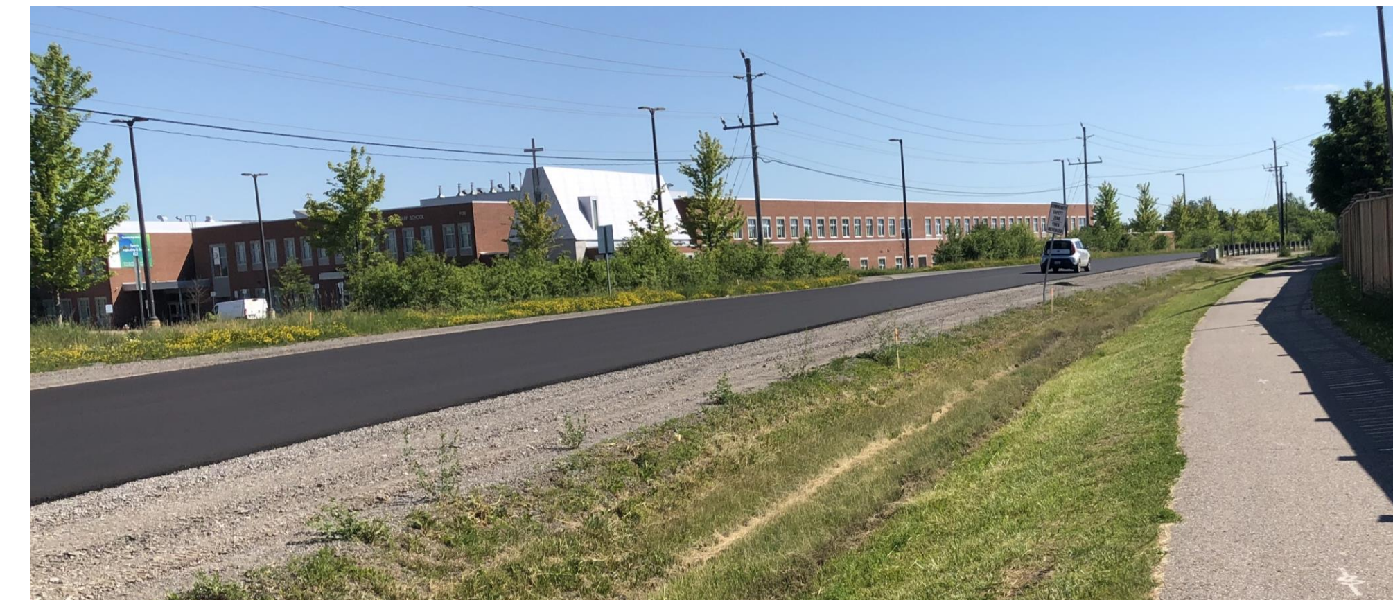
Shoulder in front of school being utilized for student pick-up & drop-off
