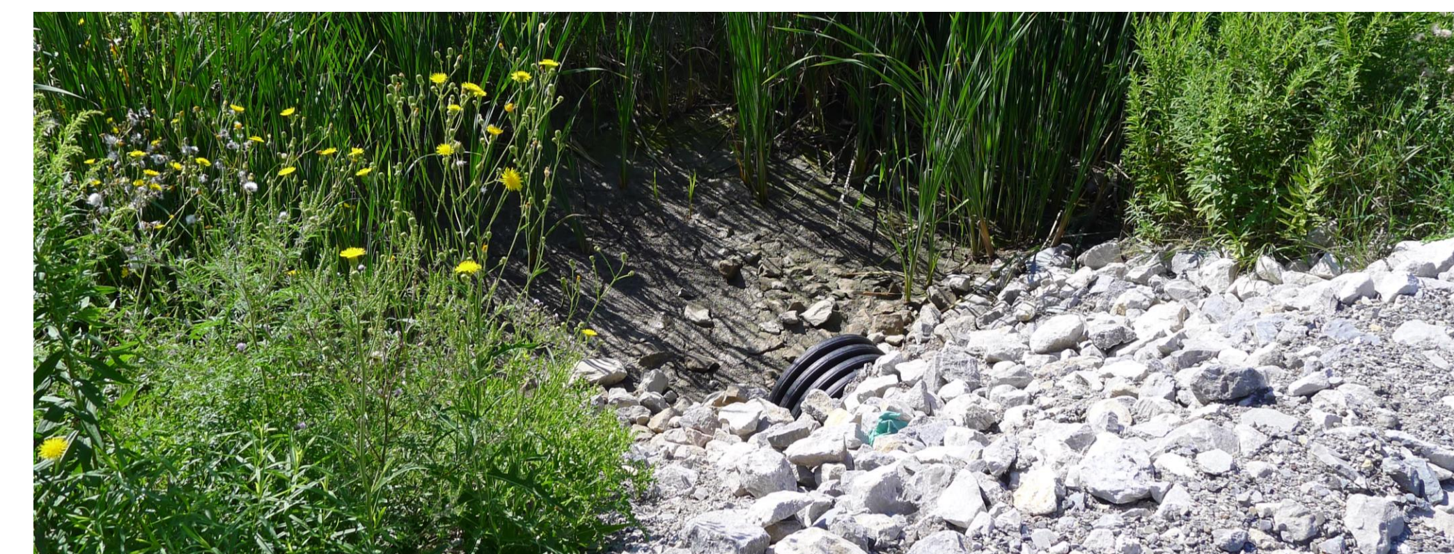
Recently upsized culvert in area 9706 Columbia Way
