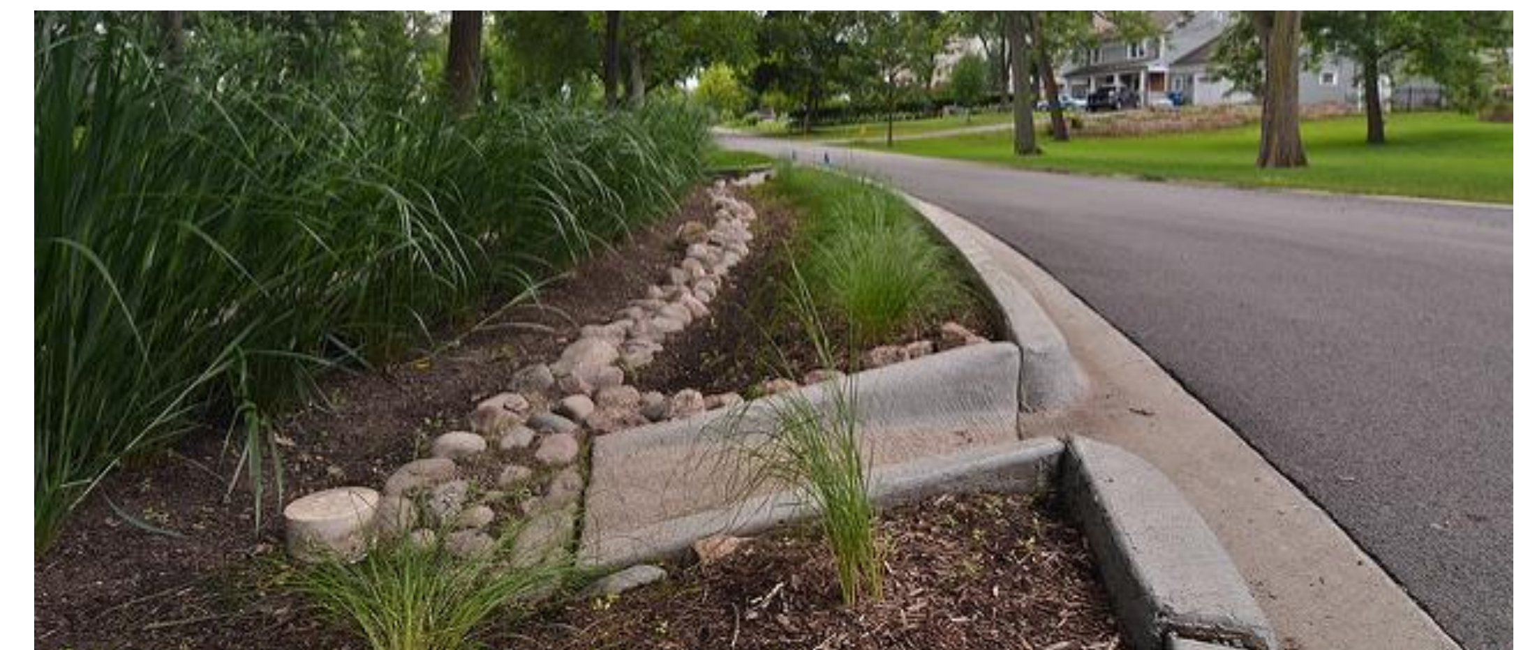
Example of rip rap installed at curb cutout inlet to dissipate power and reduce erosion. Photo credit: CNT.
