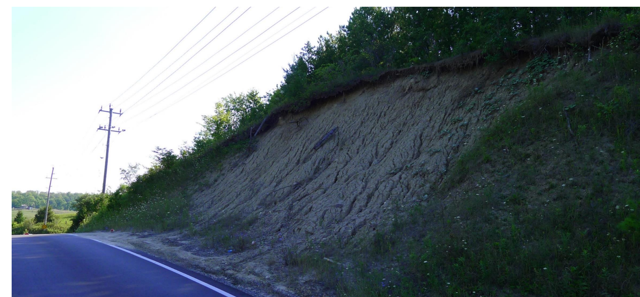
Bank washout onto roadway at cut slope west of Caledon King Townline
