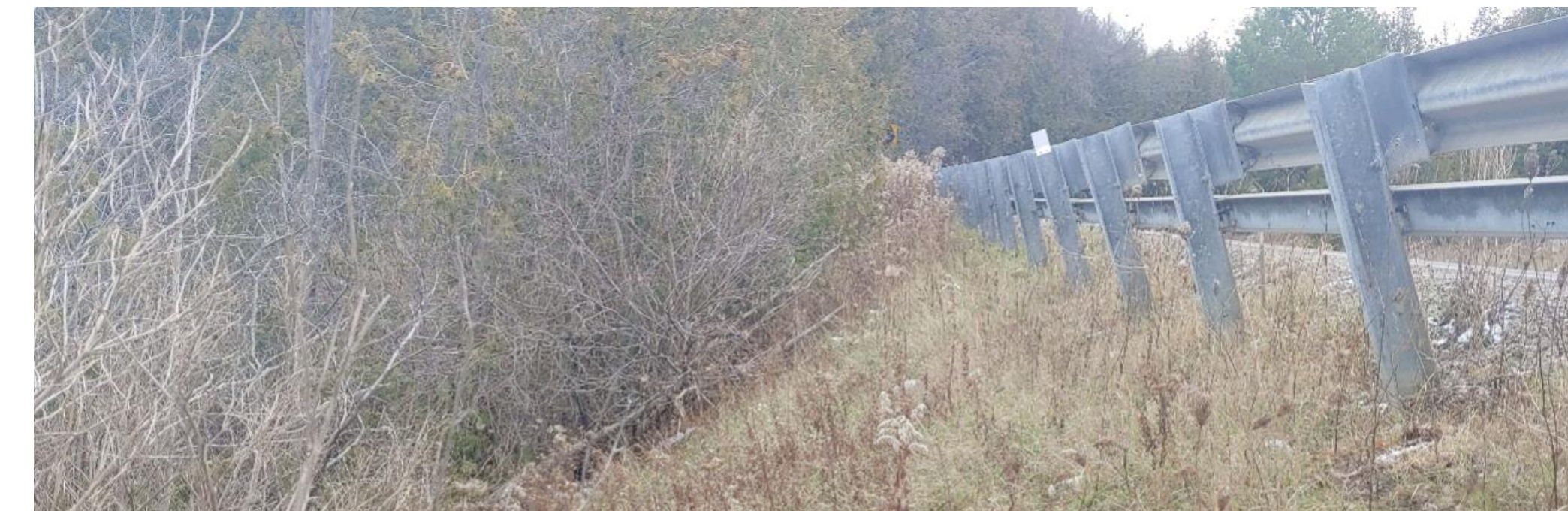
Guardrail and downslope at slope east of Forest Gate Avenue
