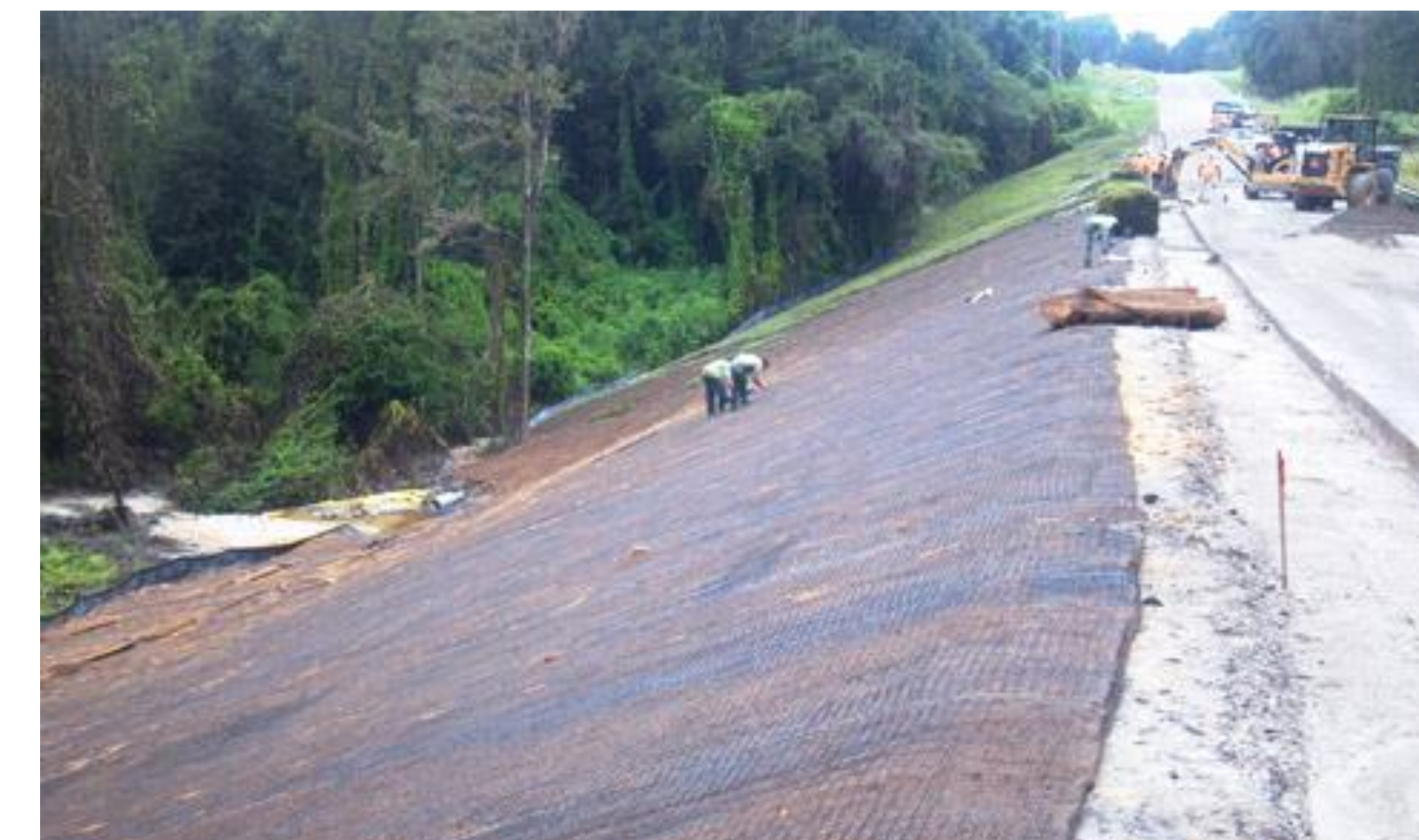
Example Geotextile mat to secure re-established slope
