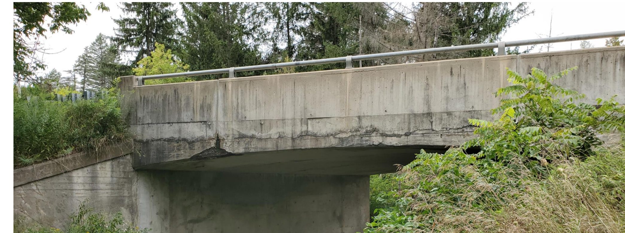
Coventry Bridge Structure
