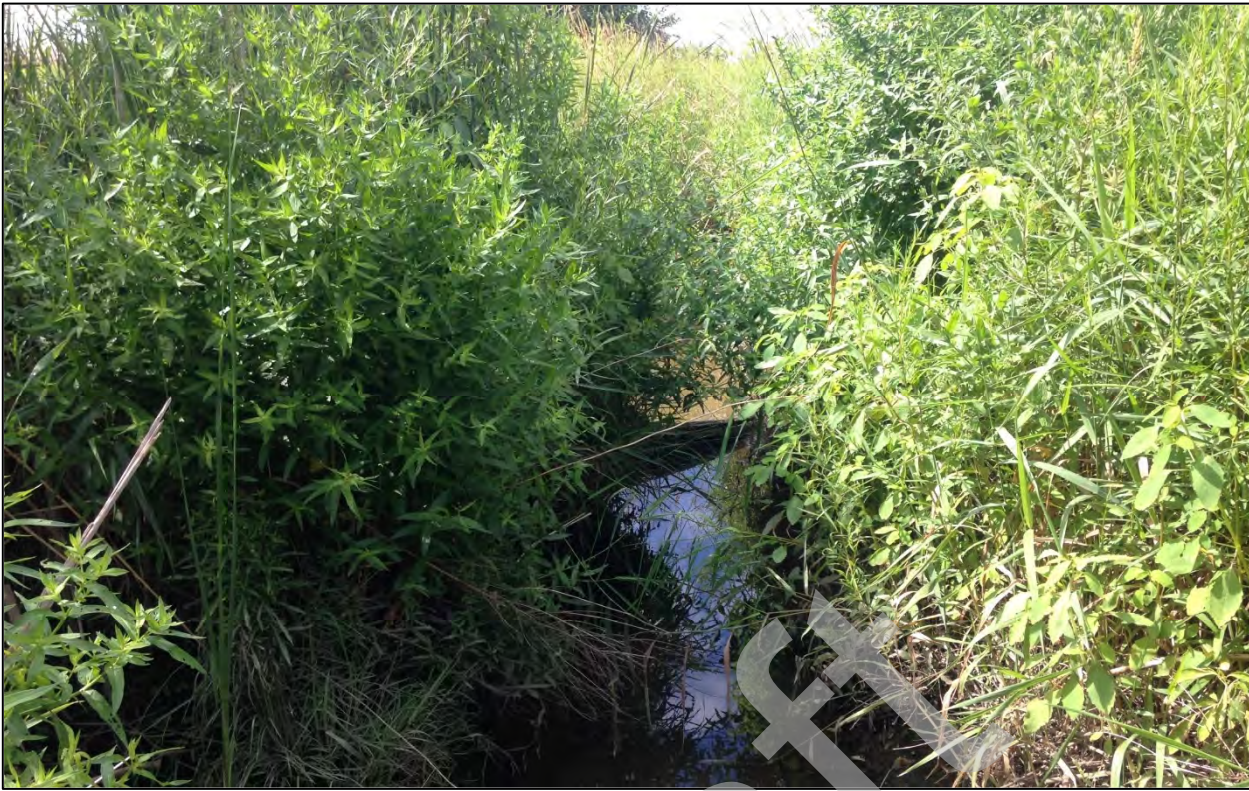
Photo 10: The low-flow channel in SWMF #16 within an open herbaceous marshy area of the facility.
