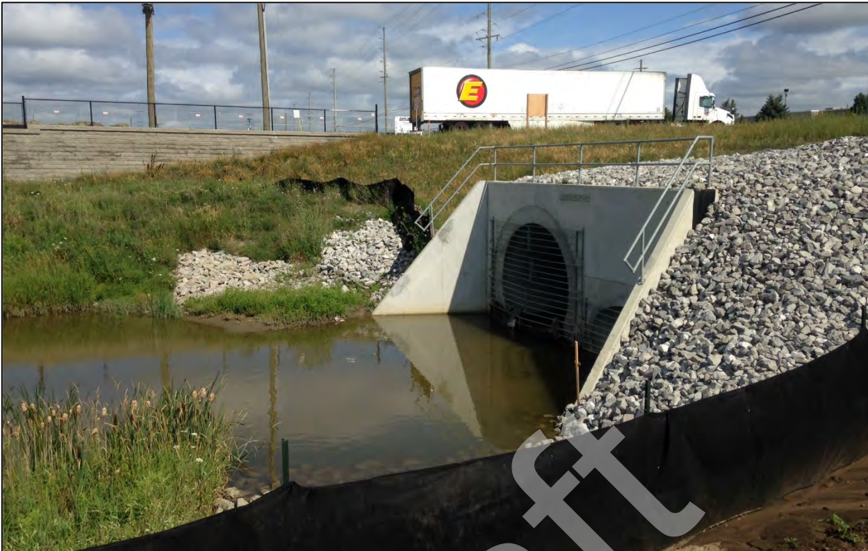
Photo 9: The outlet of the piped watercourse enclosure more than 800 metres downstream of the SWMF #16 outlet.
