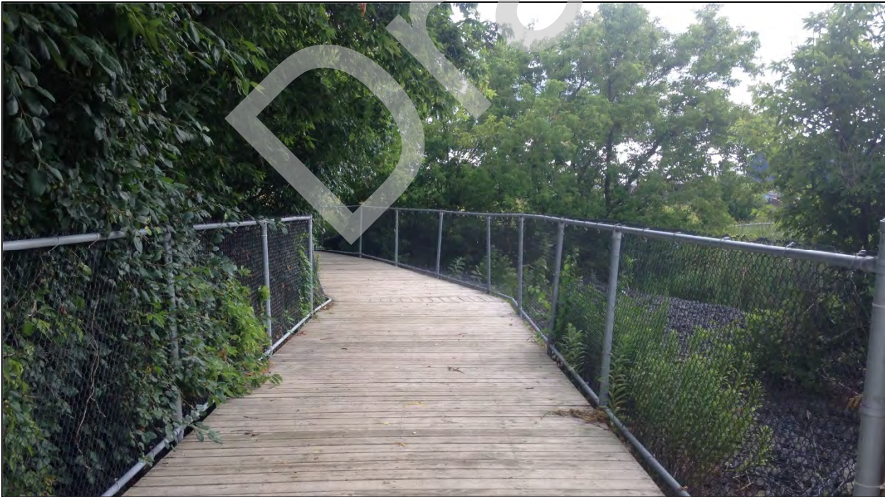
Photo 6: The fenced boardwalk over the SWMF #16 “dam” and outlet connects the manicured and semi-manicured portions of the leash-free dog park.
