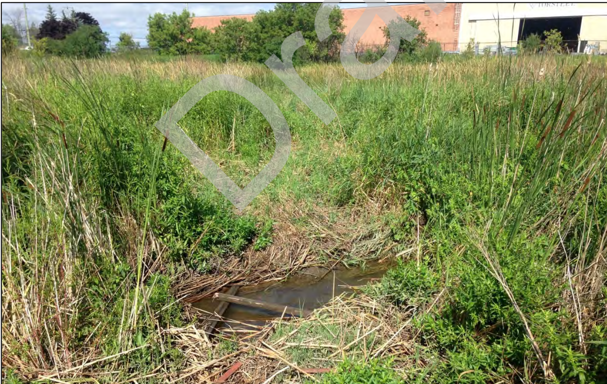
Photo 4: Tiny low-flow channel (foreground) within the Cattail stand in the centre of the SWMF #16 basin, made temporarily visible in this location where traverse of a tracked drill rig had knocked down a trail through the Cattail stand vegetation.
