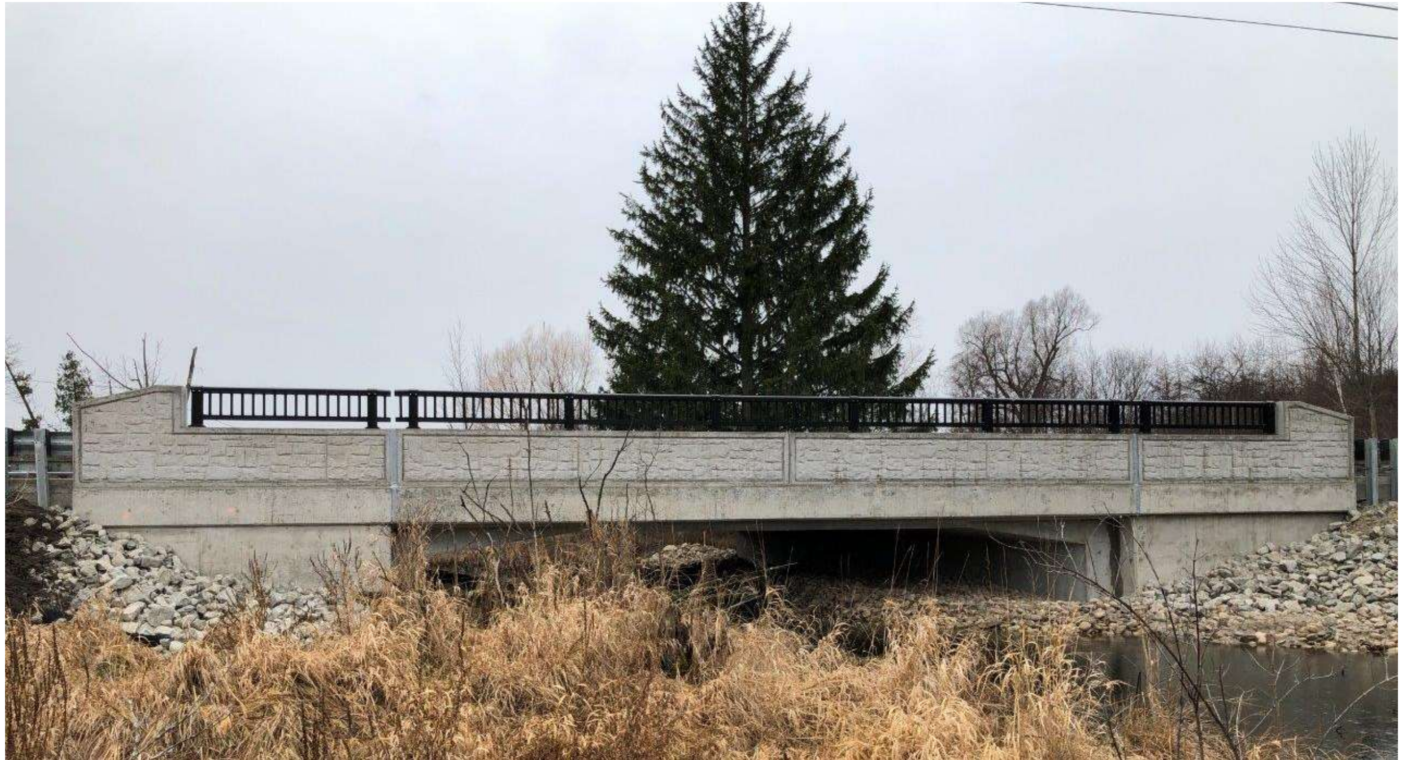
Figure 6.6 - Example Bridge Barrier Style (Main Street Bridge Preferred Design Concept)
