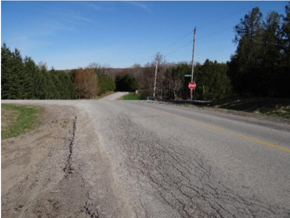
Plate 1: SE view Main St and Highpoint Side Rd – Area west of disturbed road requires Stage 2 survey
