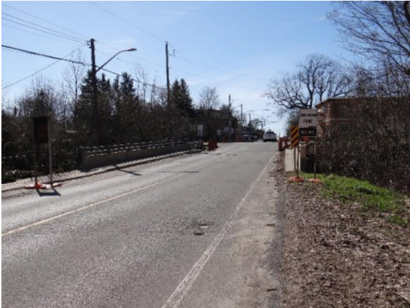
Plate 13: SE view Main St bridge – Area beyond disturbed road requires Stage 2 survey
