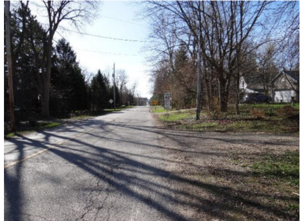
Plate 8: SE view Main St – Area beyond disturbed road requires Stage 2 survey
