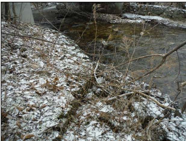
Shaw's Creek: Gabion basket bank treatments downstream of Main Street crossing.
