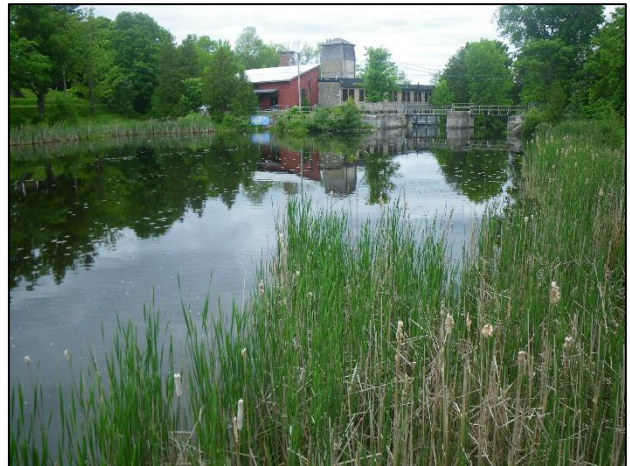
Shaw's Creek at Alton Mill Pond: facing downstream (east) at dam.
