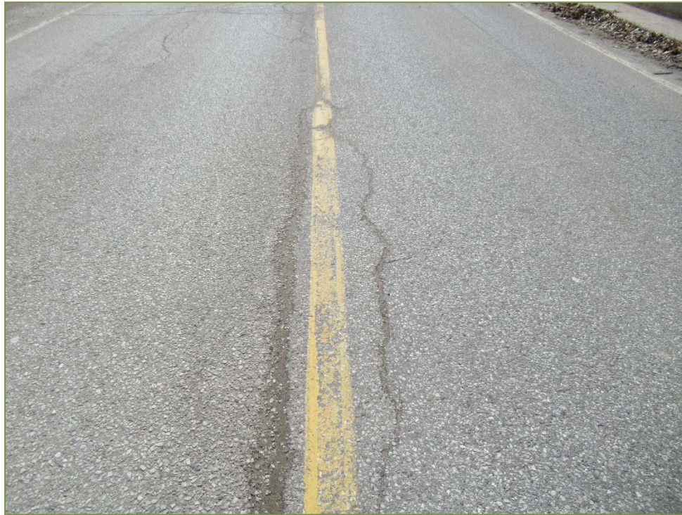
Photo P5 – Deck Wearing Surface (fair condition – unsealed cracks)
