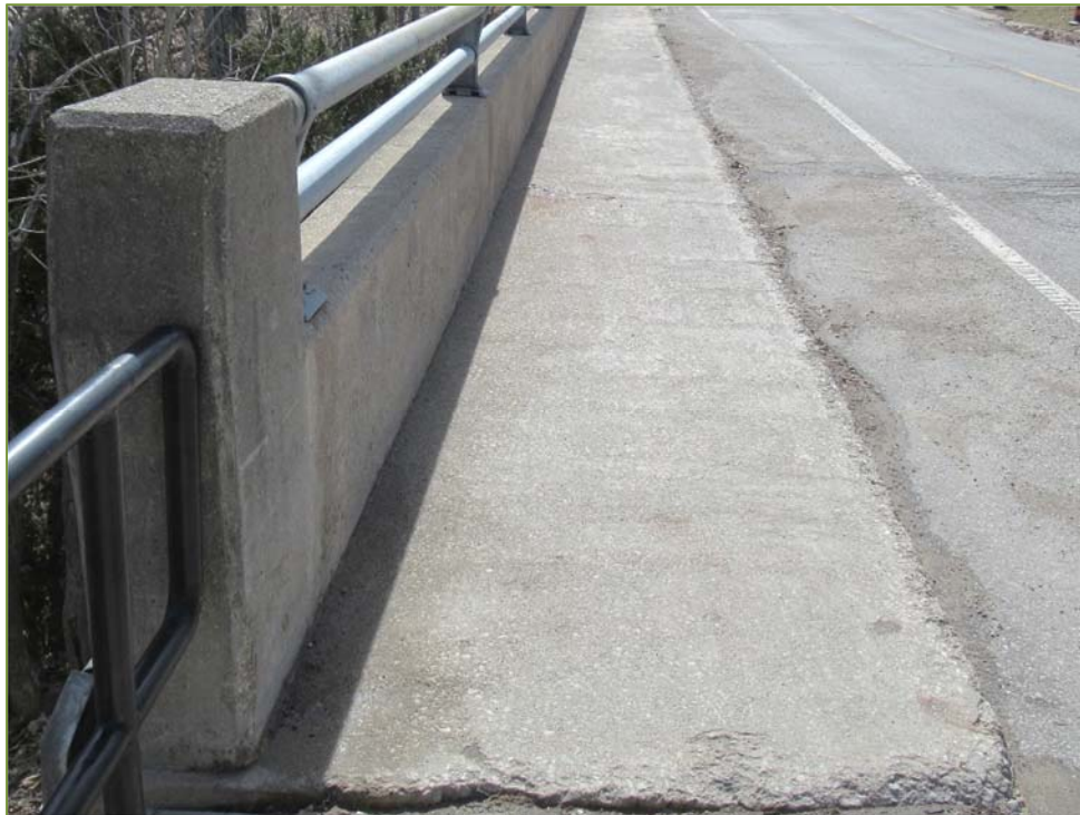
Photo P36 – Northeast End Post (fair to good condition – light scaling)
