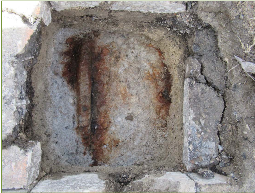
Photo S5 – Sawn Sample SS5 (disintegration) note exposed and corroded rebar
