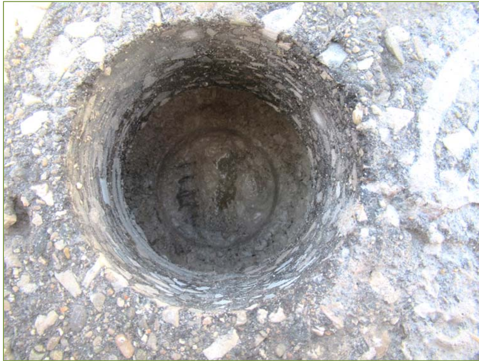
Photo P65 – Typical Condition of Inside Core – C8 (disintegration)
