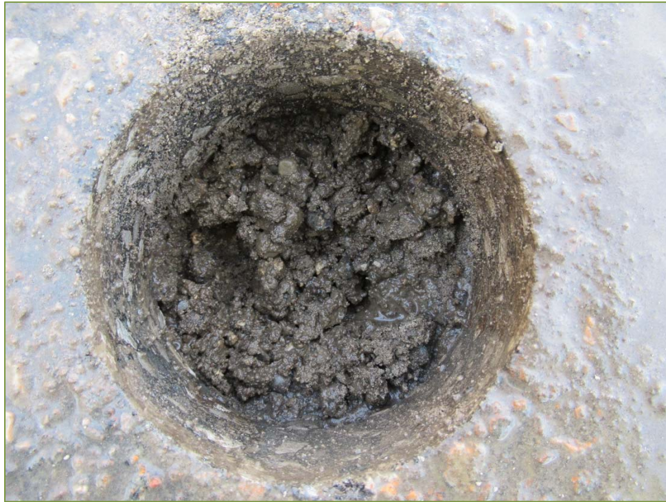
Photo P61 – Typical Condition of Inside Core – C1 (north approach; granular)
