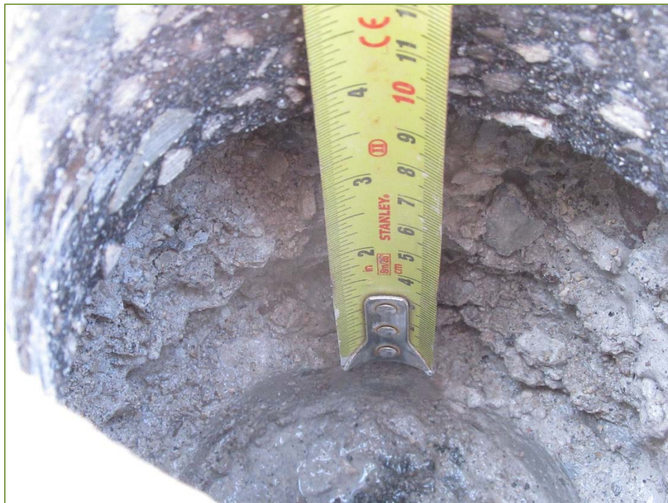
Photo P66 – Typical Condition of Inside Core – C8 (disintegration)
