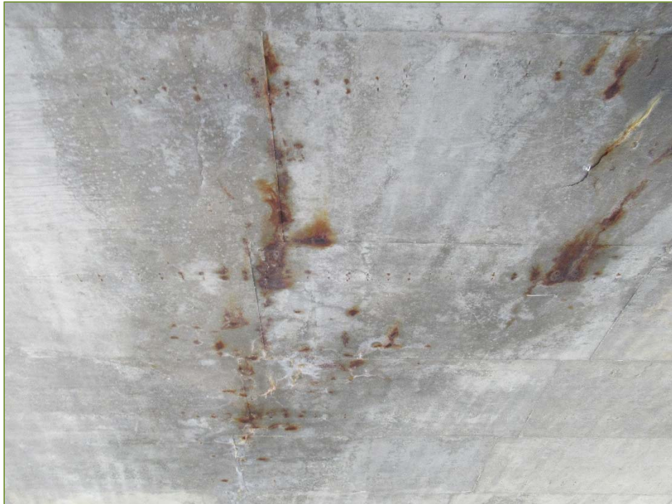
Photo P12 – Soffit (cracks, delamination and wet area)
