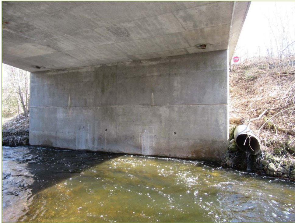
Photo P45 – South Abutment (good condition – cracks)
