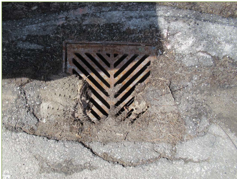
Photo P22 – Northwest Catch Basin
