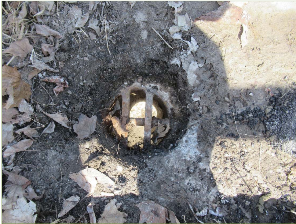
Photo P17 – Northeast Deck Drainage
