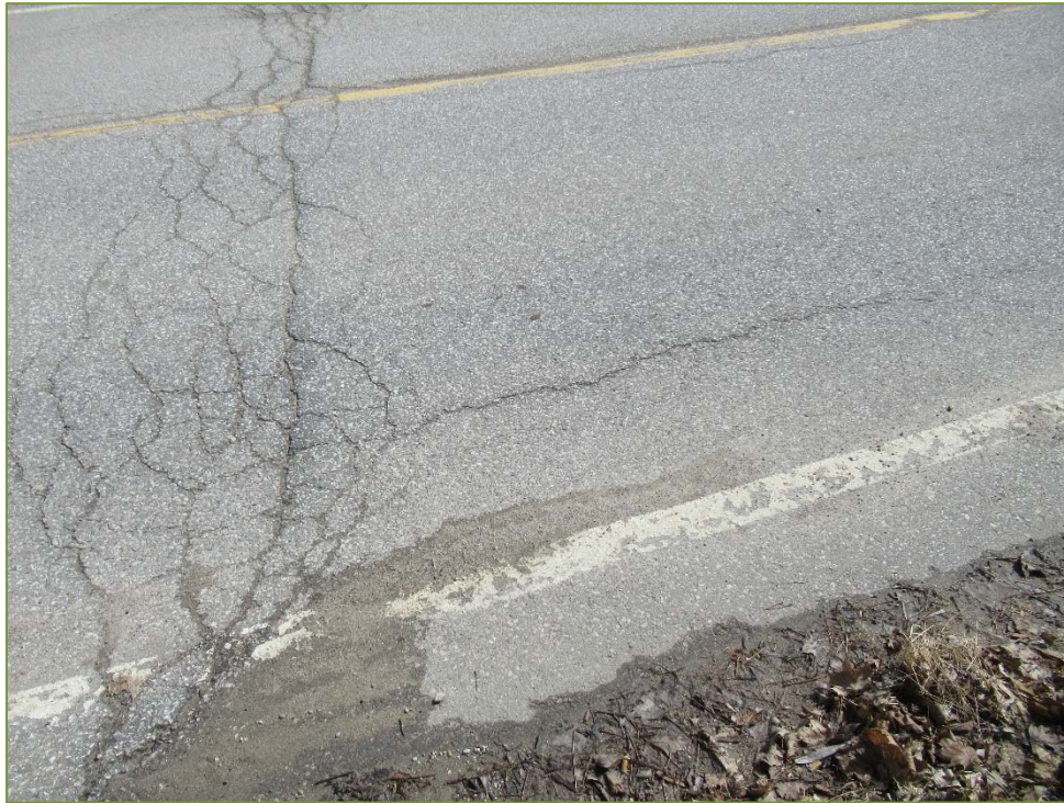
Photo P7 – Deck Wearing Surface (unsealed cracks)
