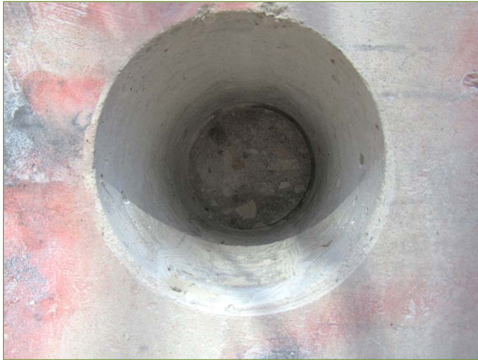
Photo P73 – Typical Condition of Inside Core – C18 (Northwest wingwall)
