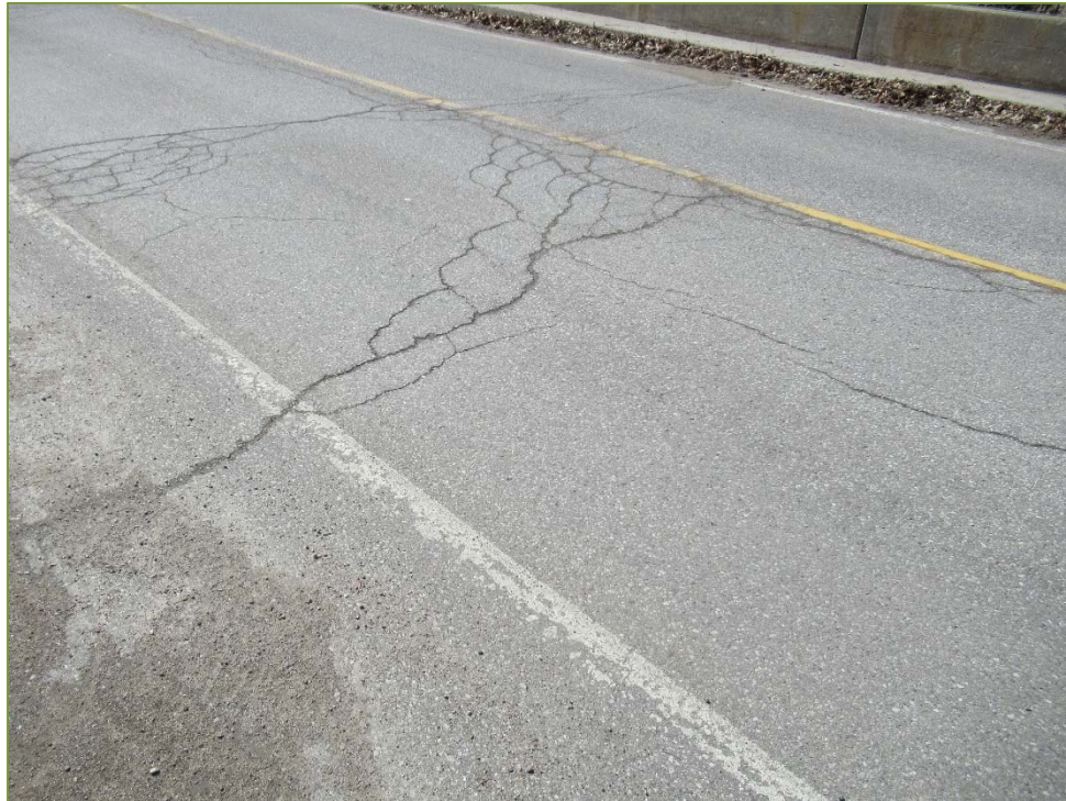
Photo P6 – Deck Wearing Surface (unsealed cracks)
