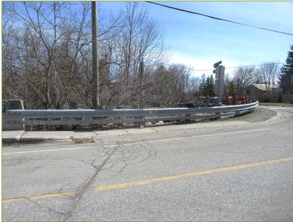
Photo P41 – Southeast Guiderail (good condition)
