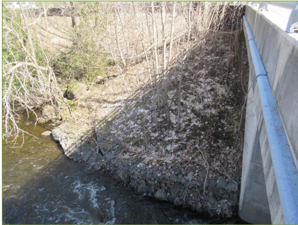
Photo P59 – Southeast Embankment (fair to good condition – soil erosion)
