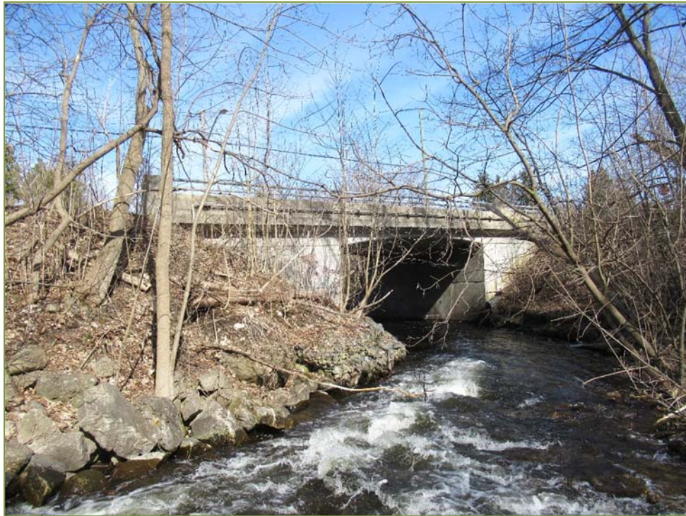
Photo P2 – West Elevation
