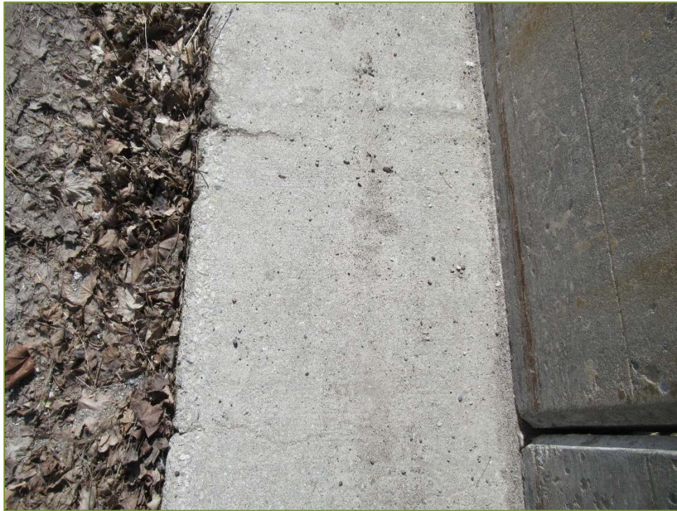
Photo P35 – West Curb (crack and medium scaling)
