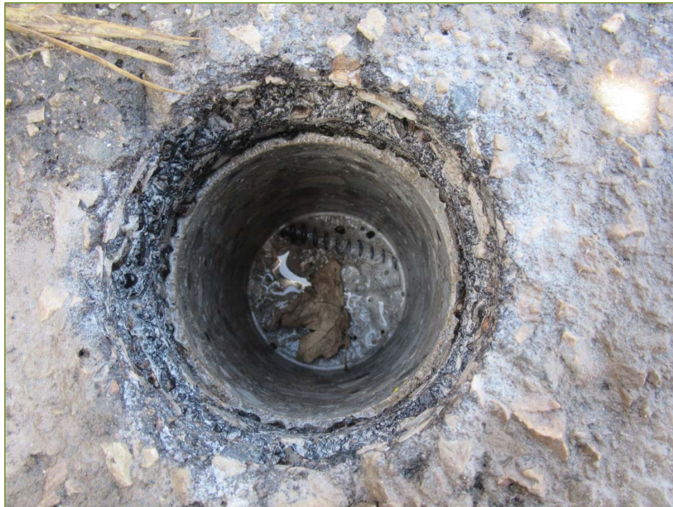
Photo P62 – Typical Condition of Inside Core – C4
