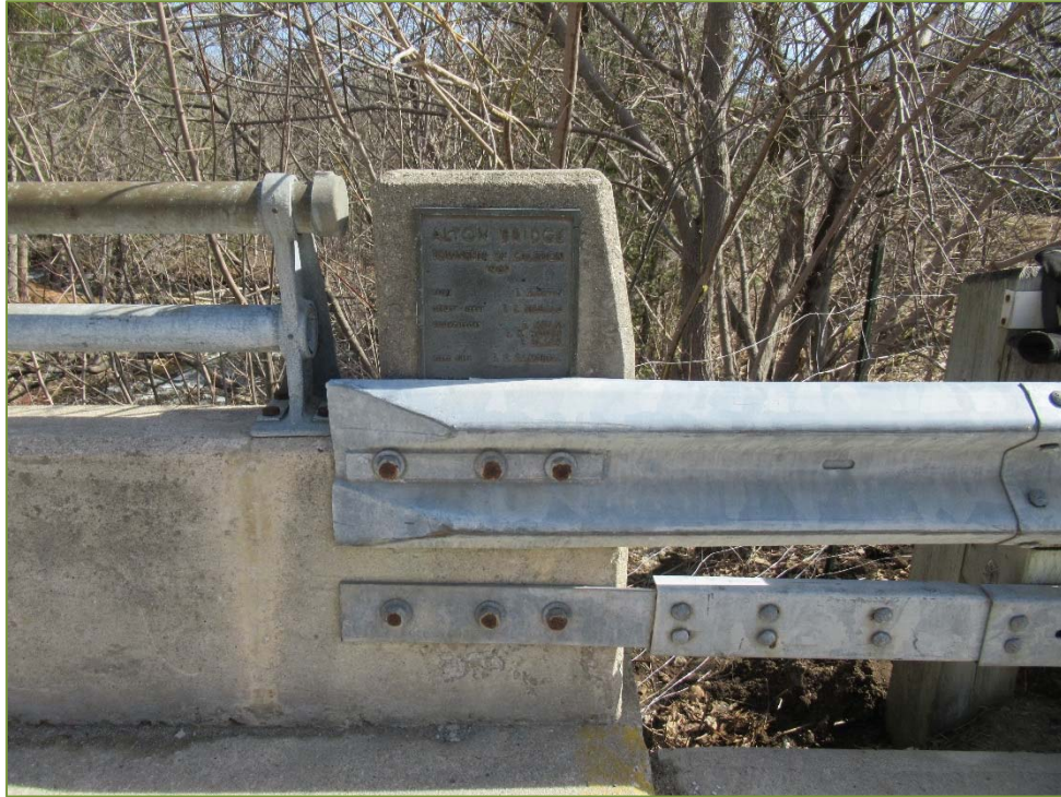
Photo P39 – Southeast End Post note missing handrail end cap
