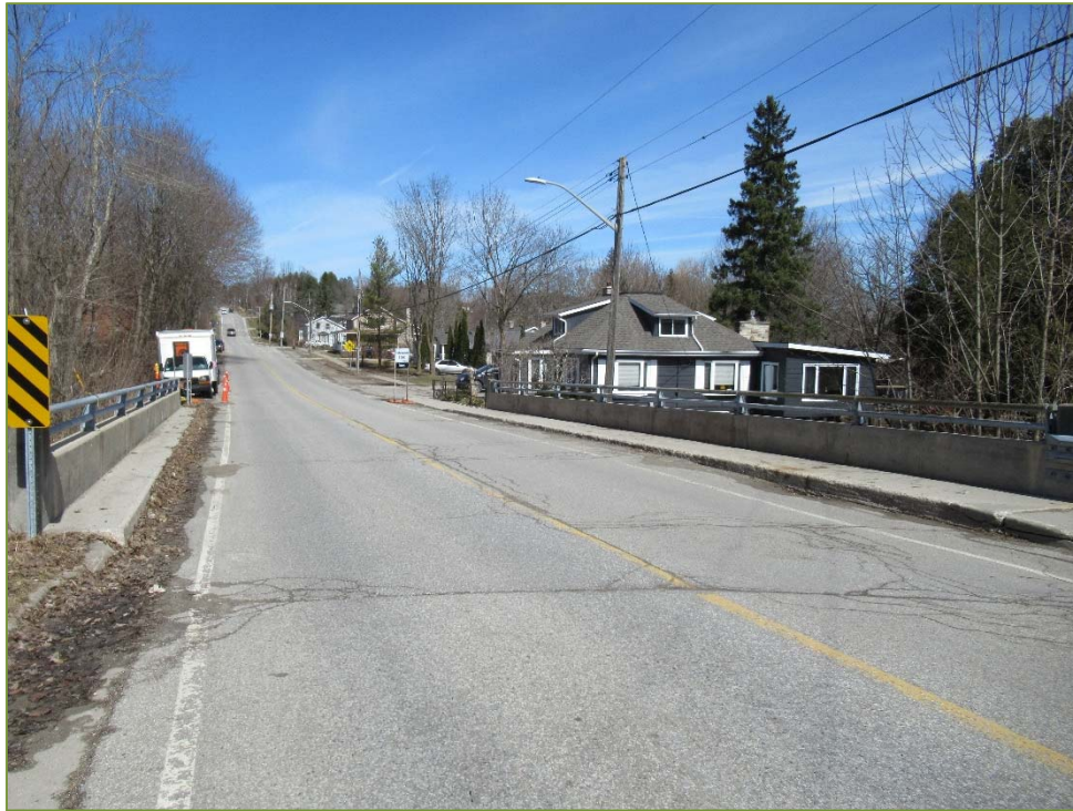
Photo P3 – Deck General View, looking north
