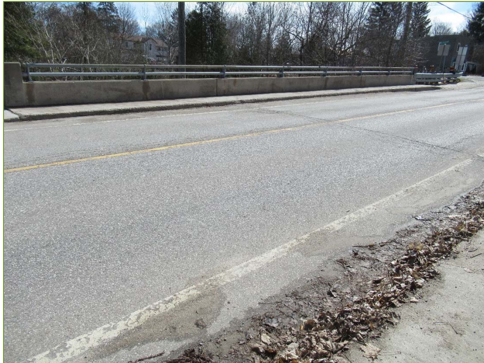
Photo P14 – North Approach Wearing Surface (fair condition – unsealed cracks) note settlement
