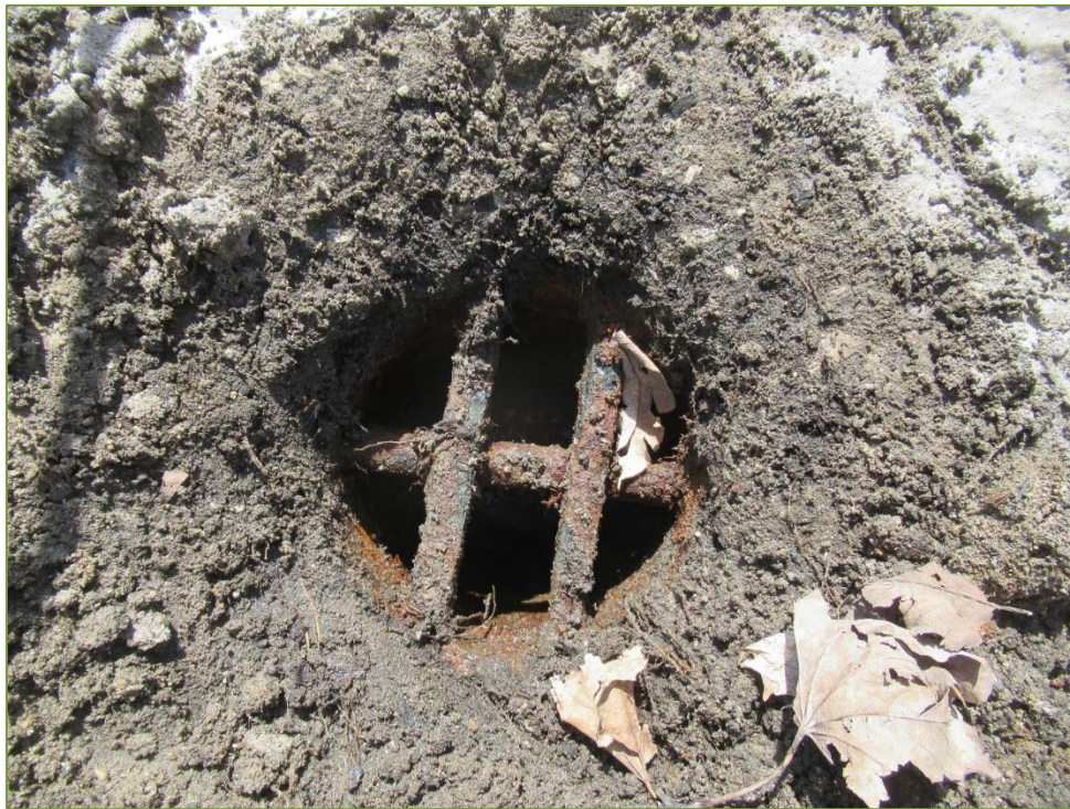
Photo P18 – Northwest Deck Drainage
