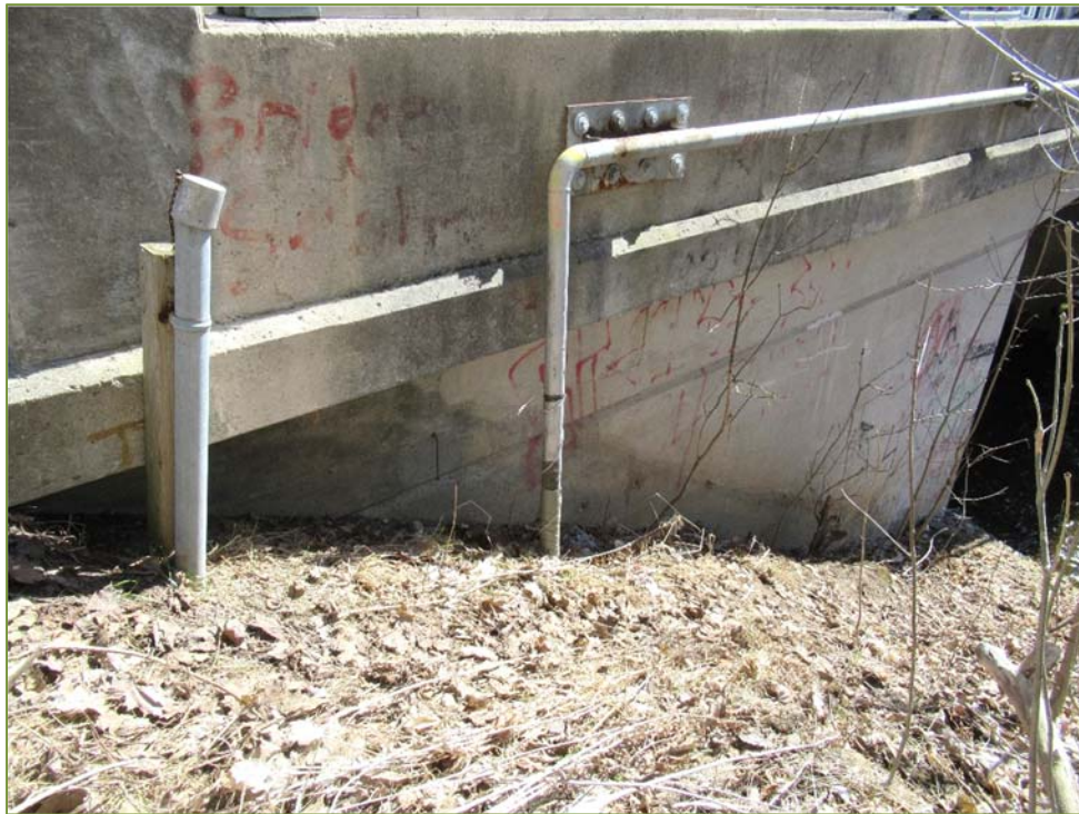
Photo P48 – Northwest Wingwall (good condition)
