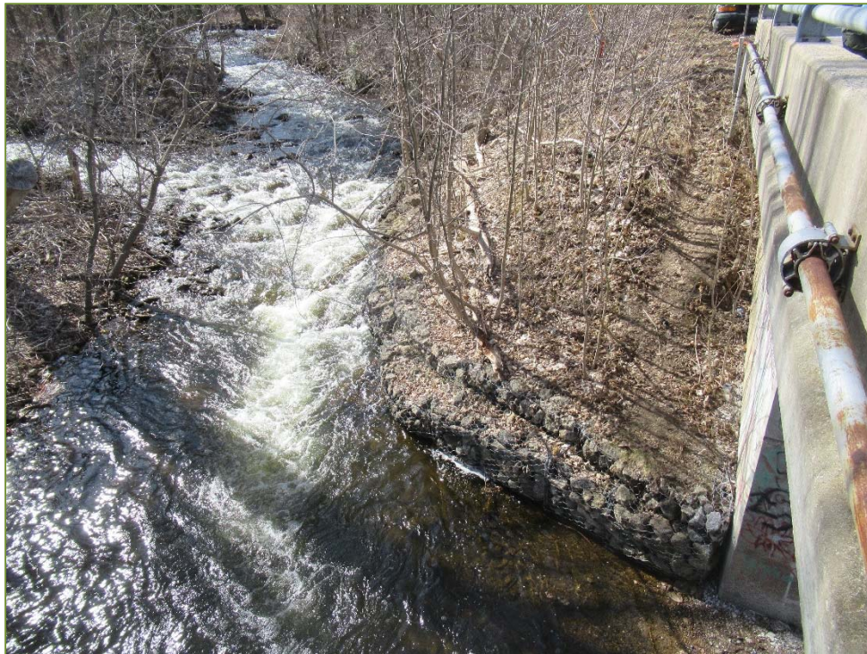
Photo P58 – Northwest Embankment (fair to good condition – soil erosion)
