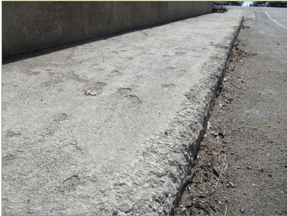
Photo P27 – East Sidewalk (light/medium scaling)
