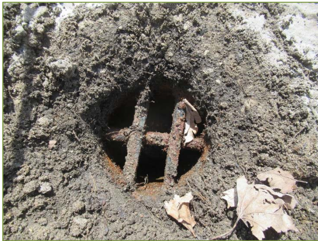
Typical Condition of Deck Drain @ Northwest
