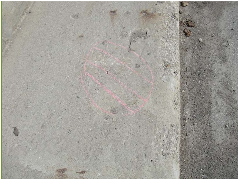
Photo P28 – East Sidewalk @ South Approach (spall, delamination and light/medium scaling)
