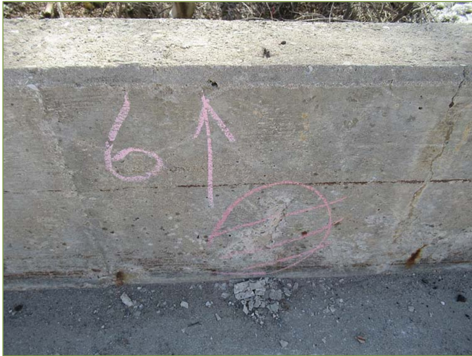
Photo P33 – West Parapet Wall (crack, spall and delamination)
