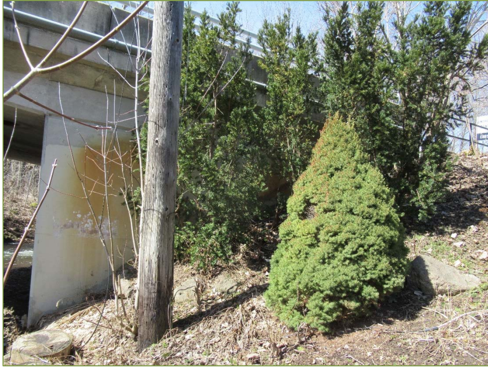
Photo P47 – Northeast Wingwall (good condition)
