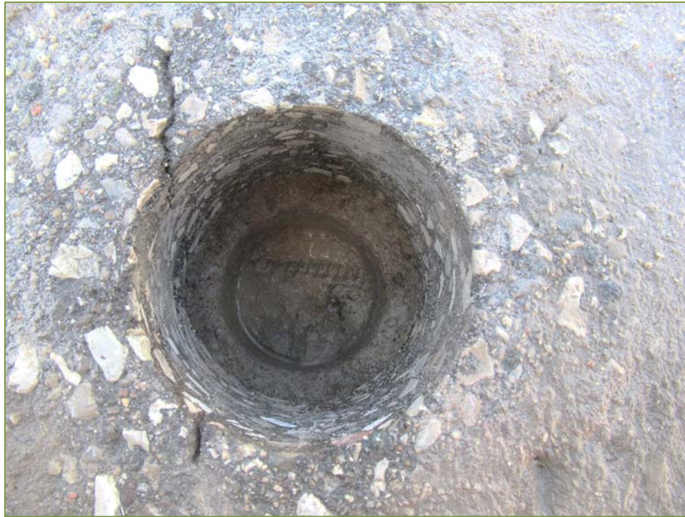
Photo P63 – Typical Condition of Inside Core – C6 (disintegration)
