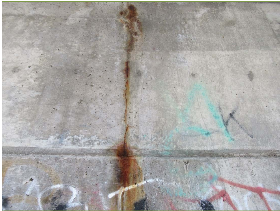
Photo P43 – North Abutment (wide crack and wet area)
