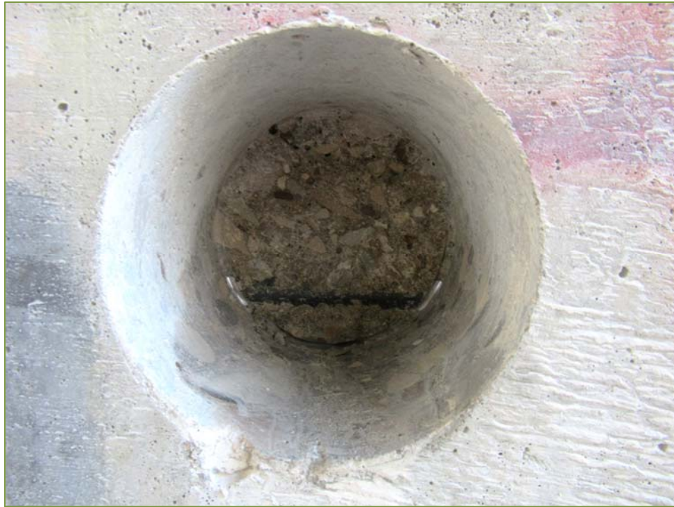
Photo P71 – Typical Condition of Inside Core – C13 (north abutment)
