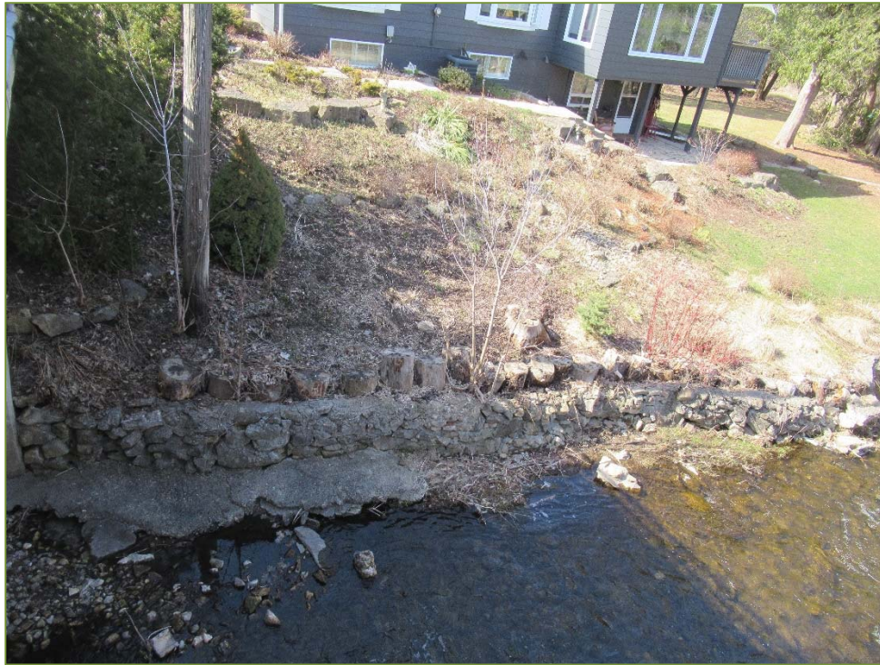
Photo P57 – Northeast Embankment (fair to good condition – soil erosion)
