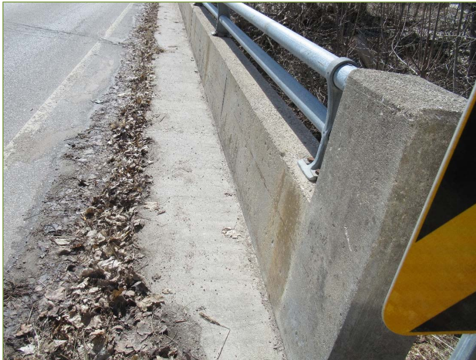
Photo P38 – Northwest End Post (good condition)
