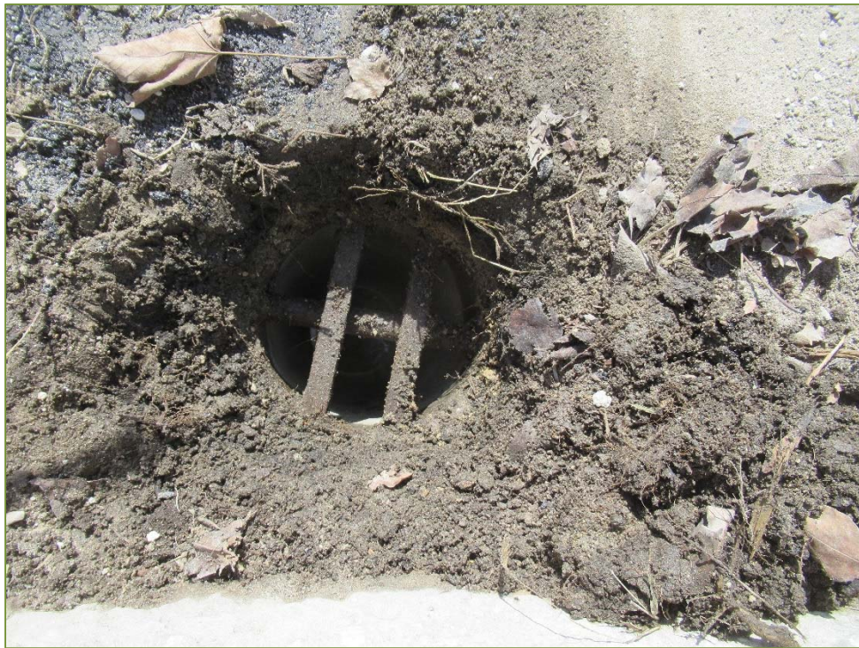
Photo P20 – Southwest Deck Drainage
