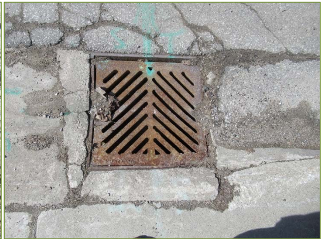
Typical Condition of Catch Basin @ Southeast
