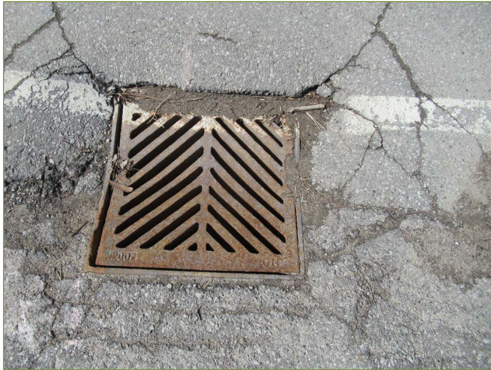
Photo P21 – Northeast Catch Basin
