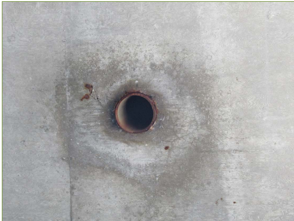
Photo P10 – Soffit at North Abutment, east edge (cracks, delamination and wet area) note medium corrosion on deck drain
