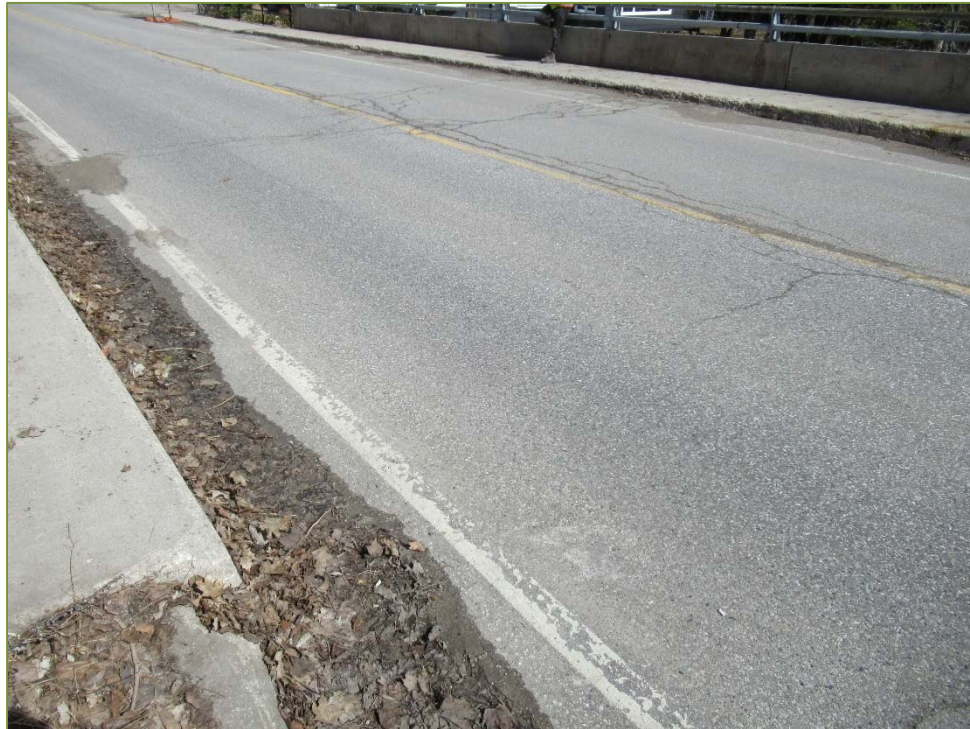
Photo P16 – South Approach Wearing Surface (fair to good condition – unsealed cracks)
