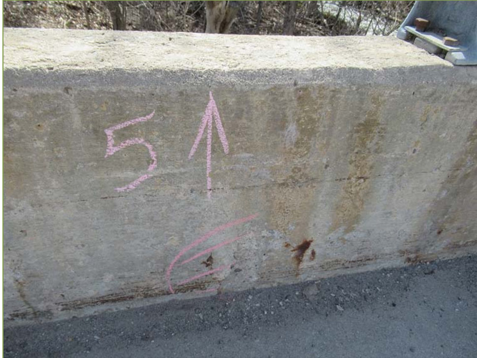
Photo P32 – West Parapet Wall (spall and delamination)
