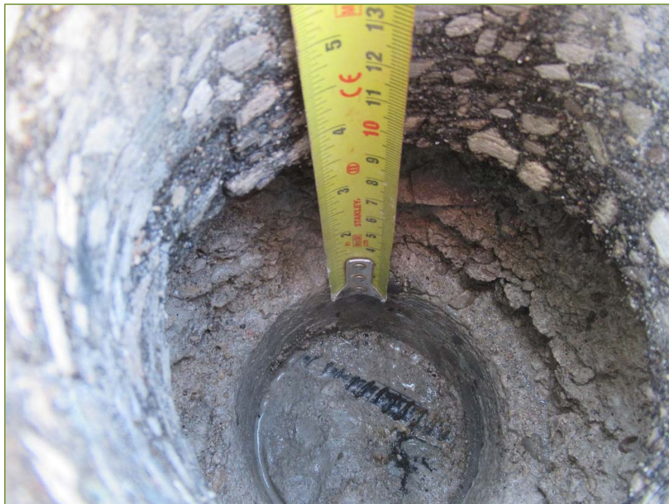
Photo P64 – Typical Condition of Inside Core – C6 (disintegration)
