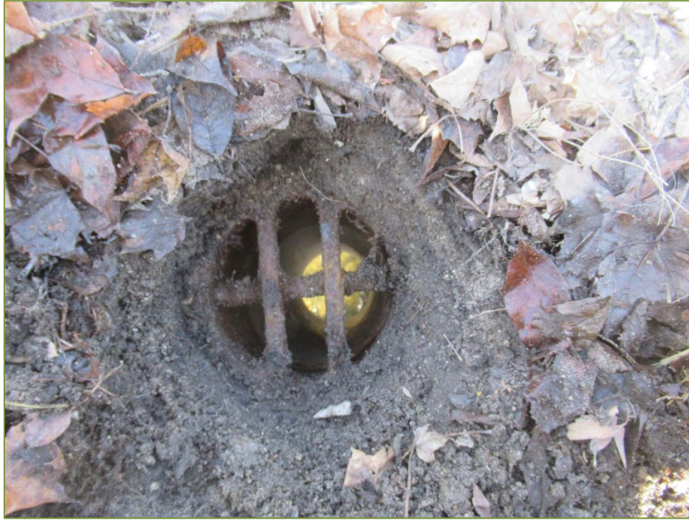
Photo P19 – Southeast Deck Drainage
