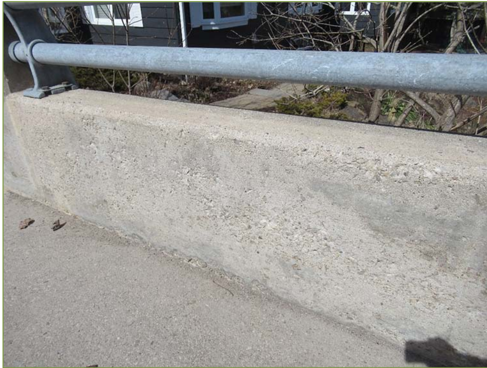
Photo P37 – Northeast End Post (light scaling)
