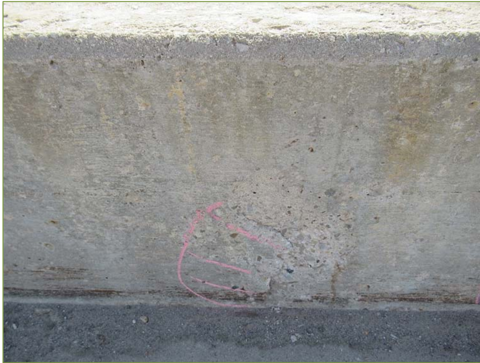
Photo P31 – West Parapet Wall (spall and delamination)
