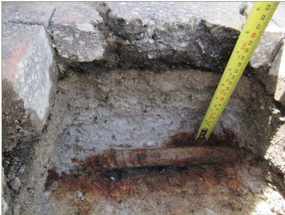
Photo S6 – Sawn Sample SS5 (disintegration) note exposed and corroded rebar
