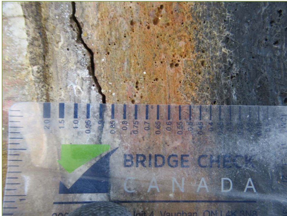
Photo P44 – North Abutment (wide crack and wet area)
