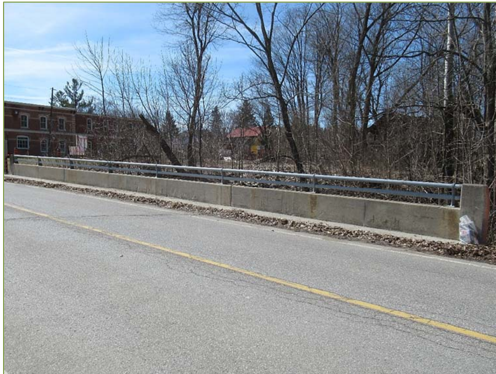
Photo P30 – West Curb (fair to good condition – cracks and medium scaling) and Parapet Wall (fair condition – cracks, spall and delamination)
