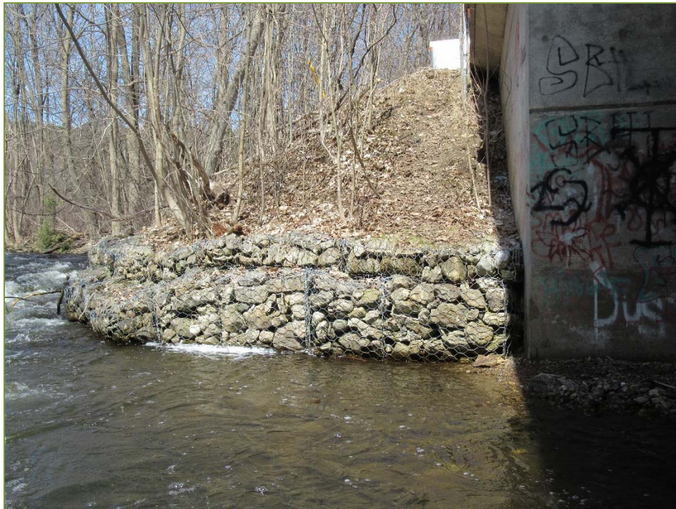
Photo P52 – Northwest Gabion Wall (fair to good condition – bulging)
