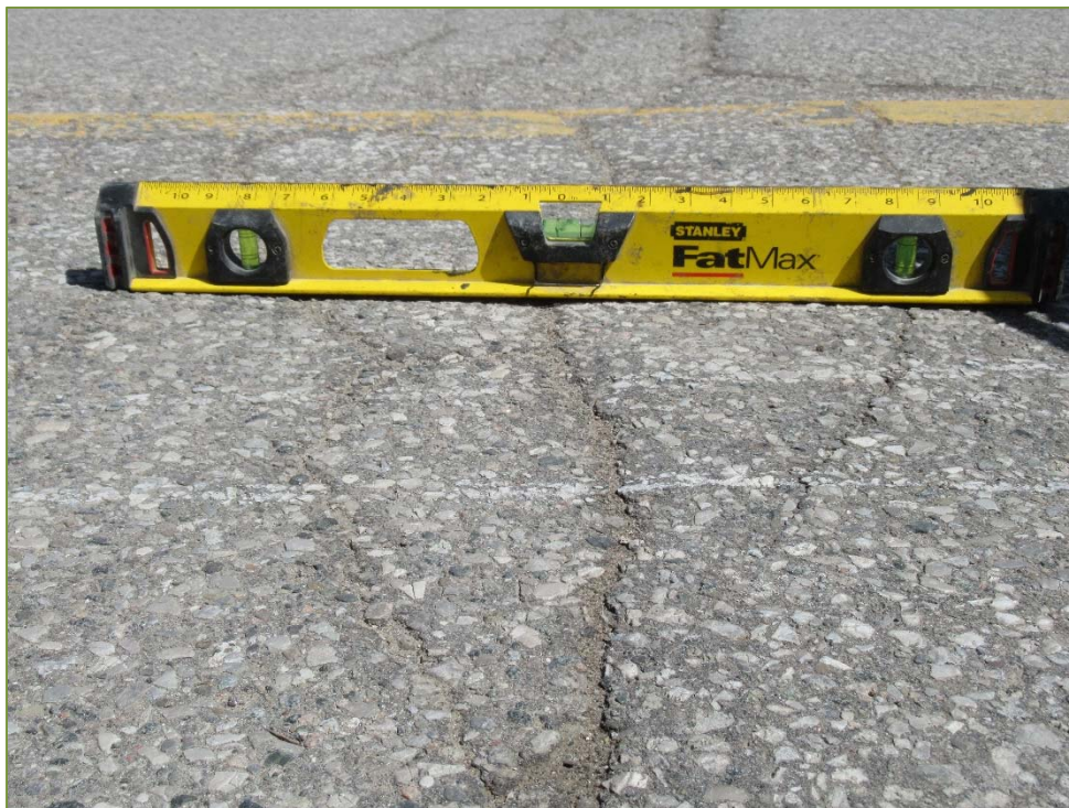
Photo P8 – Deck Wearing Surface (unsealed cracks) note minor settlement
