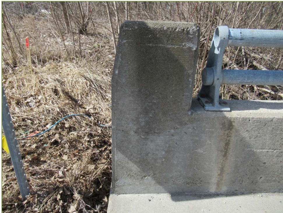
Photo P40 – Southwest End Post note missing handrail end cap
