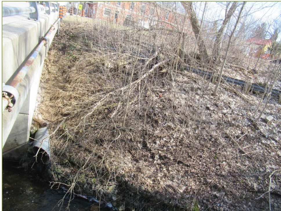
Photo P60 – Southwest Embankment (fair to good condition – soil erosion)
