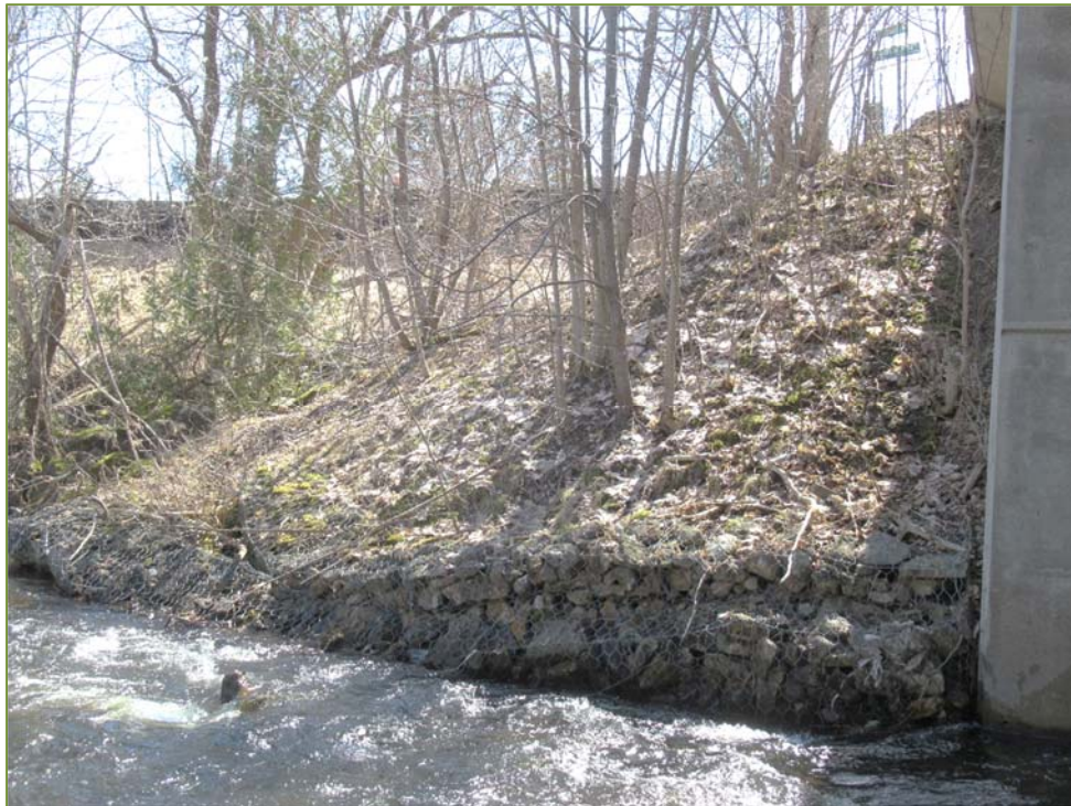
Photo P54 – Southeast Gabion Wall (fair condition – overturning)
