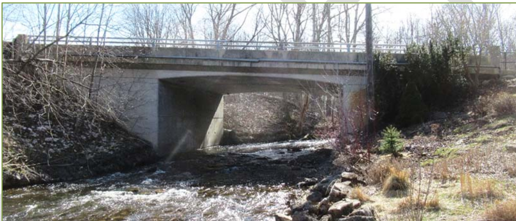
East Elevation of Site B26030042, Main Street, Alton
