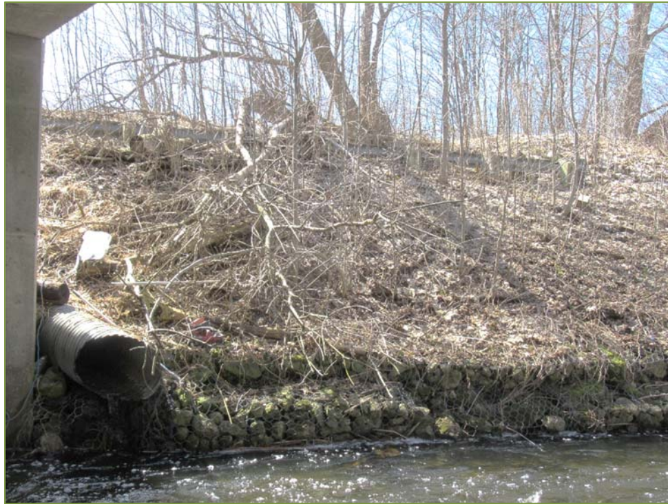
Photo P55 – Southwest Gabion Wall (fair condition – overturning and damaged gabion basket)
