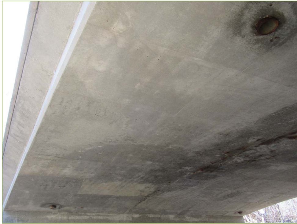
Photo P9 – Soffit (fair condition – cracks, delamination and wet area)
