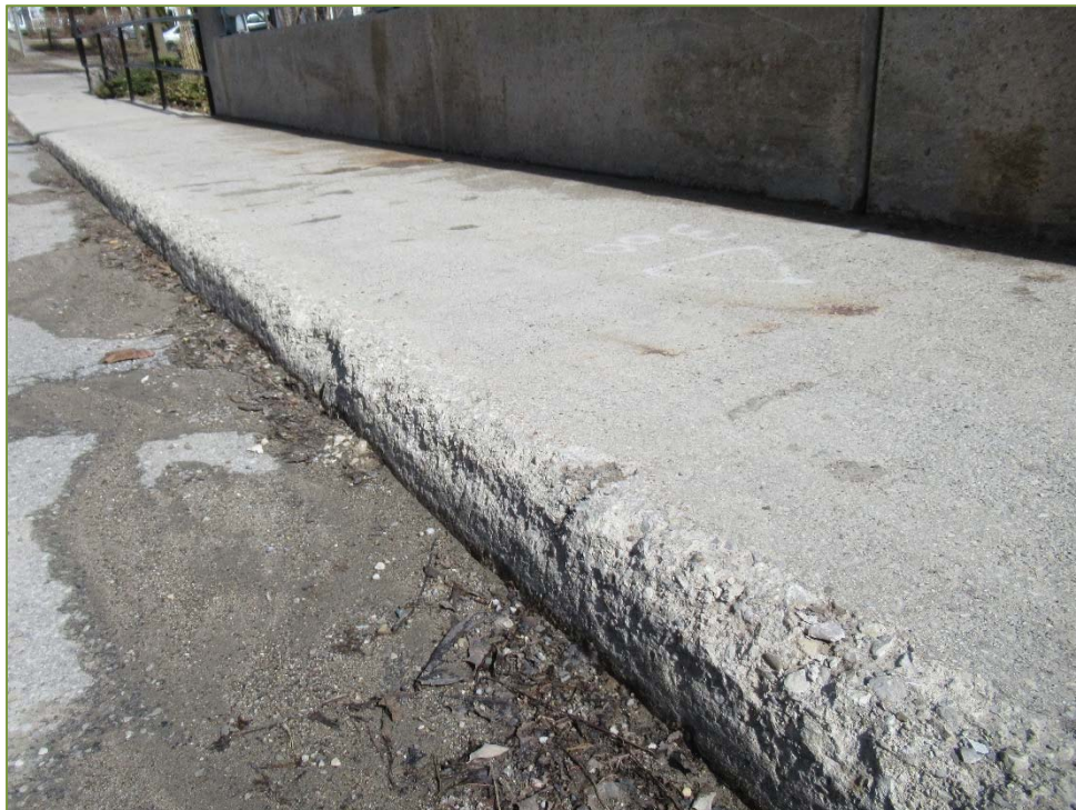
Photo P26 – East Sidewalk (medium scaling)
