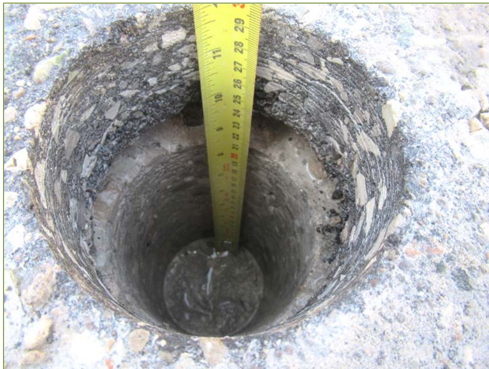
Photo P70 – Typical Condition of Inside Core – C12 (disintegration)
