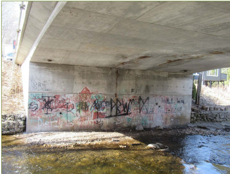
Photo P42 – North Abutment (fair to good condition – wide crack and wet area)
