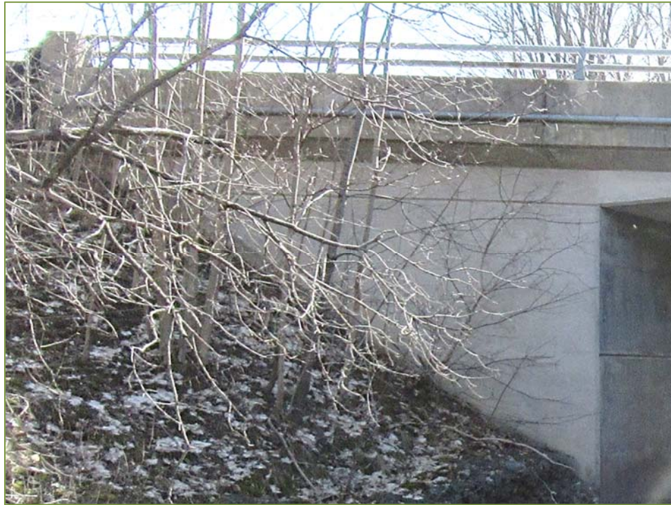
Photo P49 – Southeast Wingwall (good condition)
