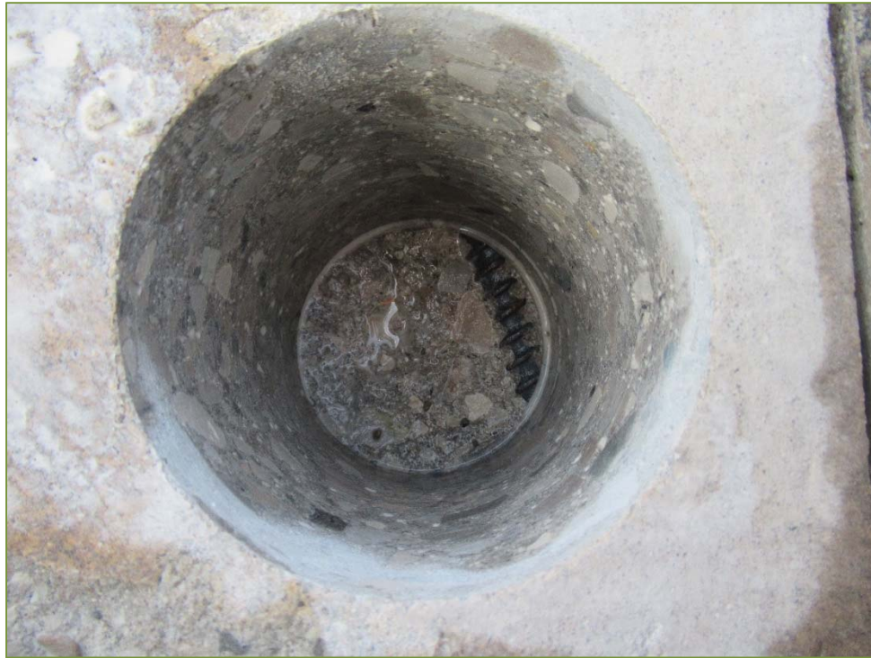
Photo P69 – Typical Condition of Inside Core – C11 (inside SS8)
