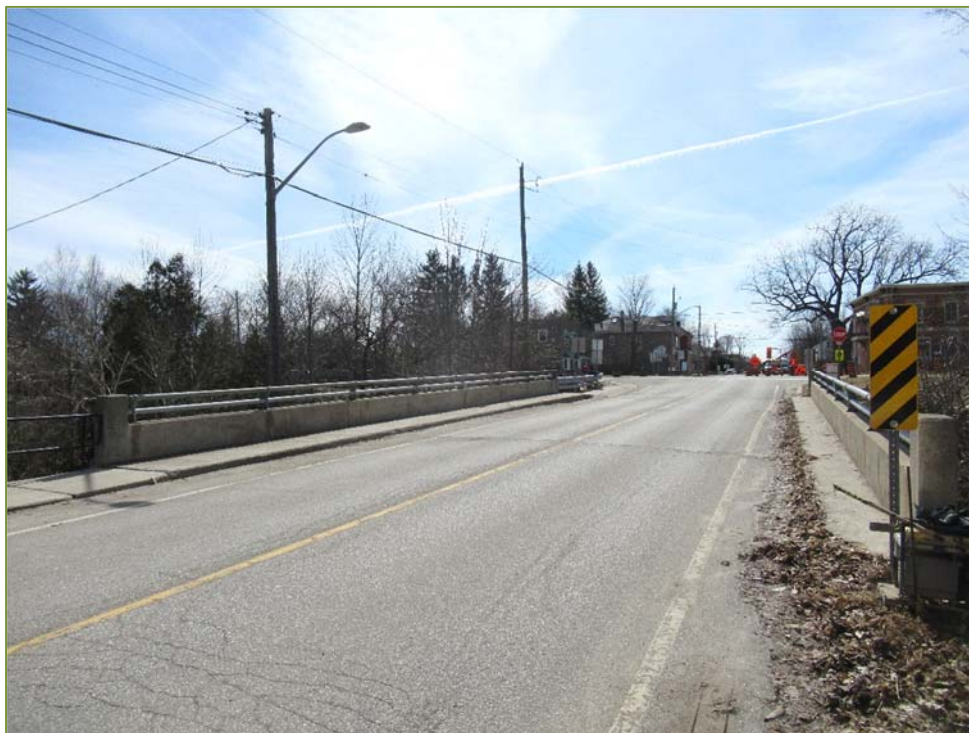
Photo P4 – Deck General View, looking south
