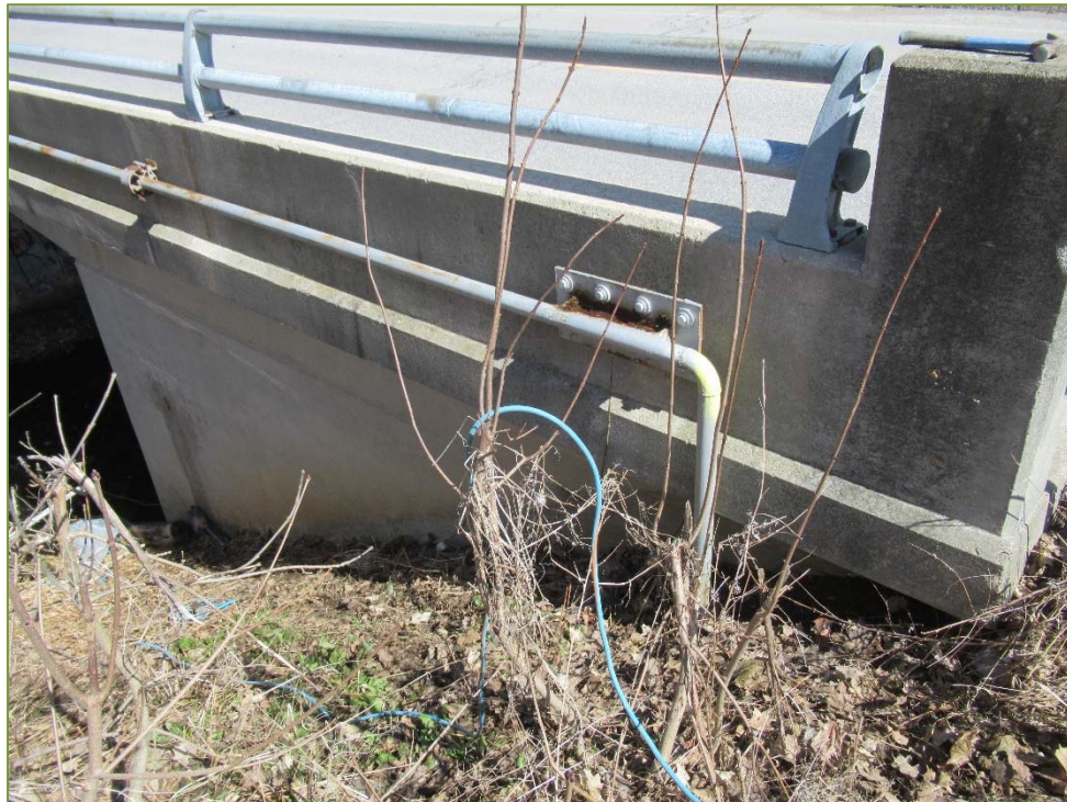
Photo P50 – Southwest Wingwall (good condition)
