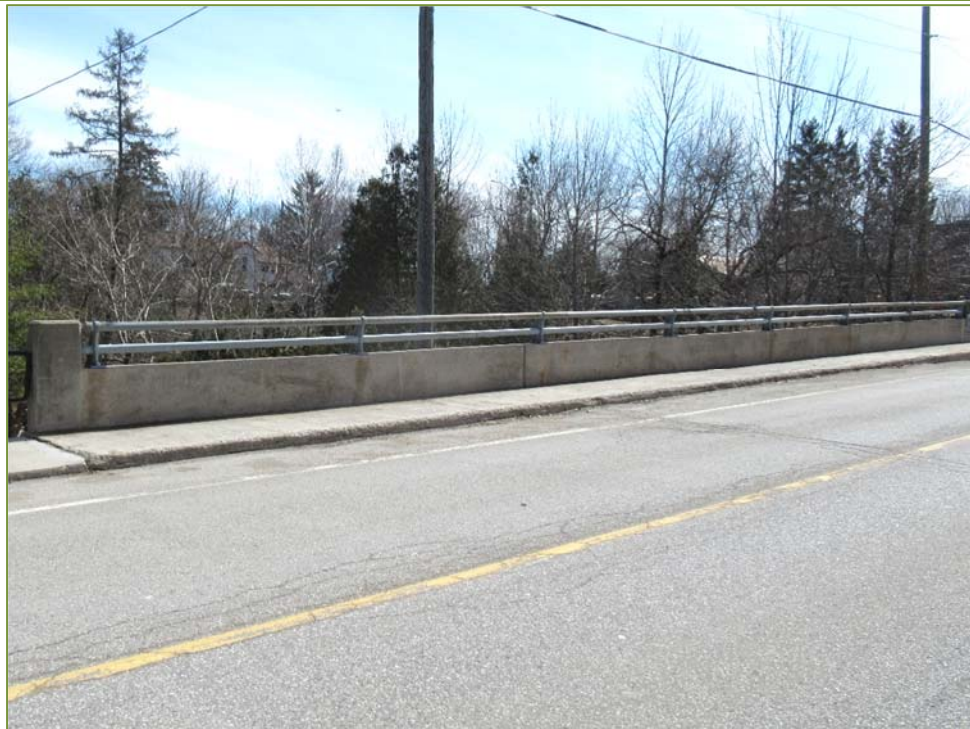
Photo P24 – East Sidewalk (fair condition – wide crack, spall, delamination and light/medium scaling) and Parapet Wall (fair to good condition – cracks, delamination and light scaling)
