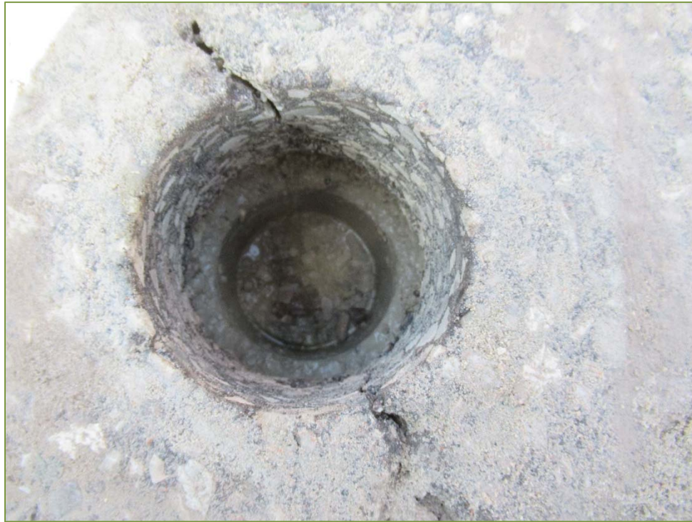
Photo P67 – Typical Condition of Inside Core – C9 (disintegration)
