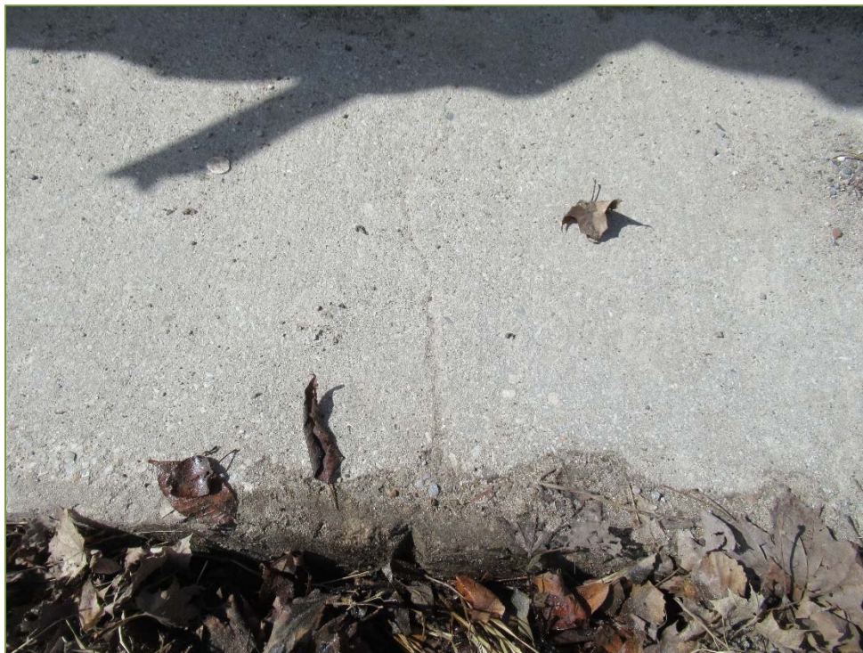
Photo P34 – West Curb (crack and medium scaling)
