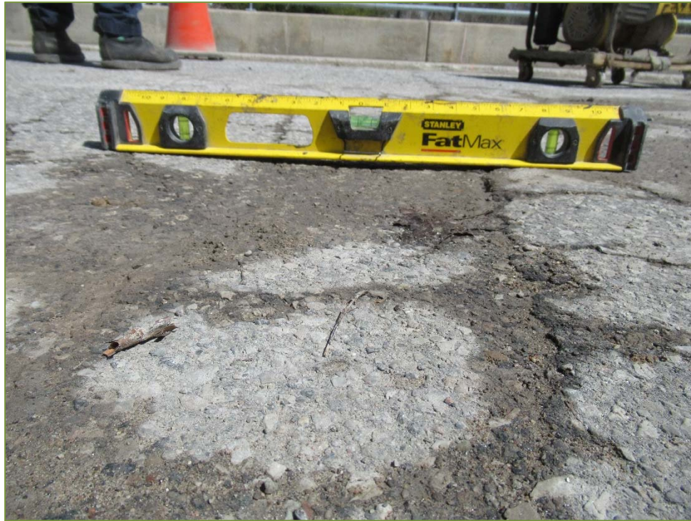
Photo P15 – North Approach Wearing Surface (unsealed cracks) note settlement
