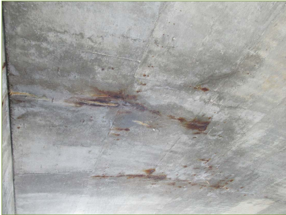
Photo P11 – Soffit at North Abutment (cracks, delamination and wet area)
