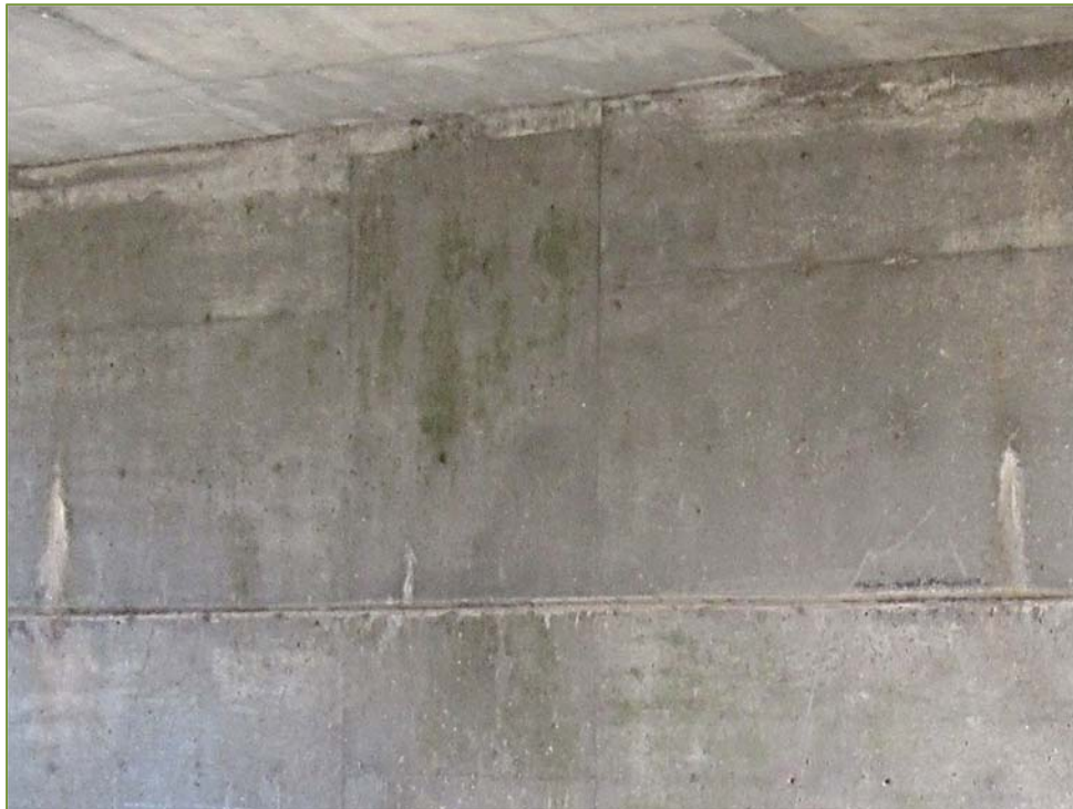
Photo P46 – South Abutment (cracks)
