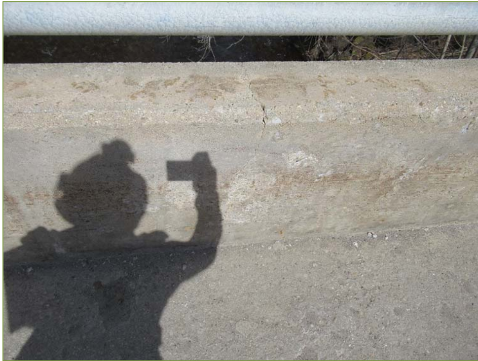
Photo P25 – East Parapet Wall (crack and light scaling)
