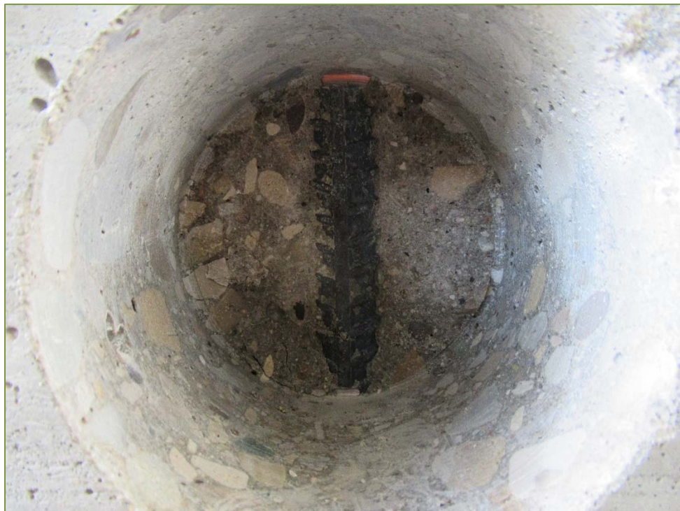
Photo P72 – Typical Condition of Inside Core – C15 (south abutment)
