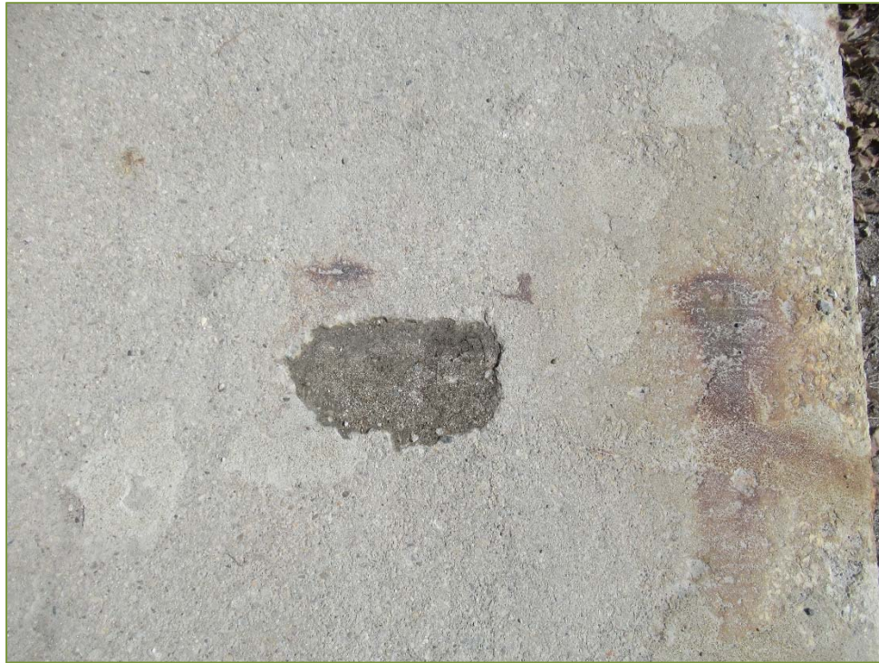
Photo P29 – East Sidewalk @ South Approach (spall and light scaling)
