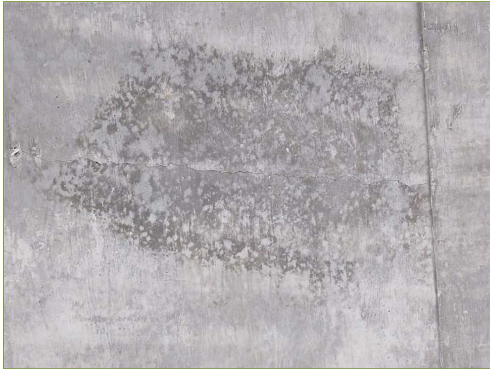
Photo P13 – Soffit (crack and wet area)
