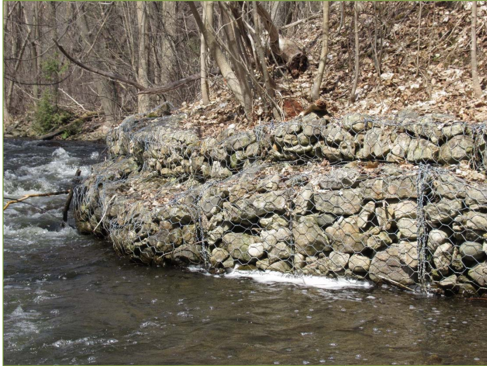
Photo P53 – Northwest Gabion Wall (bulging)
