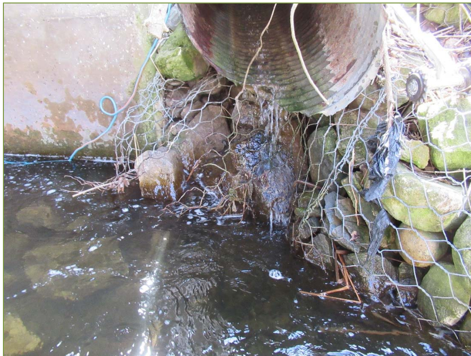
Photo P56 – Southwest Gabion Wall (overturning and damaged gabion basket)
