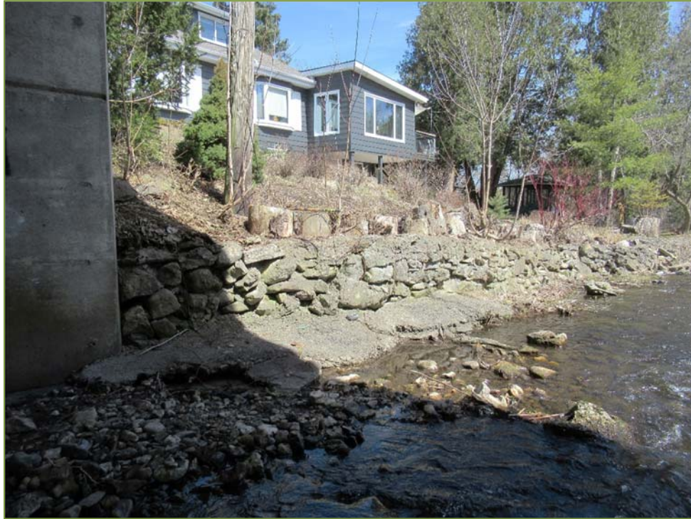
Photo P51 – Northeast Gabion Wall (good condition)
