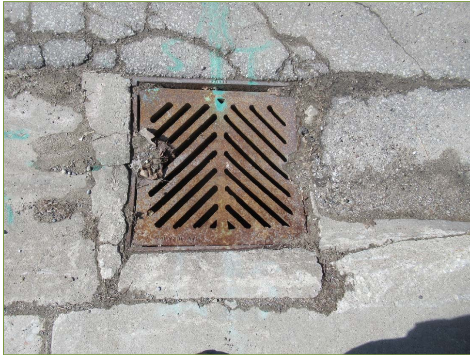
Photo P23 – Southeast Catch Basin
