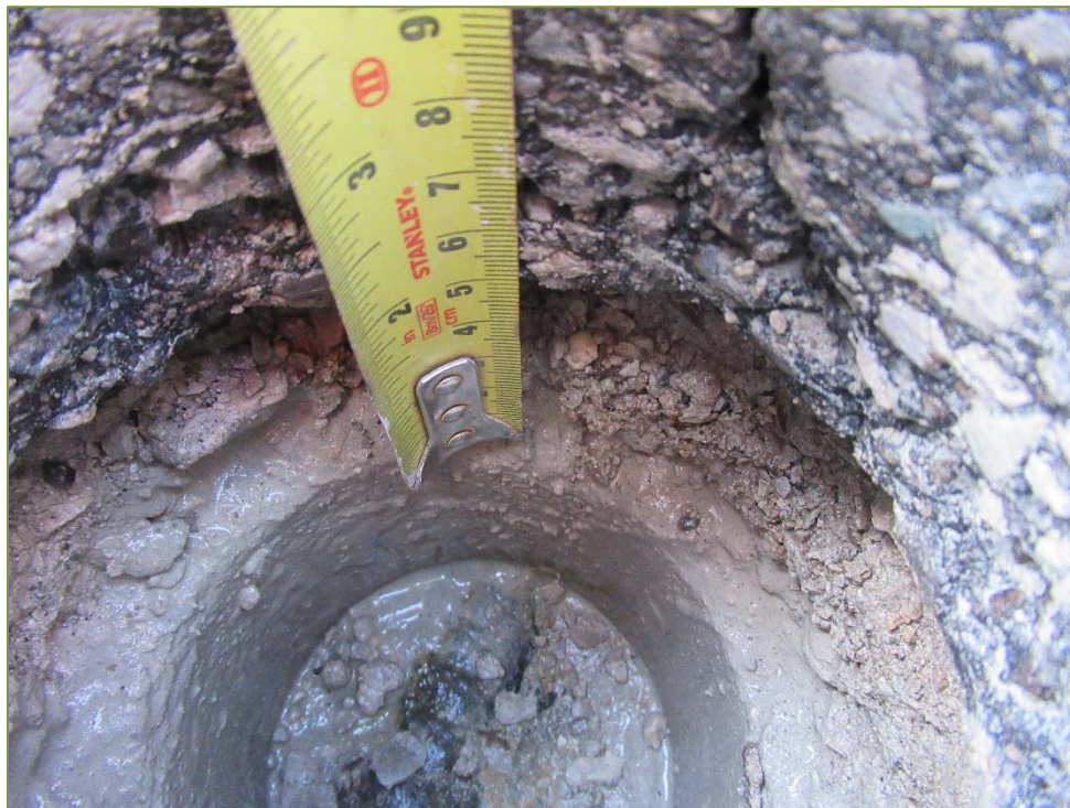
Photo P68 – Typical Condition of Inside Core – C9 (disintegration)
