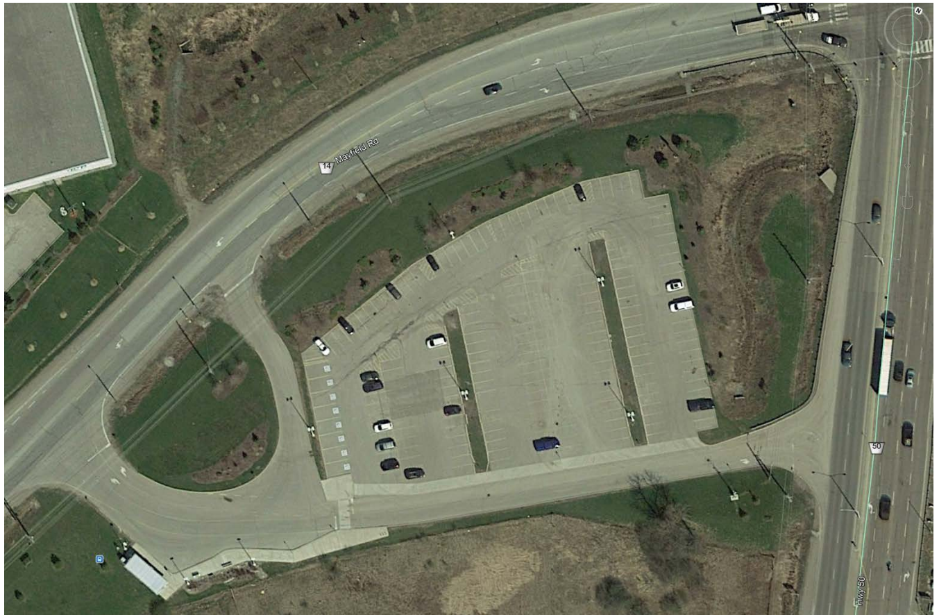
GO TRANSIT'S PARK & RIDE BUS STATION – SW CORNER OF QUEEN STREET (HIGHWAY 50) & MAYFIELD ROAD
