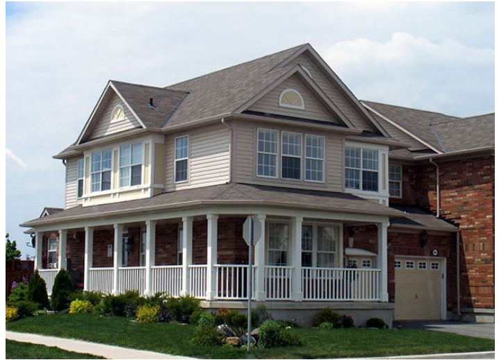
Corner lot with front entrance on flanking street, increased fenestration and a dominant porch.
