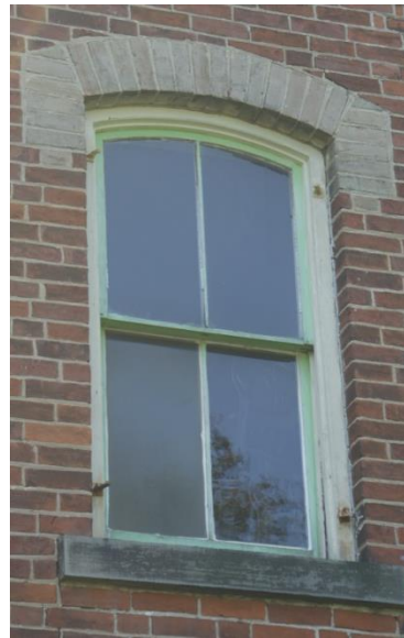
Figure 18 – Window & Arched Brick Header
