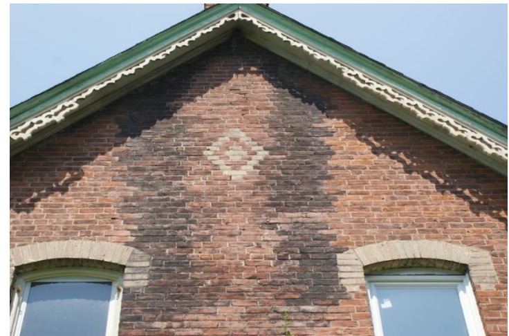
Figure 10 – Damage to Brick
