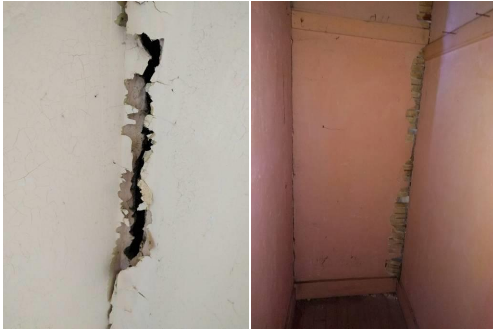
Plate 23a - 23b: Detail of signs of settling, front of house, lathe and plaster separation.
