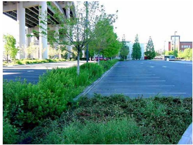
Figure 7.2a – Image example of integrating bio-retention swales for managing stormwater within expansive areas of runoff.
