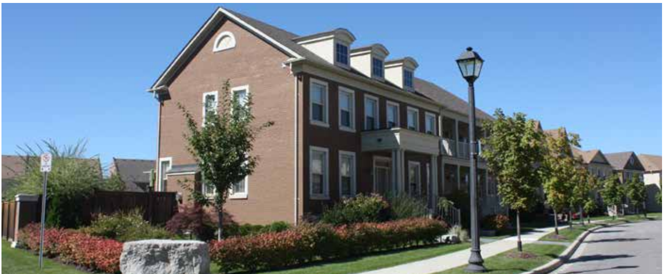
Figure 8.5.8f – Dwellings with rear-accessed garages contribute to the streetscape appearance.
