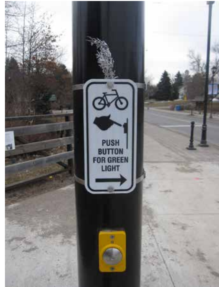
Figure 5.4j – Signage related to pedestrian / cyclist activated signal crossing ahead.
