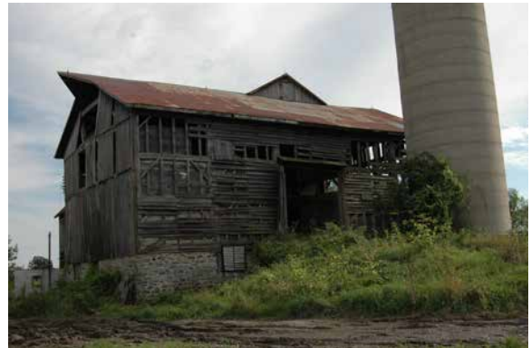
Figure 5.9a – Photograph showing the existing gable roofed barn structure.
