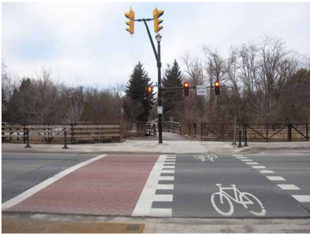
Figure 5.4n – Image example of a recently installed signalized mid-block trail crossing of an arterial road within Caledon, including pedestrian and cycling signals, transition space and decorative crosswalk paving.
