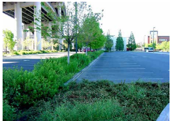
Figure 4.5g – Example of bio-retention swales used to manage expansive areas of runoff.
