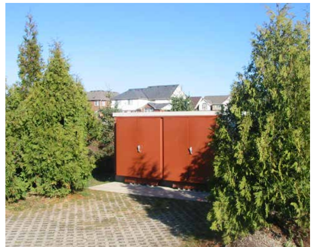
Figure 6.10.4 – Image example of a Bell CUE unit partially screened within an easement adjacent to a SWM pond facility.
