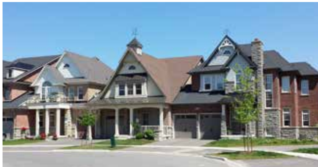
Figure 8.5.11f – Image example of street elbow dwellings terminating views with upgraded architectural treatment.
