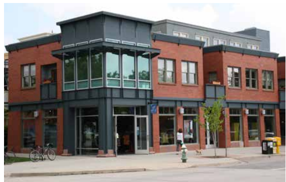
Figure 4.4.2b: – Example of commercial built form that displays a 'village character' with strong orientation to the street and access from the sidewalk.
