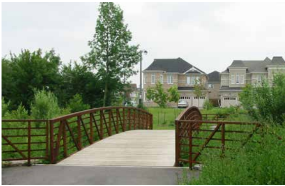
Figure 5.4k – Image example showing a prefabricated steel pedestrian bridge crossing within the NHS.
