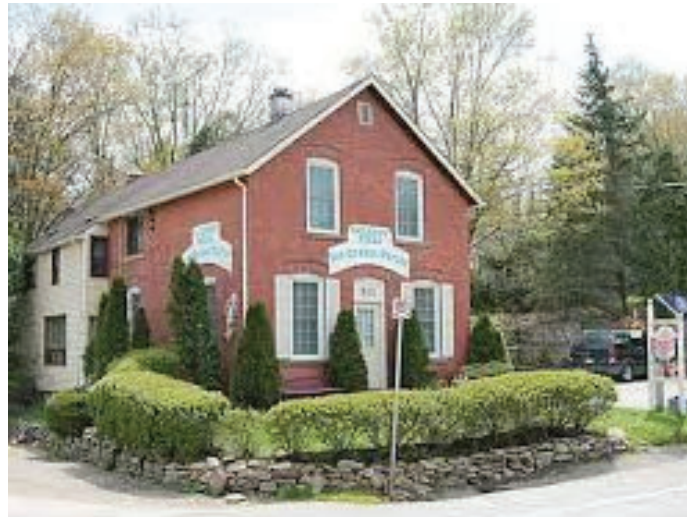
Figure 20: Building in Belfountain
