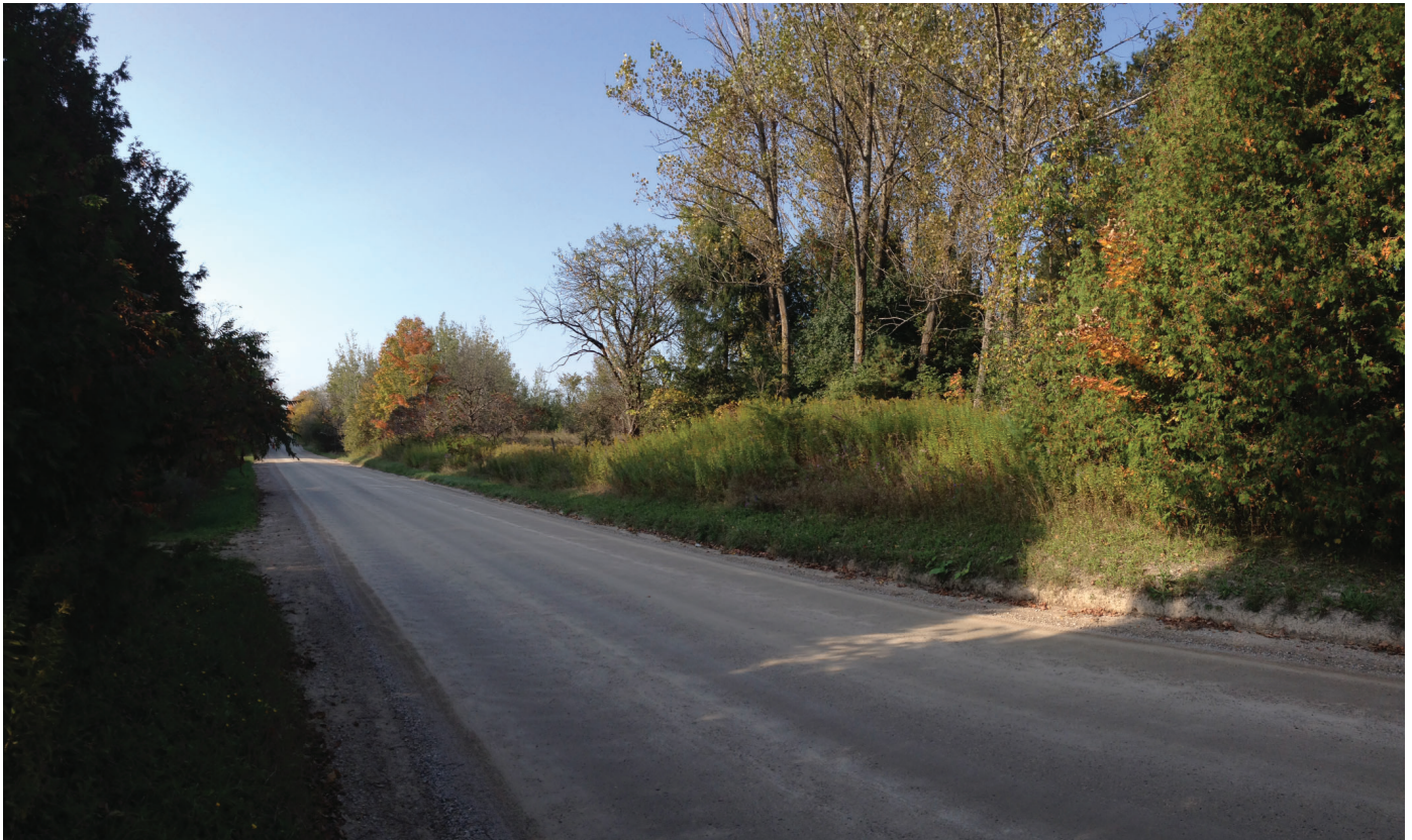
Figure 5: Photo of existing condition
