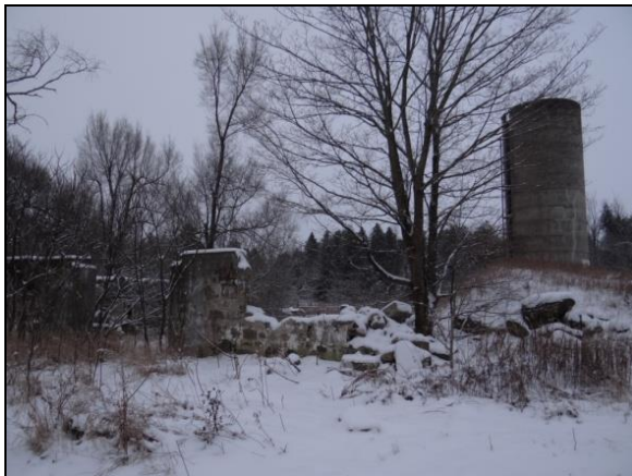
Plate 15: Remnant farmscape (CHL 2) structures, looking southwest from Mississauga Road (December 2017).
