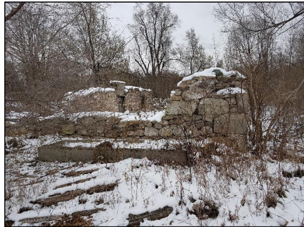
Figure 21: Barn structure ruins within the remnant farmscape, looking north
