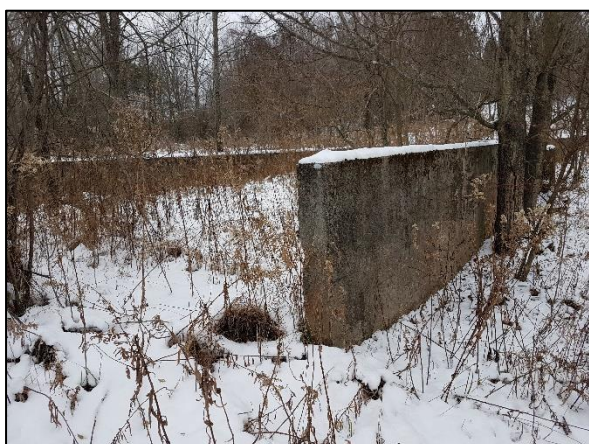
Figure 18: Concrete foundation within remnant farmscape to the south of the barn structure, looking southeast
