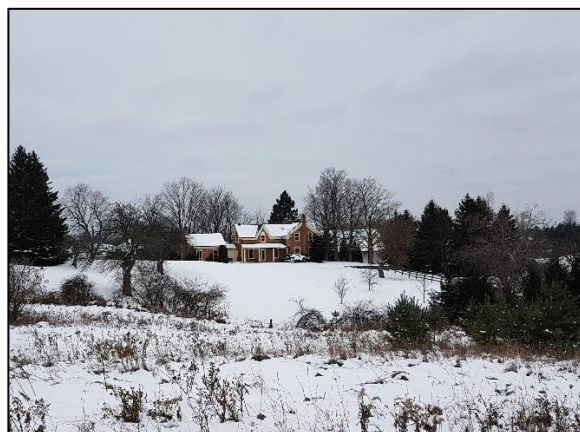
Figure 24: CHL 4 - Farm Complex, 17200 Mississauga Road (ASI 2017)
