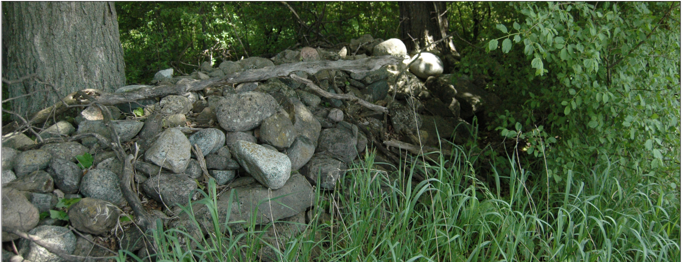
Figure 20: Photo of Existing Stone Wall 3
