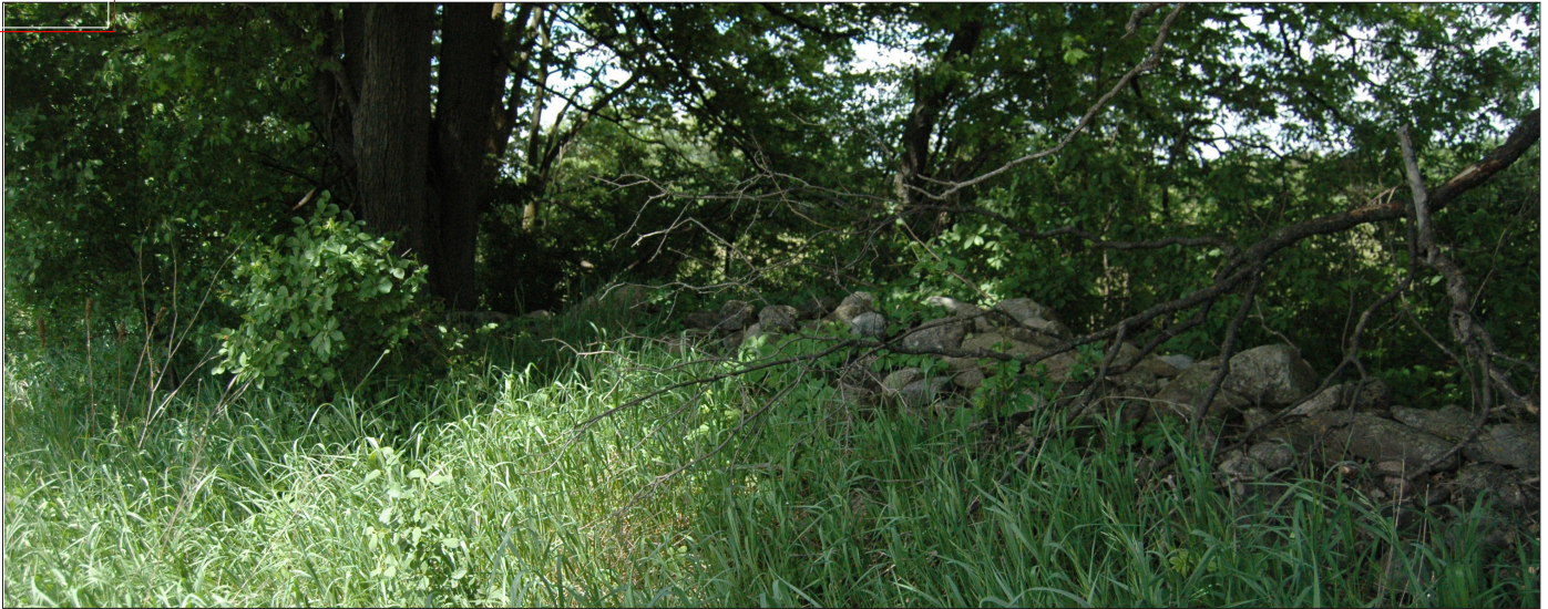
Figure 18: Photo of Existing Stone Wall 1
