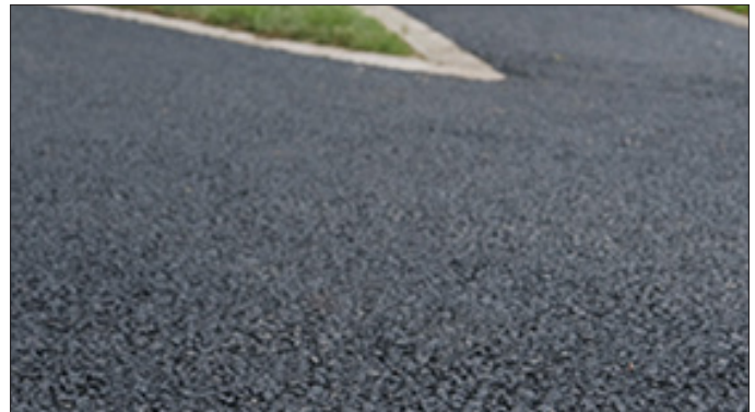
Figure 37: Tar and Chip Driveway
