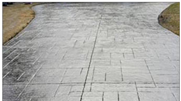
Figure 38: Patterned/Textured Concrete Driveway
