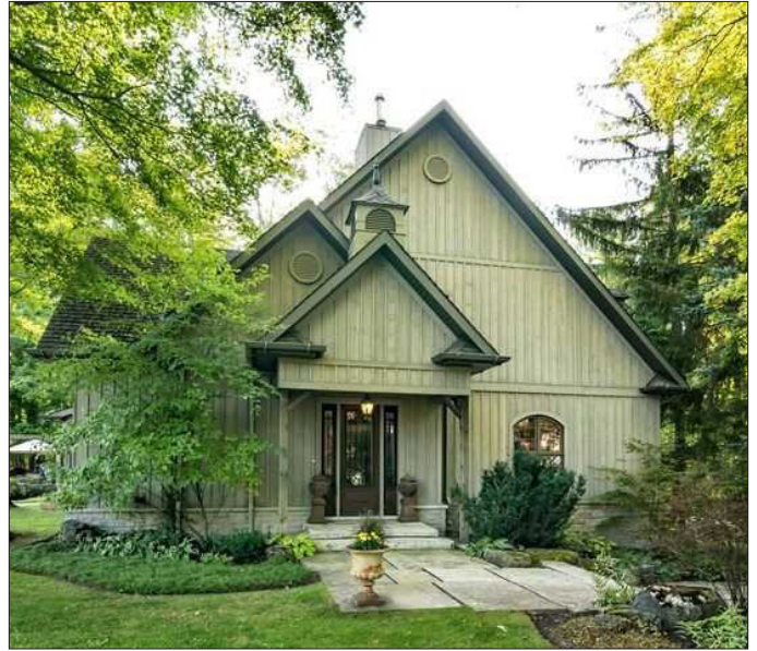
Figure 63: 35 Caledon Mountain Drive: Entry Threshold
