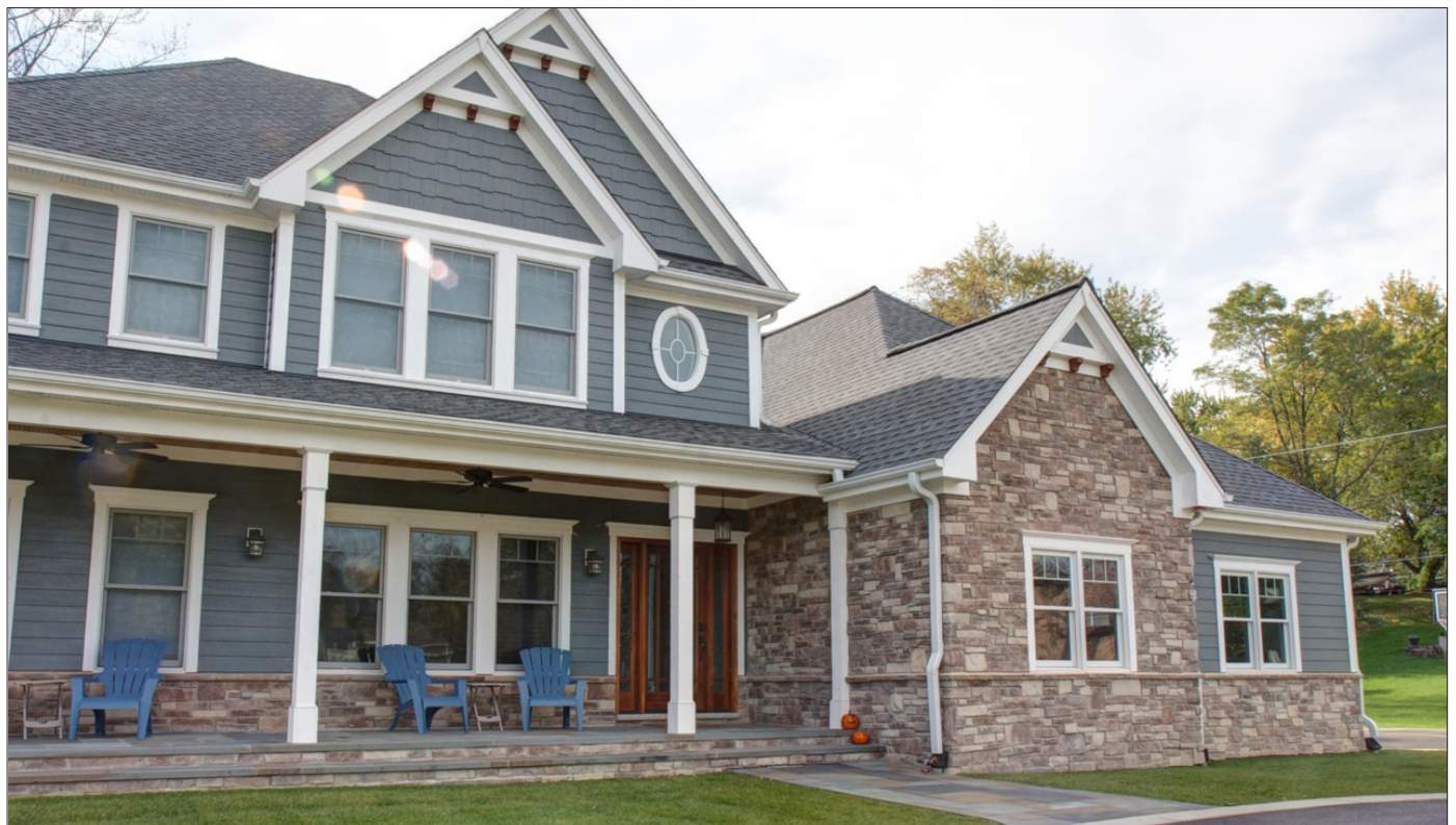
Figure 79: Example of a Combination of Fieldstone and Wooden Siding Materials
