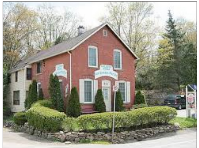
Figure 28: Building in Belfountain
