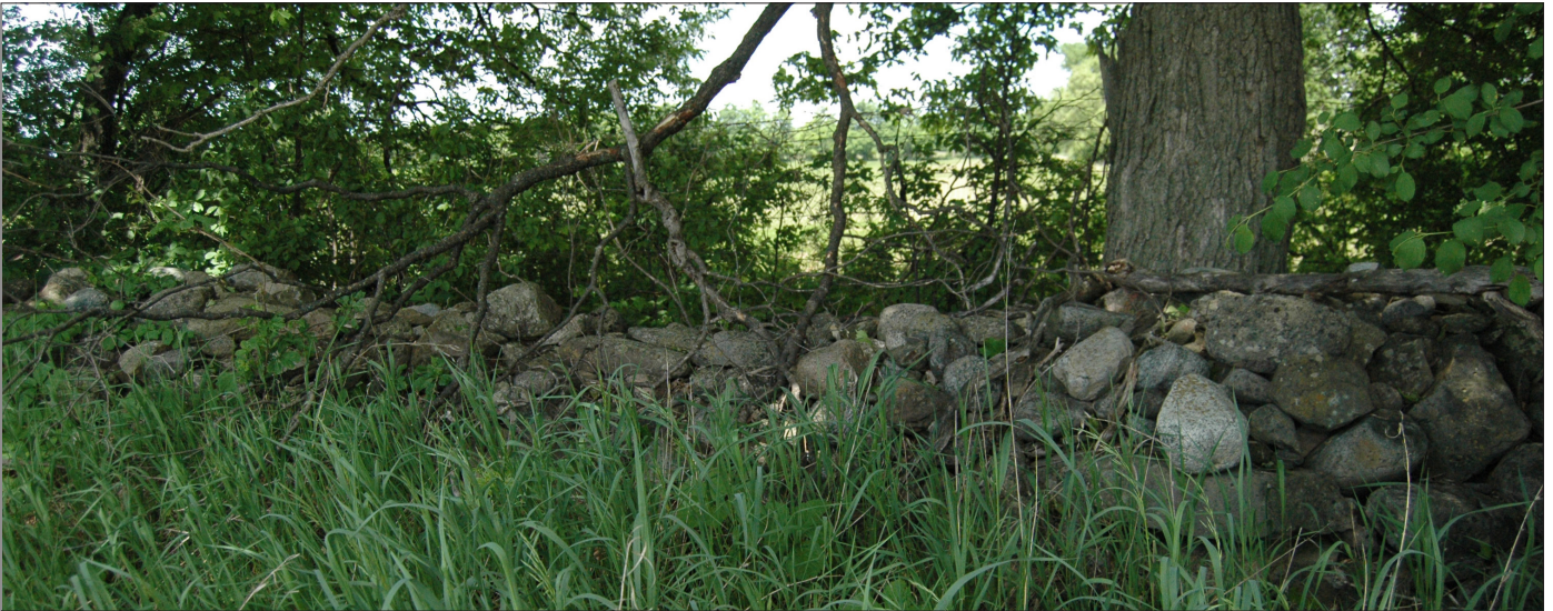
Figure 19: Photo of Existing Stone Wall 2
