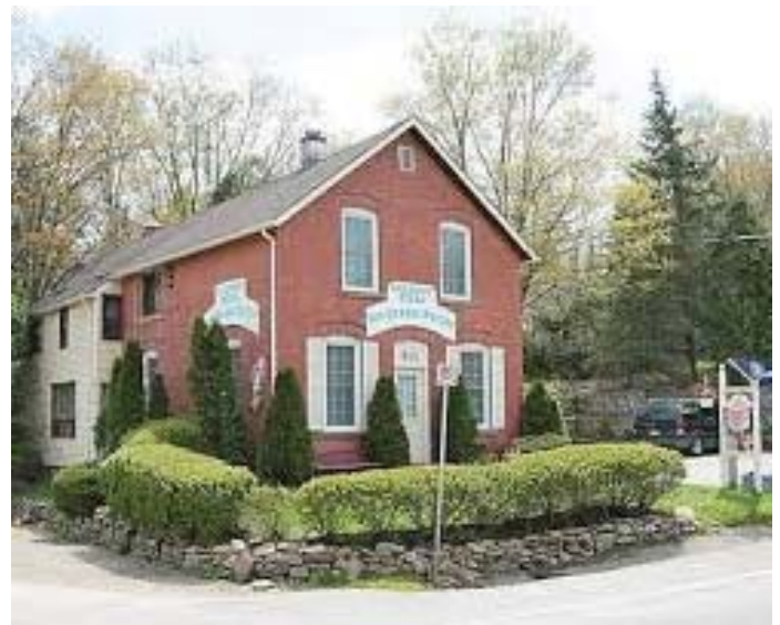
Figure 19: Building in Belfountain
