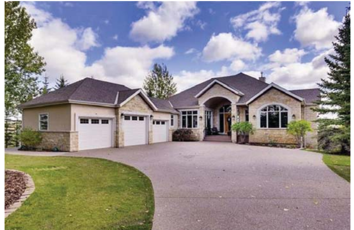
Figure 28: Textured Concrete Driveway
