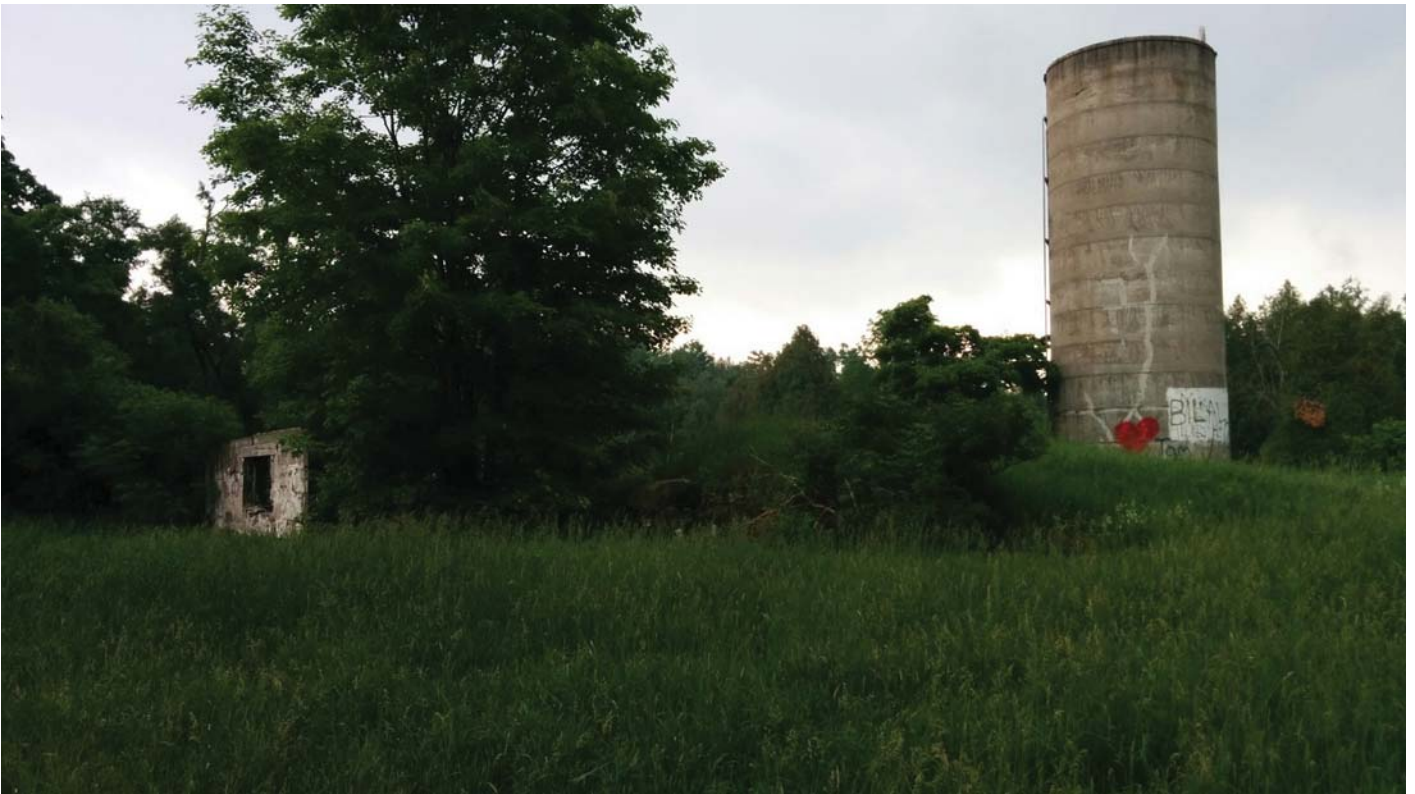
Figure 10: Photo of Existing Condition
