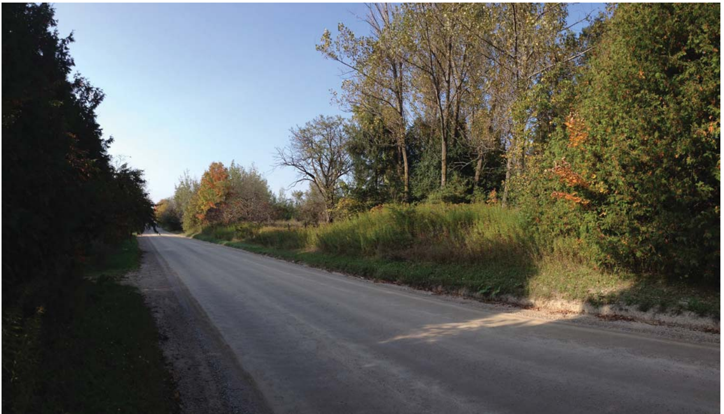
Figure 05: Photo of Existing Condition
