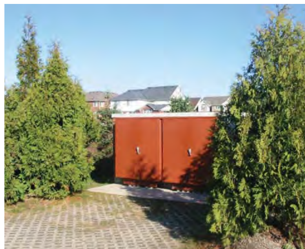
Figure 6.10.5 – Image example of a Bell CUE unit partially screened within an easement adjacent to a SWM pond facility.
