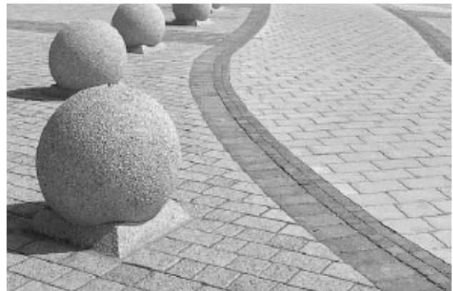
Figure 7.2b – Image example of light-coloured paving which reflects light and serves to reduce the urban heat island effect.
