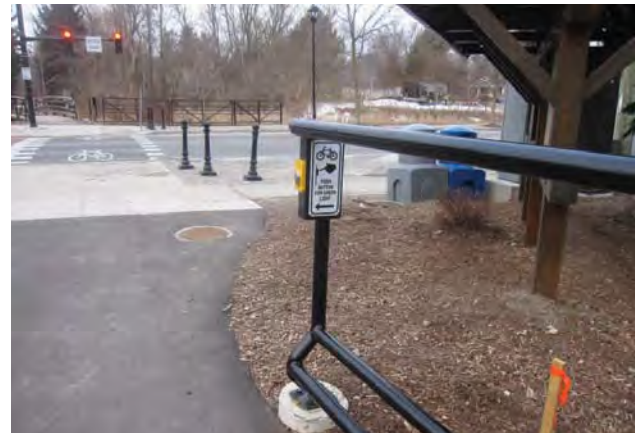
Figure 5.4q – One of the components that provides for a more convenient cycling experience is a signal activated rail.
