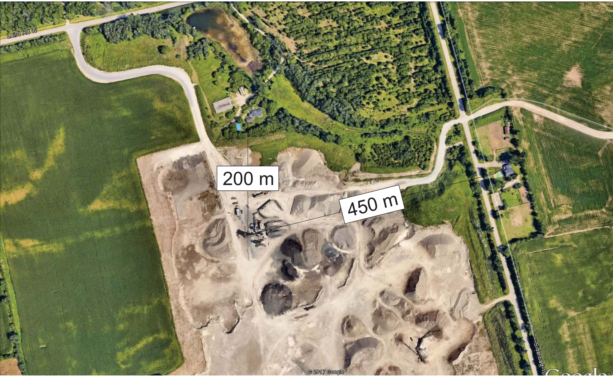
Cox Construction, Guelph Plant
