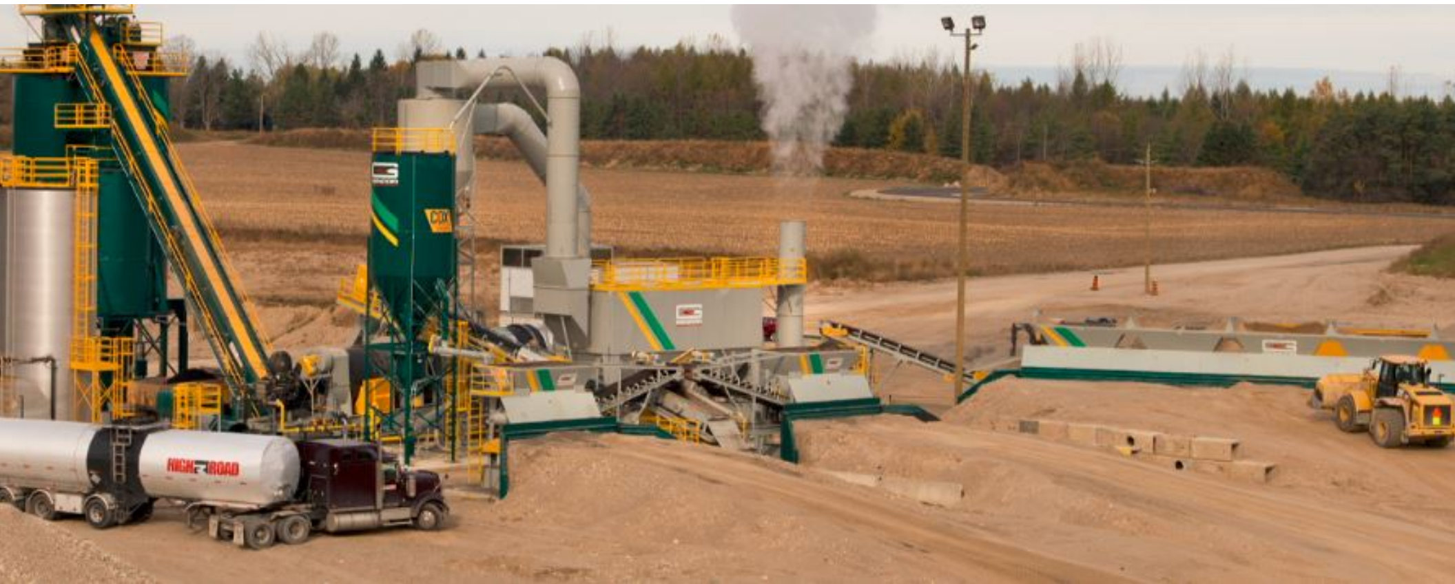
Cox Construction, Guelph Plant
