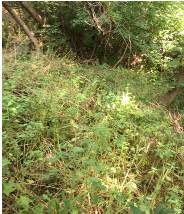
Photo 8: Vegetation on Slope Surface (looking southwest-downslope)
