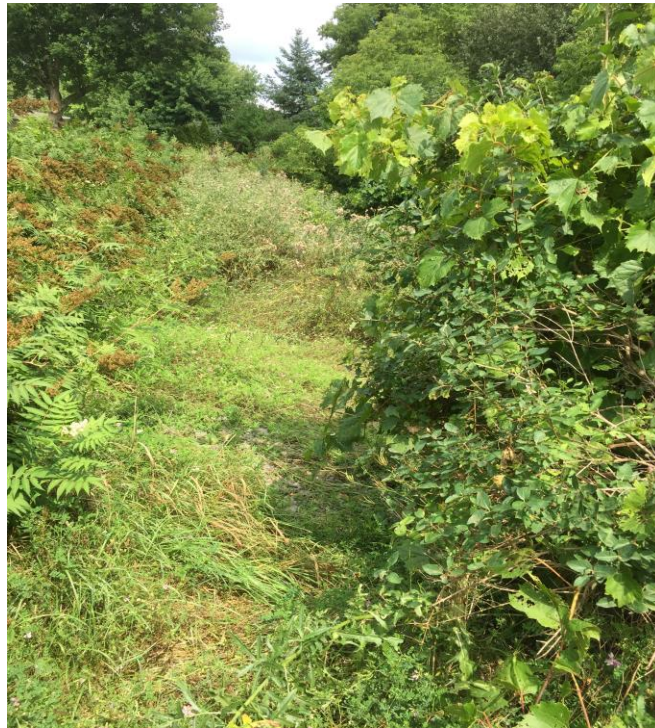
Photo 4: Vegetation on Slope Surface near the top of slope (looking East)
