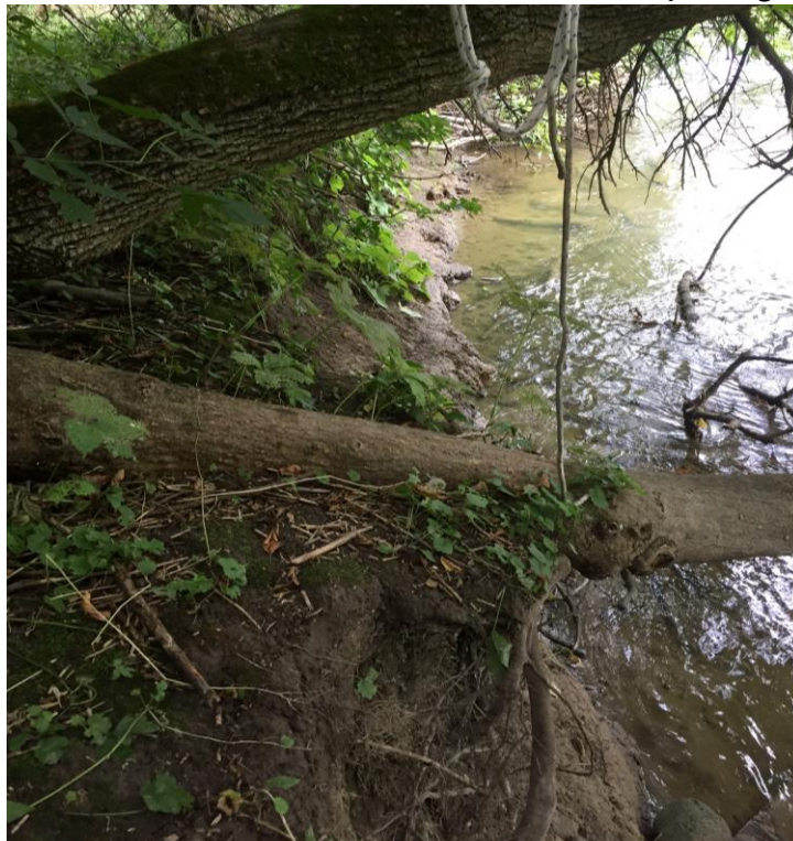
Photo 10: Watercourse Conditions Near Section B-B (looking east)
