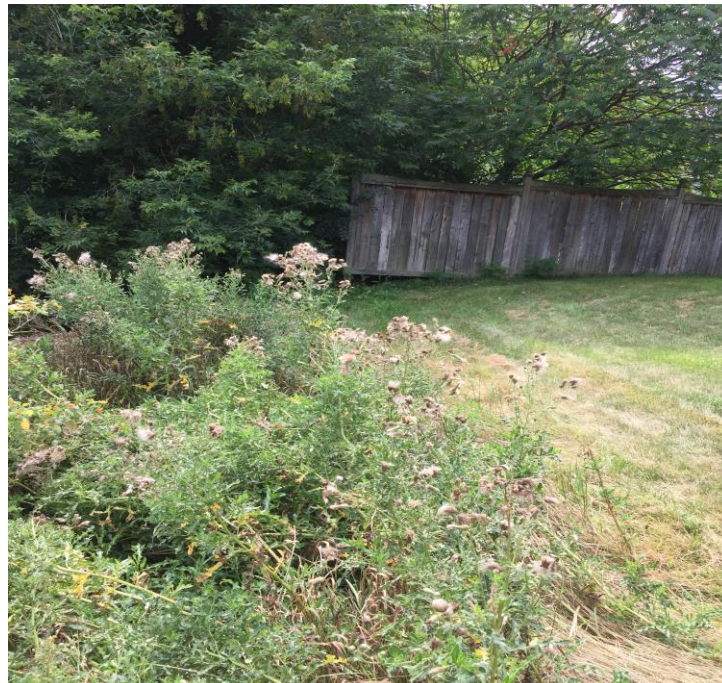
Photo 2: Tableland near Top of Slope Looking west, standing close to BH18-5
