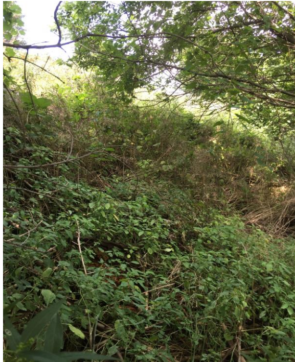
Photo 5: Vegetation on Slope Surface (looking southeast-downslope)
