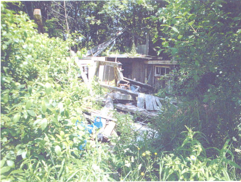
View of the collapsed barn located in the northern section of the subject site (viewing north)
