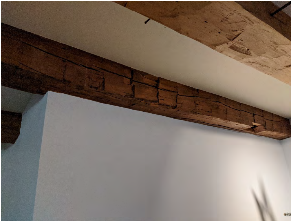
Figure 24: Hand-hewn structural beams (CY 2019).
