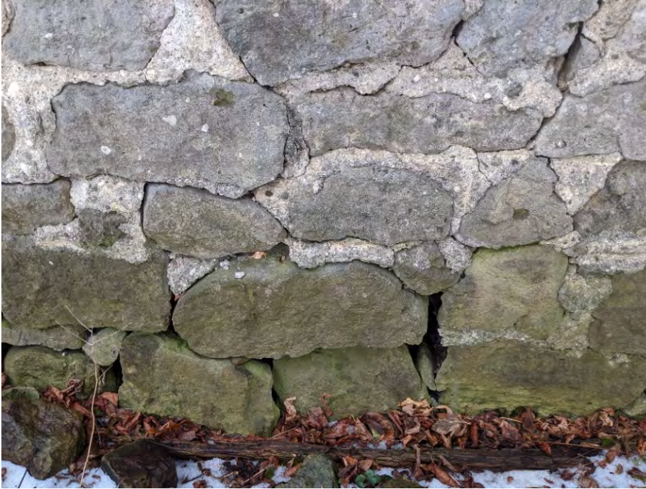
Figure 36: Detail of stone and mortar; materials used for north elevation of attached outbuilding (CY 2019).
