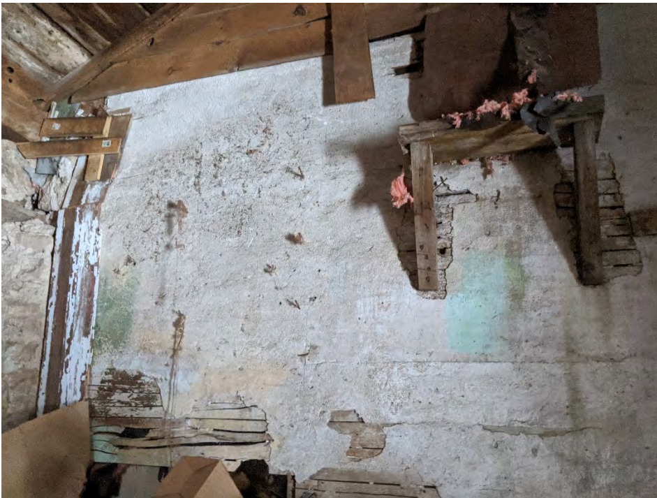
Figure 40: Interior view of attached outbuilding, exposed plaster and lathe – east elevation (CY 2019).
