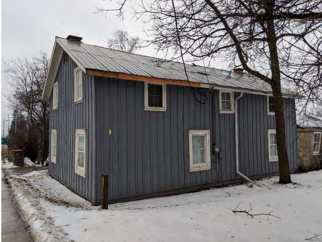
Figure 16: North elevation of structure. Note the two chimneys, wooden soffits, and projecting eaves (CY 2019).
