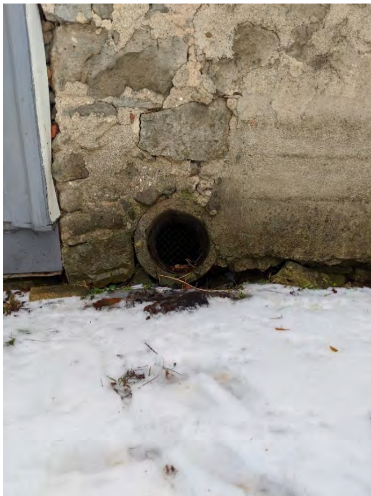
Figure 38: Pipe to attached addition, to which cooling water was delivered to the structure.
