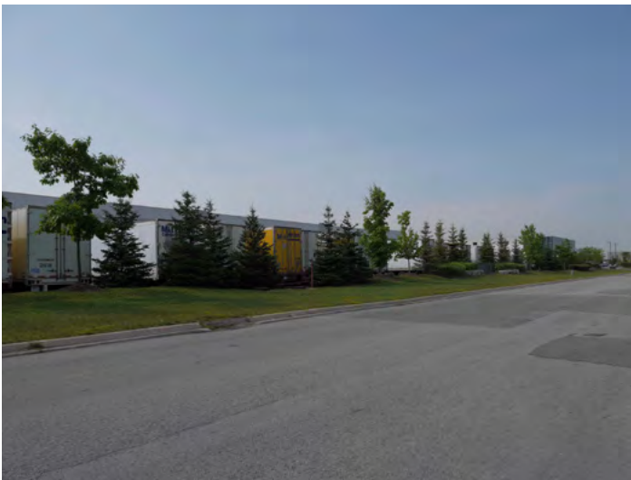
Image 152 - South Bolton Industrial Park, Bolton, ON
