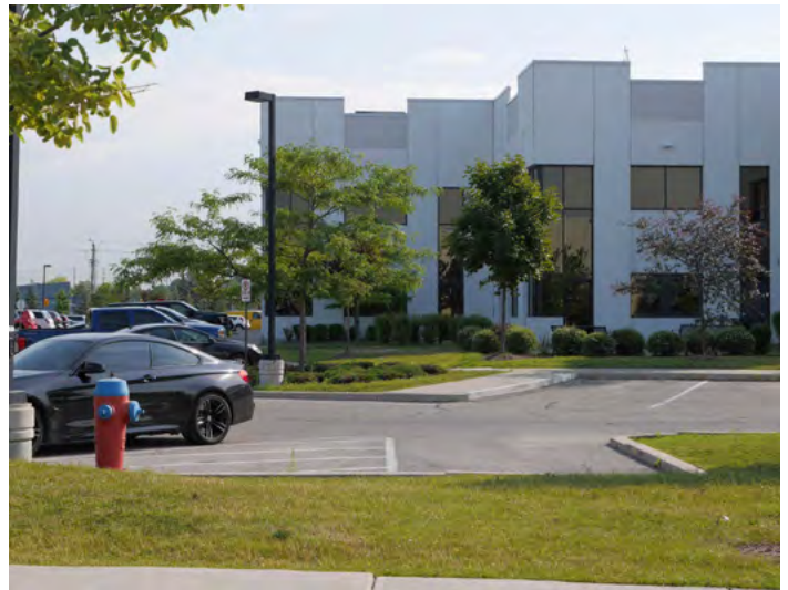
Image 145 - South Bolton Industrial Park, Bolton, ON
