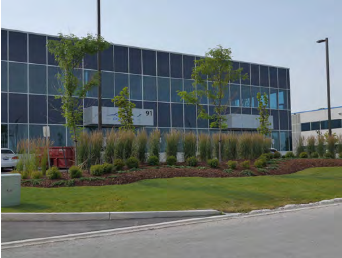
Image 148 - South Bolton Industrial Park, Bolton, ON
