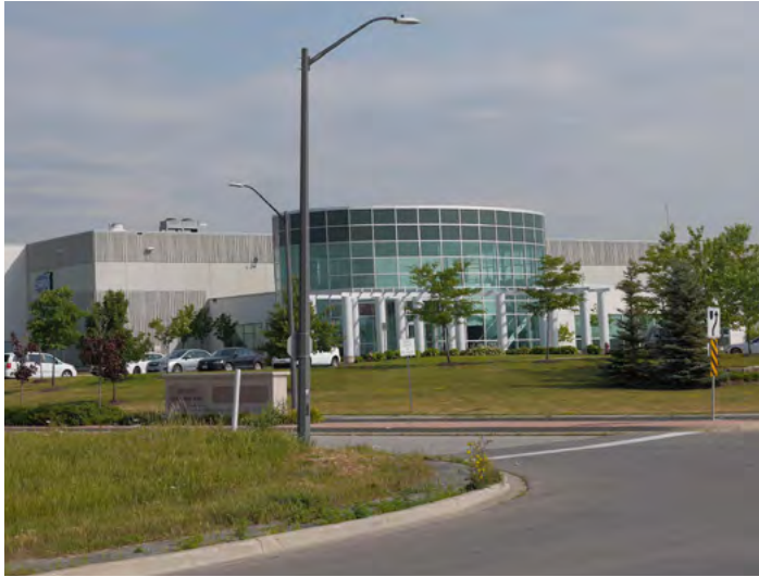
Image 140 - South Bolton Industrial Park, Bolton, ON
