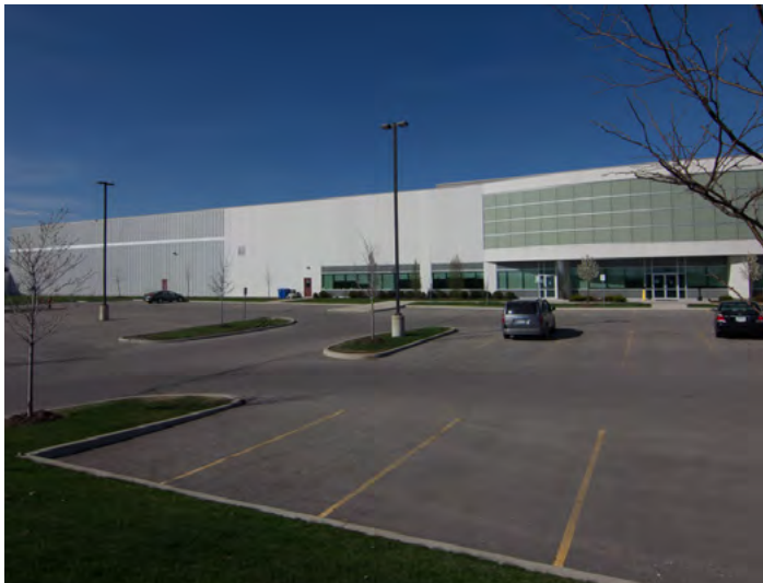
Image 144 - South Bolton Industrial Park, Bolton, ON
