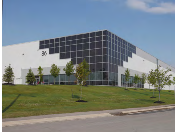
Image 141 - South Bolton Industrial Park, Bolton, ON
