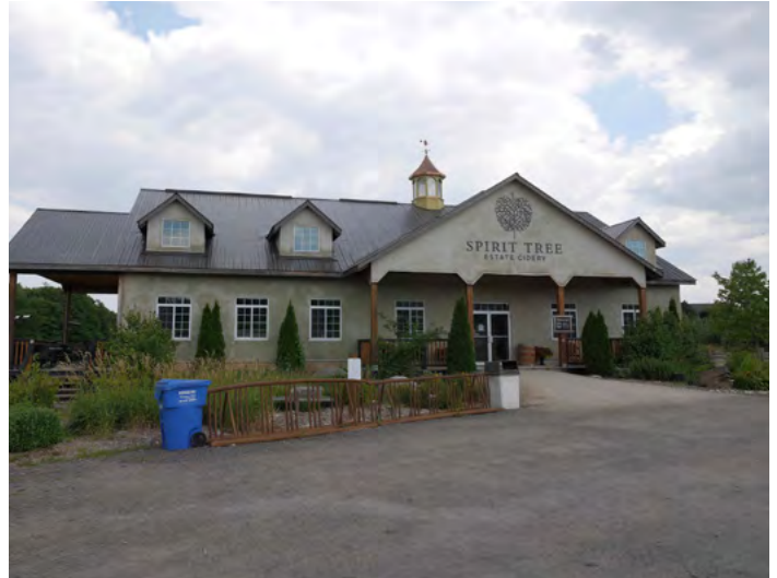
Image 159 - Boston Mills Rd, Caledon, ON
