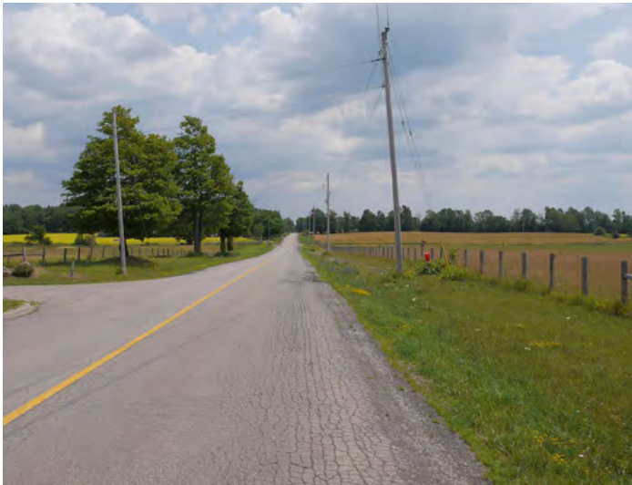
Image 31 - Mississauga Rd, Caledon, ON
