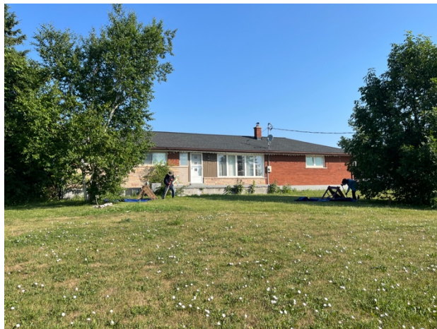
Plate 1: Test Pit Survey Conditions; Existing Structure
