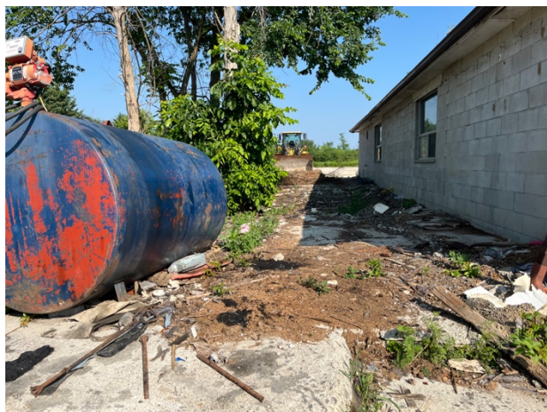
Plate 7: Disturbed Concrete and Gravel Area
