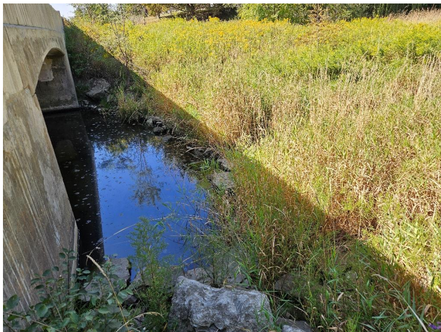
Photo 8. View of pool on the upstream side of the Mayfield Road culvert. Photo taken on September 17, 2025.
