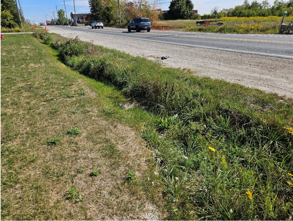
Photo 9. View of ephemeral drainage ditch along the north side of Mayfield Road, facing northeast. Photo taken on September 17, 2025.
