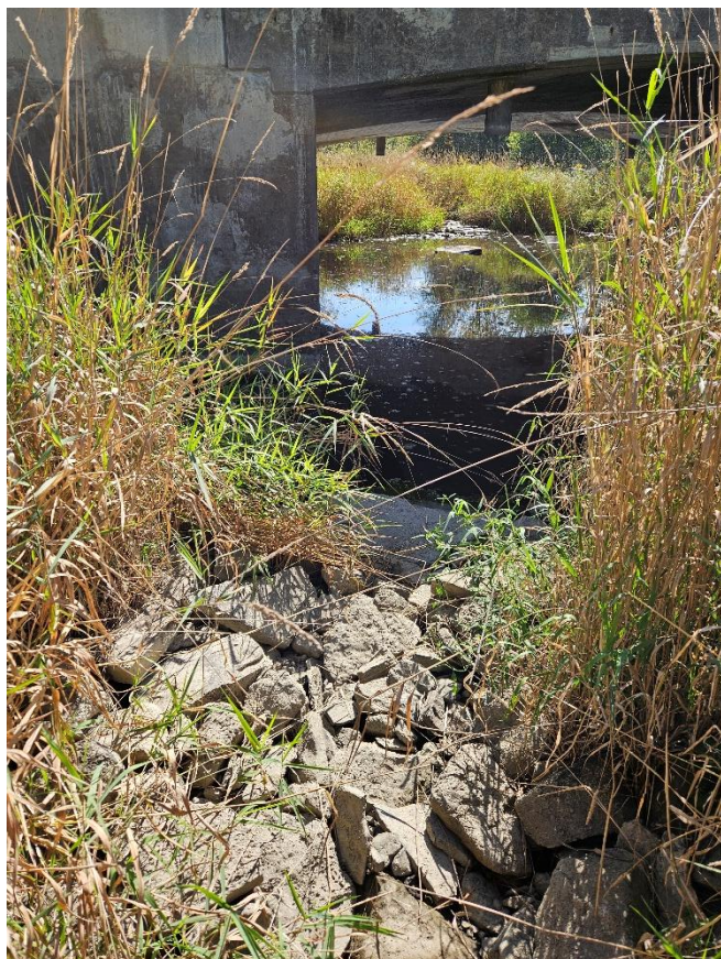
Photo 7. View of Salt Creek channel facing downstream towards Mayfield Road culvert. Photo taken on September 17, 2025.
