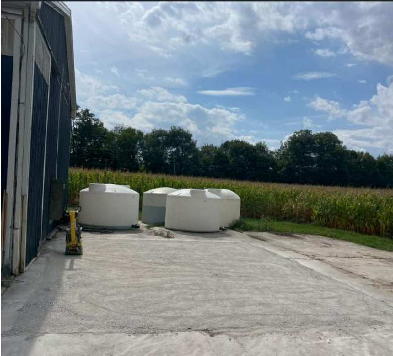
PHOTOGRAPH 6: COMPLETION OF BACKFILLING, (looking northeast)
