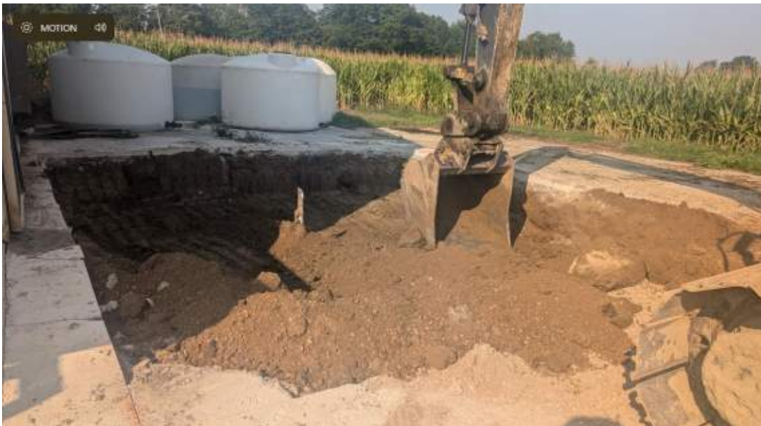
PHOTOGRAPH 2: EXCAVATION IN PROGRESS
