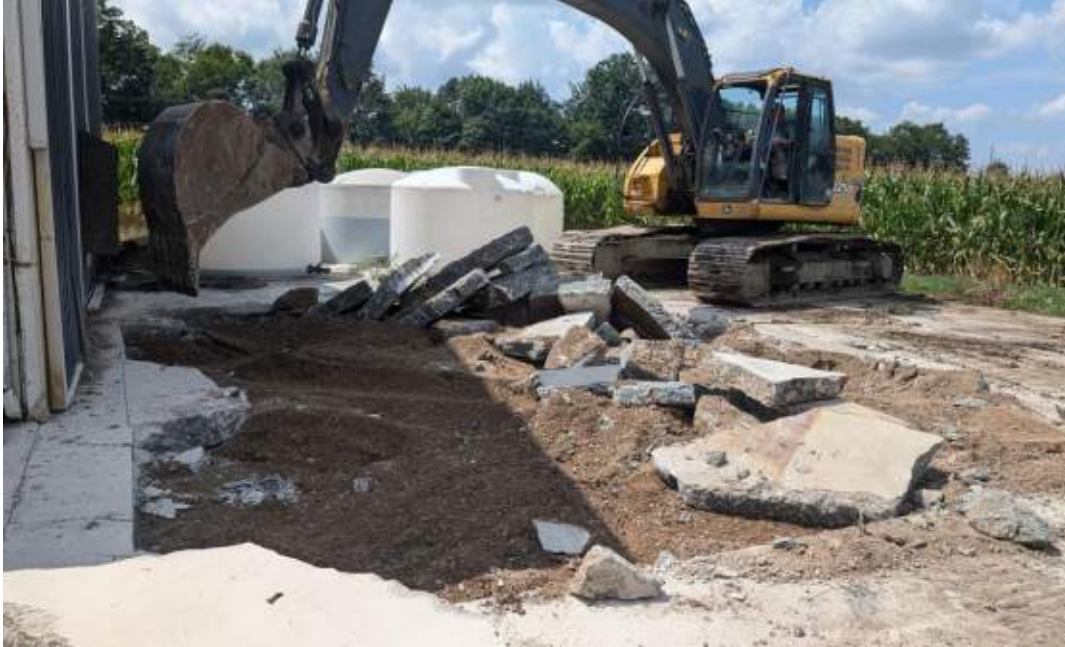
PHOTOGRAPH 1: REMOVAL OF CONCRETE SLAB AT THE SURFACE
