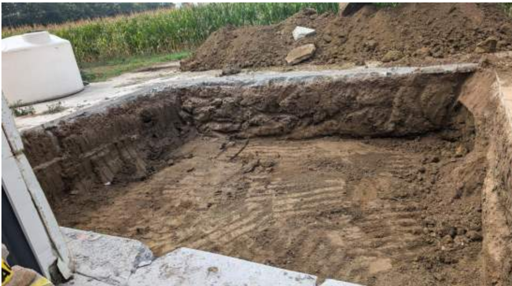
PHOTOGRAPH 4: COMPLETION OF REMEDIAL EXCAVATION, (looking northeast)
