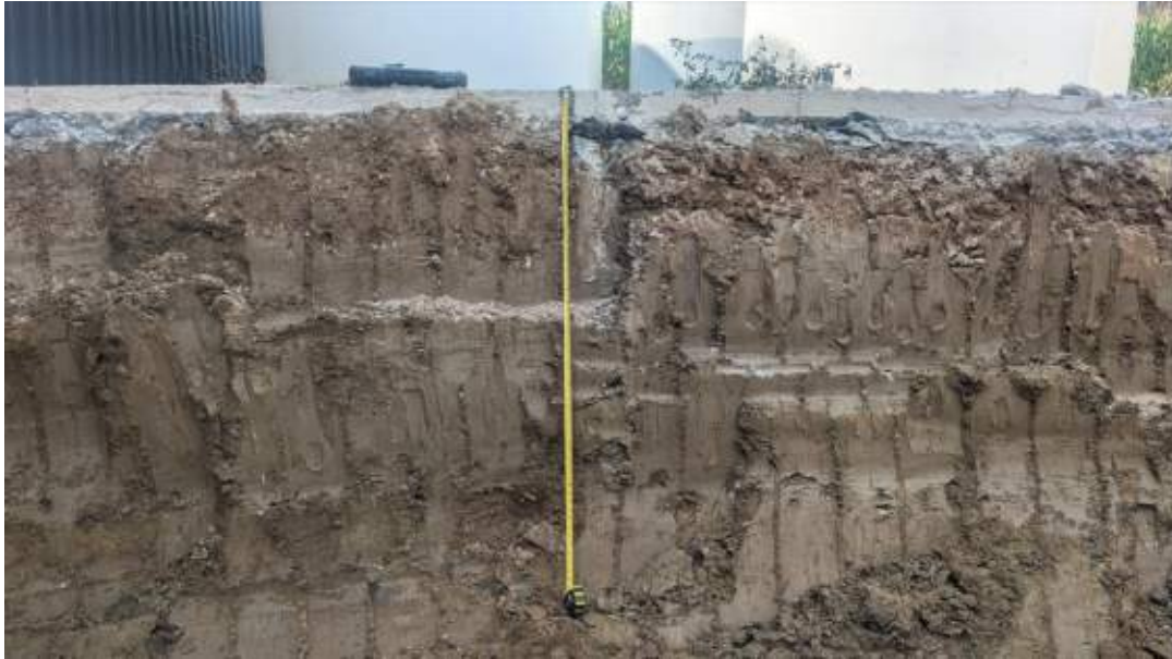
PHOTOGRAPH 3: DEPTH OF EXCAVATION ~1.5m, (looking west wall)
