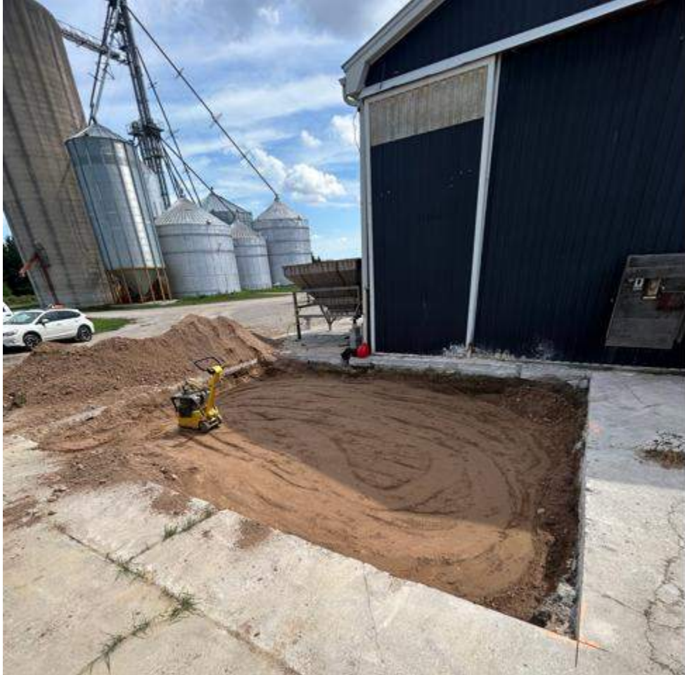
PHOTOGRAPH 5: BACKFILLING IN PROGRESS, (looking southeast)
