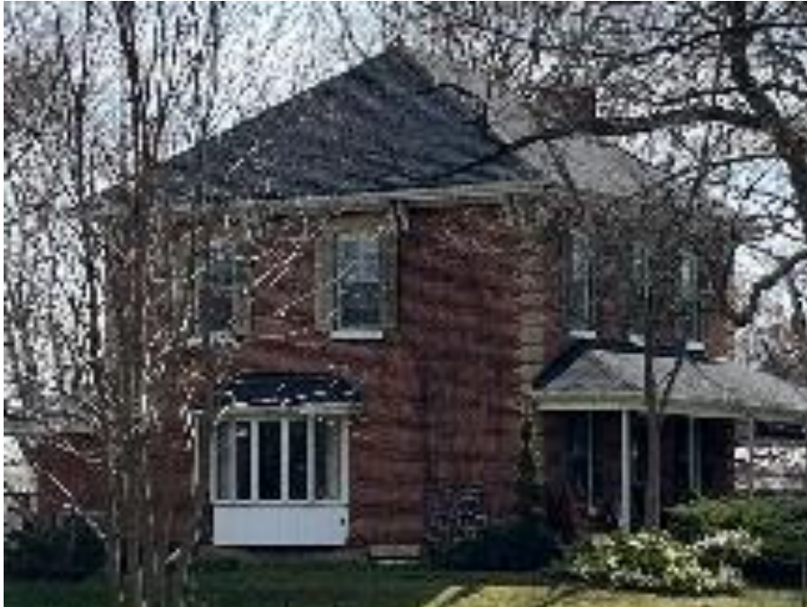
Figure 15: Replacement windows and the bay window on northwest elevation (A.S.I., 2025).
