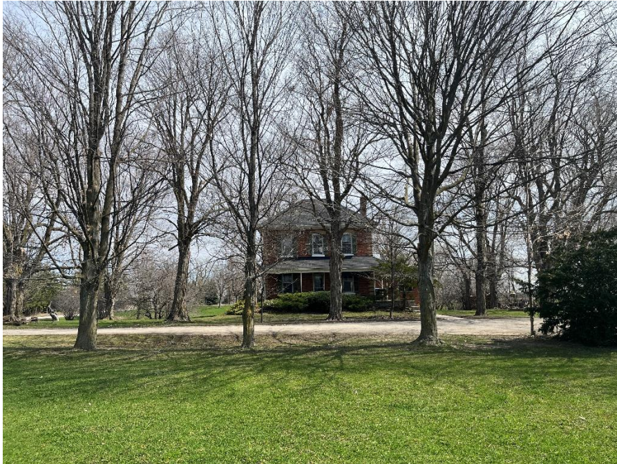
Figure 12: Southwest elevation, facing the primary façade (A.S.I., 2025).
