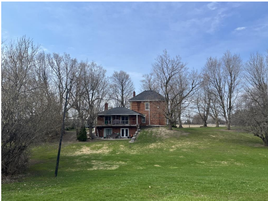
Figure 16: Rear addition on the east corner of the house, from north of the house (A.S.I., 2025).
