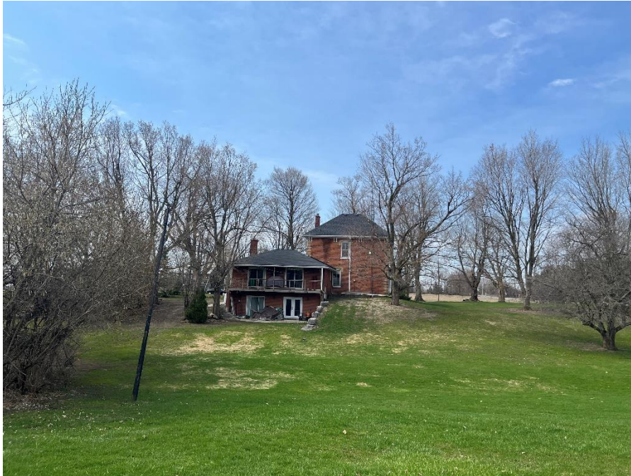
Figure 14: Northeast (rear) elevation from the northern edge of the property (A.S.I., 2025).
