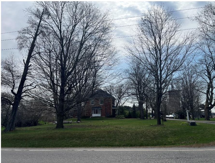
Figure 11: Northwest elevation from Old School Road (A.S.I., 2025).
