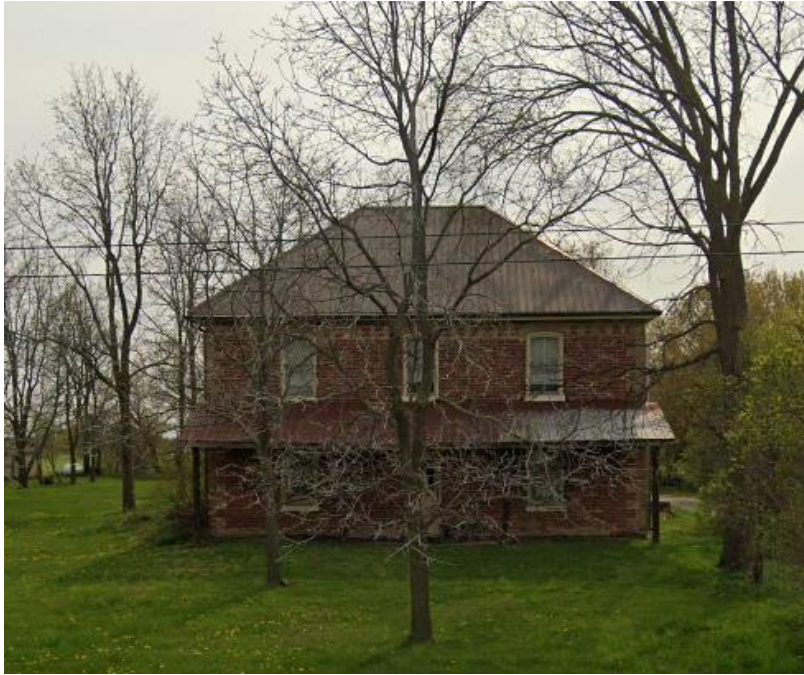
Figure 20: The residence at 14210 Airport Road, looking southwest (Google Streetview, 2023).
