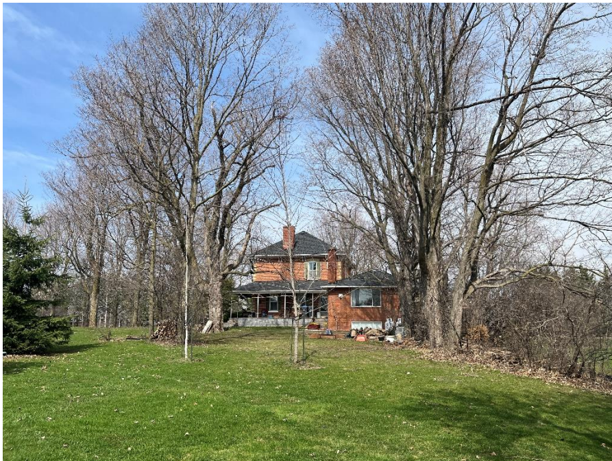
Figure 13: Southeast elevation from the eastern edge of the property (A.S.I., 2025).
