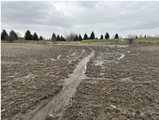
Photo 21 – H20-S1, agricultural swale looking downstream towards Mayfield Golf Club. (2024/03/27)
