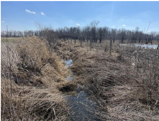
Photo 27 – H25-S1, constructed golf course drainage looking upstream. (2024/03/27)
