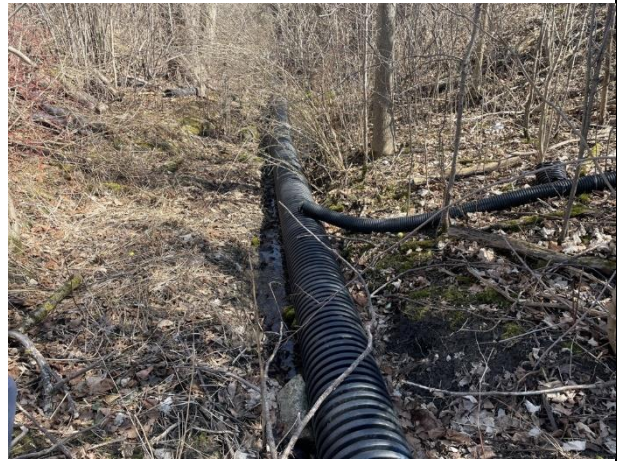
Photo 28 H26-S1, piped golf course drainage looking upstream. (2024/03/27)
