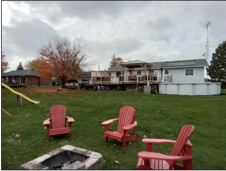
Image 7: Rear view of the residences at 5089 and 5101 Old School Road.
