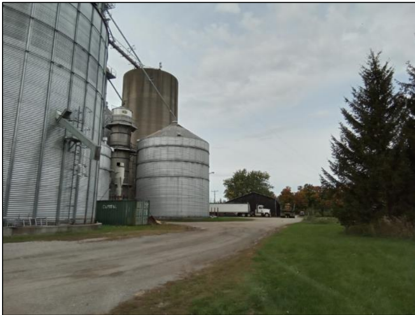
Image 4: View of paved access road, farm buildings and equipment within the farm complex.
