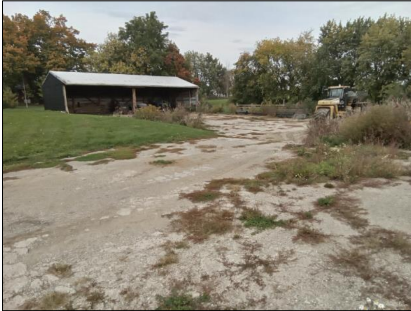
Image 1: View of paved access roads, farm buildings and equipment within the farm complex.
