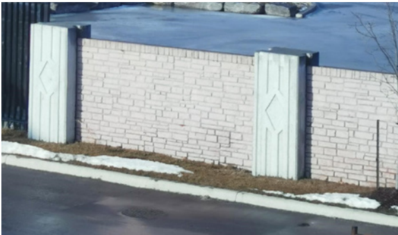
Figure 20: Existing 1.8m HT. Concrete Acoustic Fence
