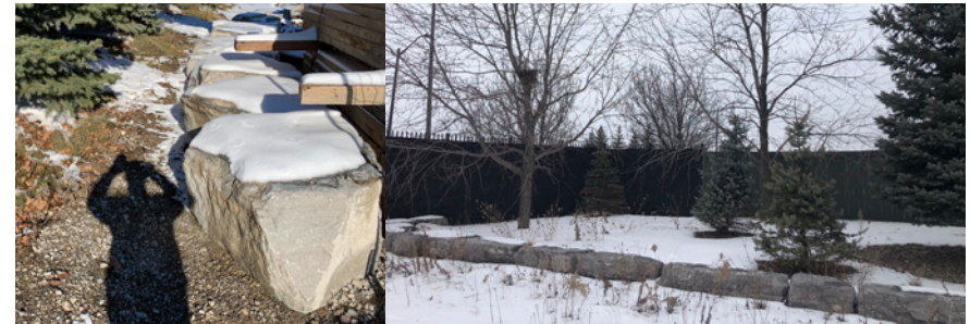
Figure 21: Existing Stone Retaining Wall
