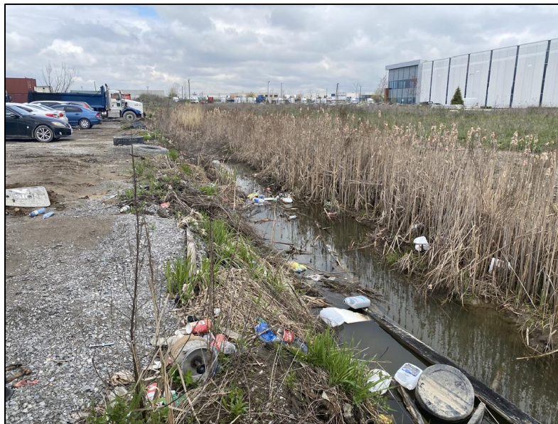
Photo 2: Fill and garbage along west bank, dense vegetation in the channel along east bank (photo taken facing upstream, north, May 2023).
