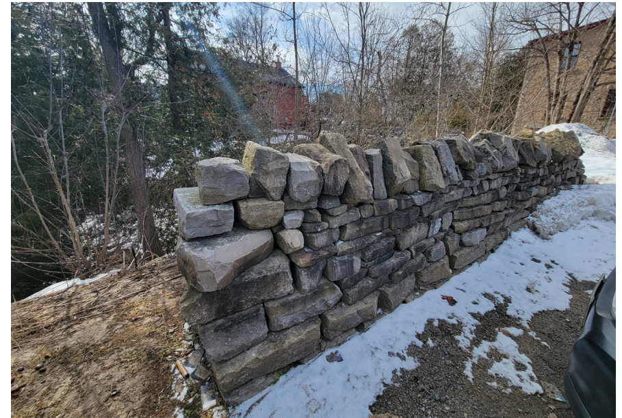
DRY STONE WALL AT THE ALTON MILL CENTRE FOR TH
