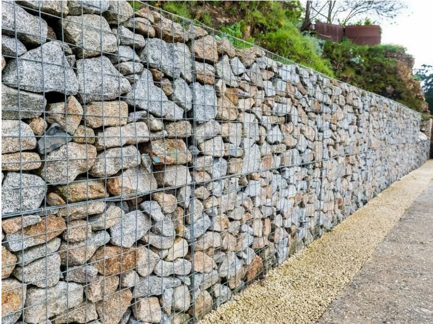
GABION STONE RETAINING WALL
