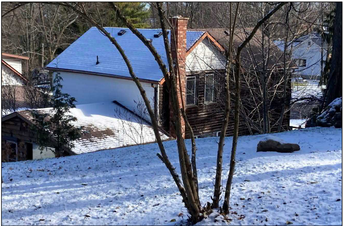
Photograph 20: West and north façade of 46 Amelia Street
