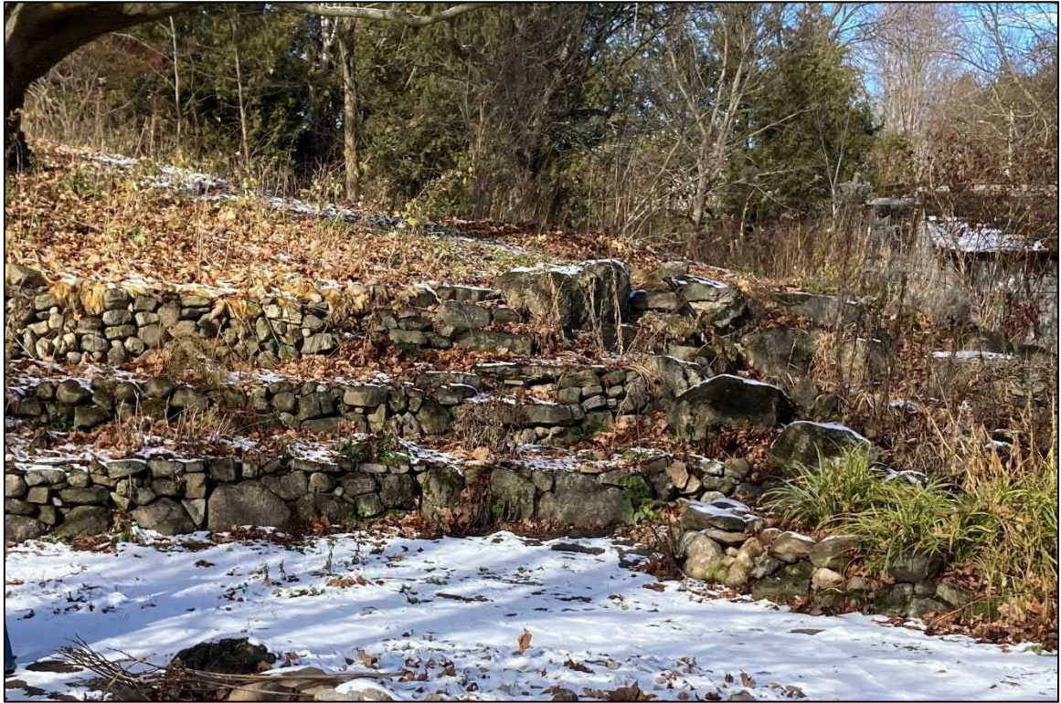
Photograph 25: Terraced drystone retaining wall west of the house at 19876 Main Street
