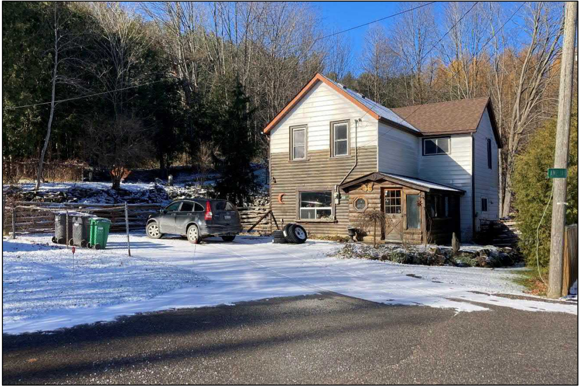
Photograph 19: Main and east façade of 46 Amelia Street
