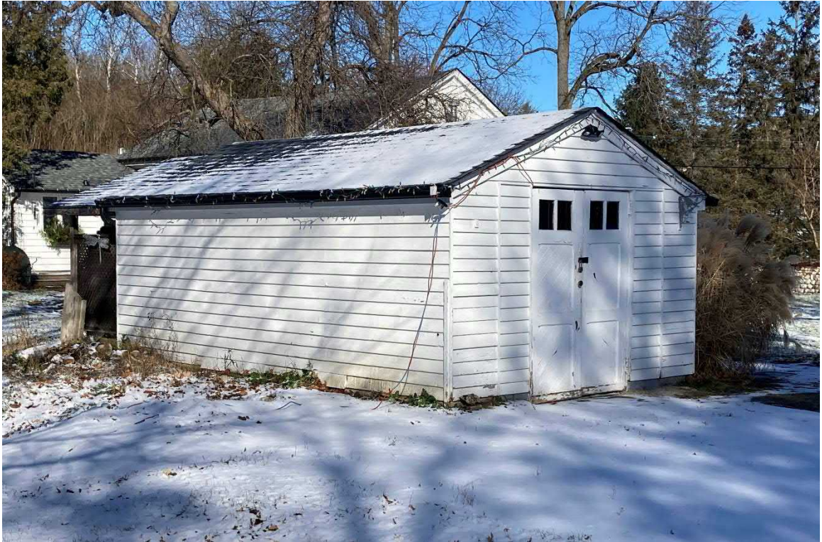
Photograph 31: One-storey garage at 19876 Main Street
