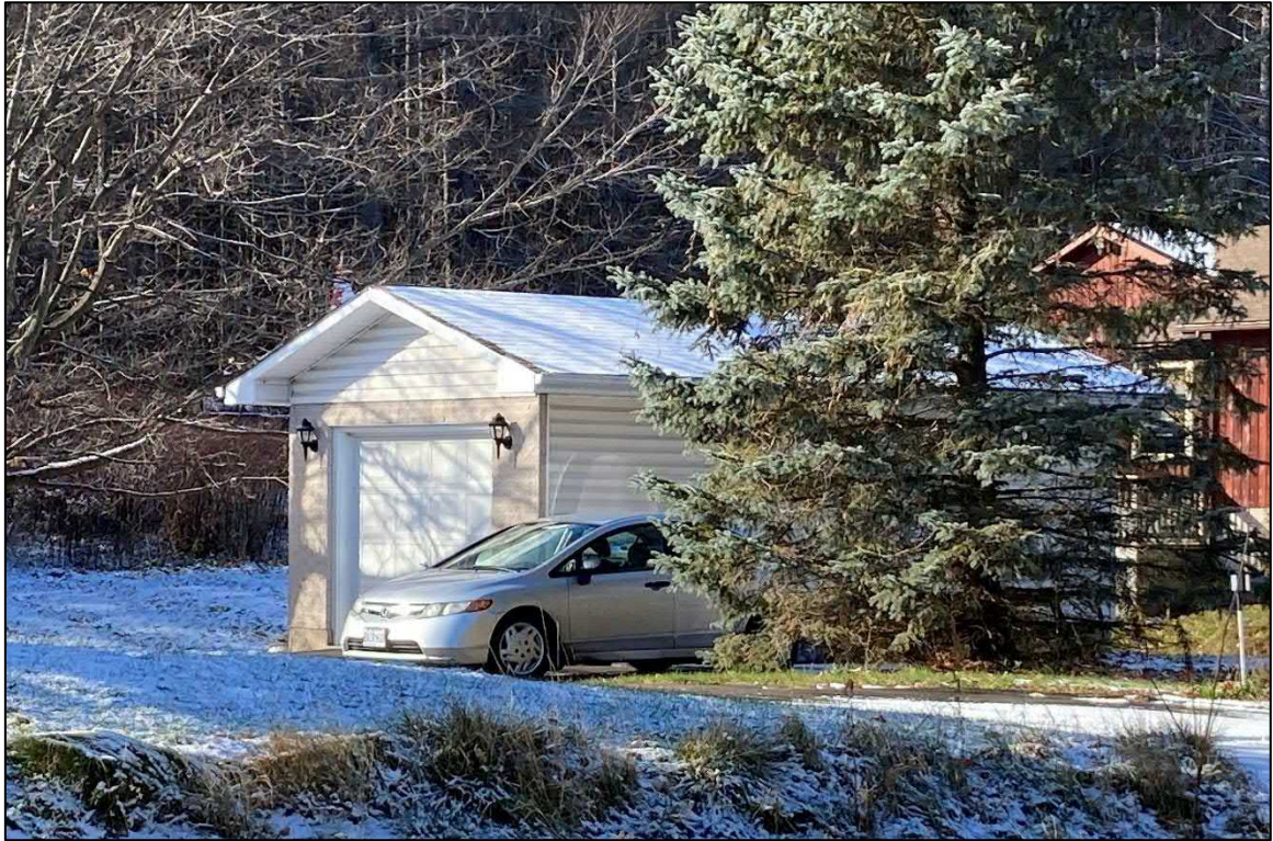
Photograph 37: Modern garage at 19904 Main Street
