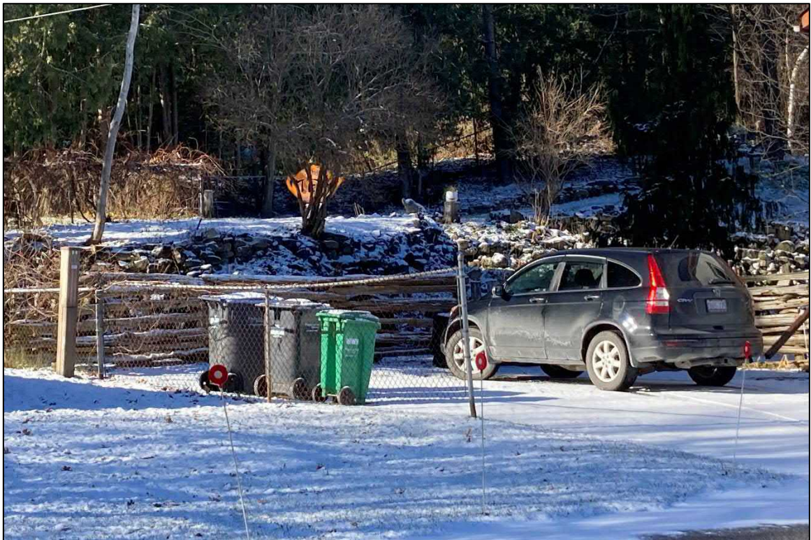
Photograph 18: View to northwest of terraced drystone retaining walls at 46 Amelia Street
