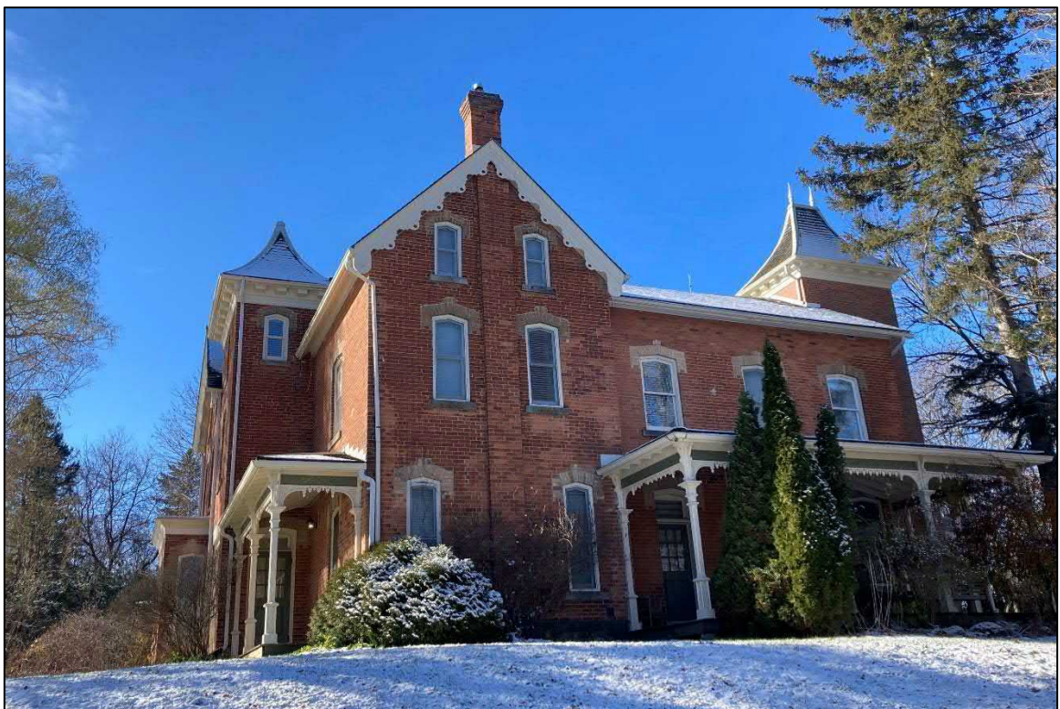
Photograph 14: Three-quarter view of the main and east façades of the Wards-Dods-Millcroft house
