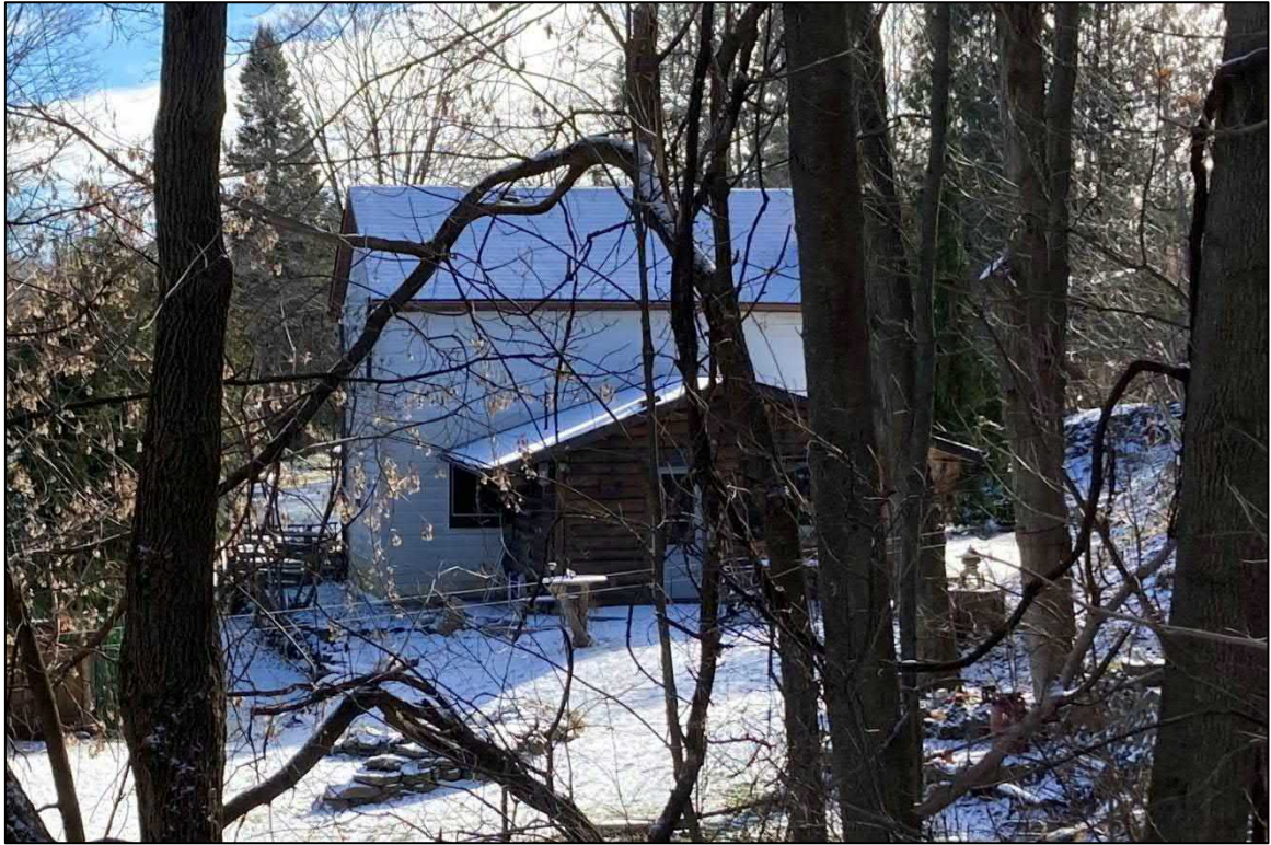
Photograph 21: North (rear) façade of 46 Amelia Street
