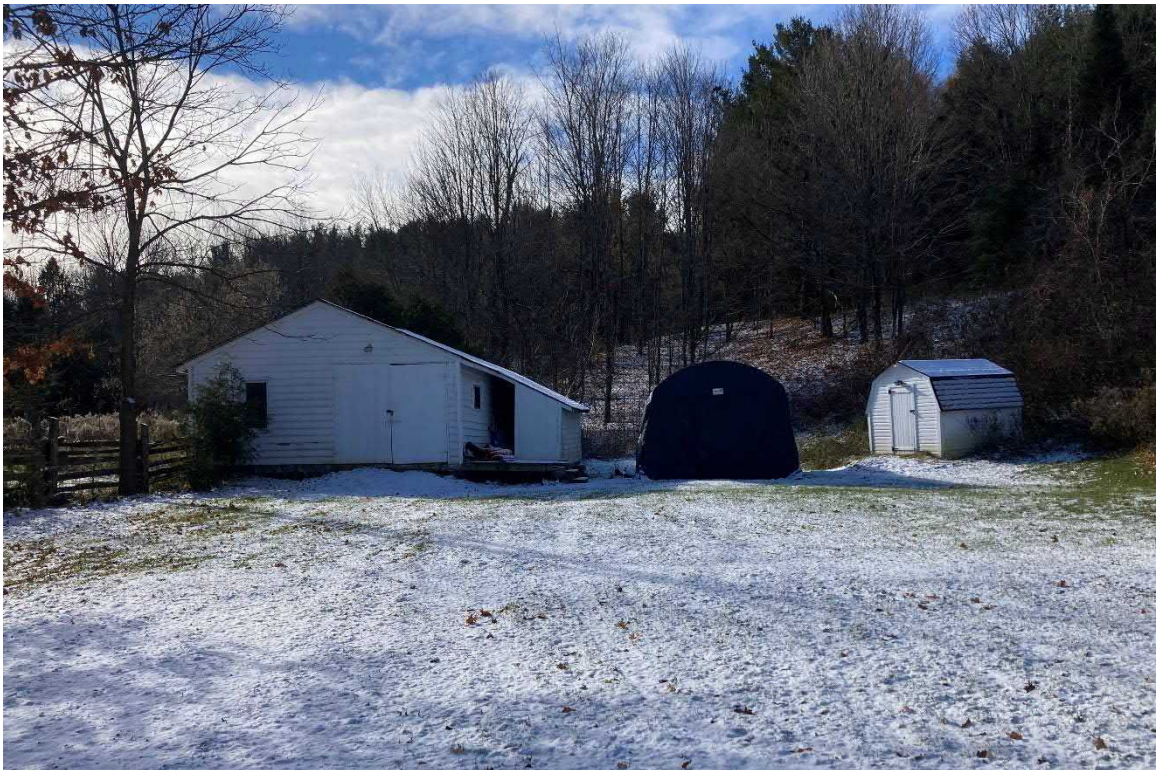
Photograph 32: Barn and shed at 19876 Main Street
