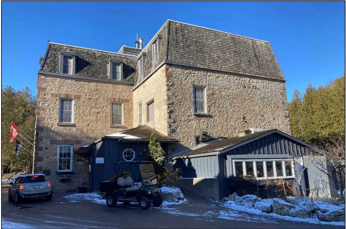
Photograph 9: East façade of the mill
