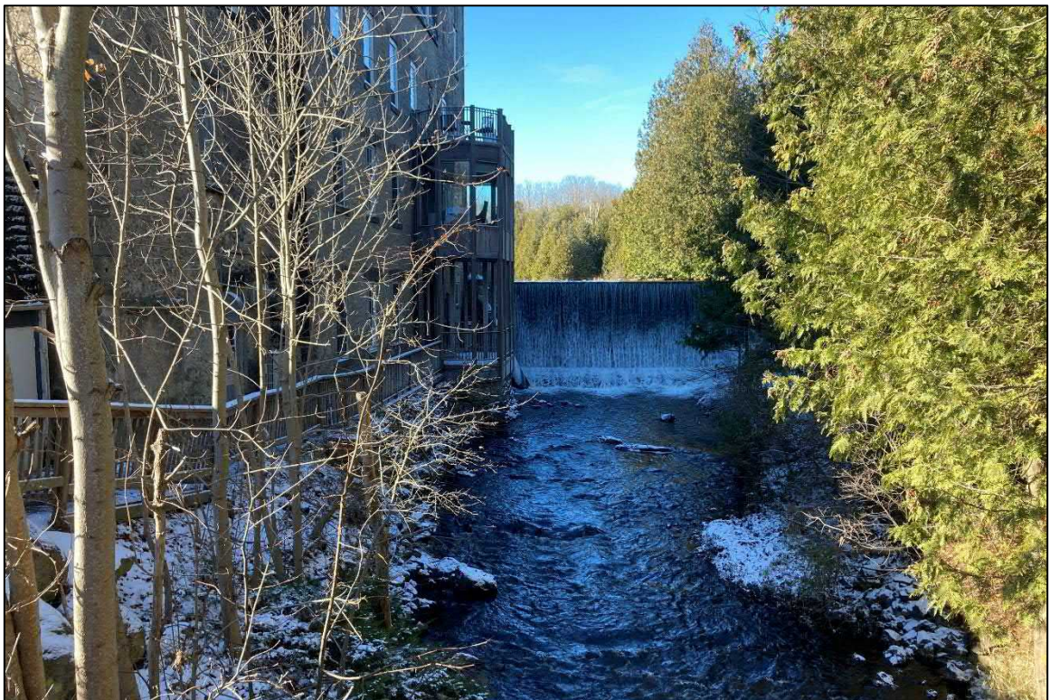
Photograph 6: View to Shaw's Creek (mill building on left)
