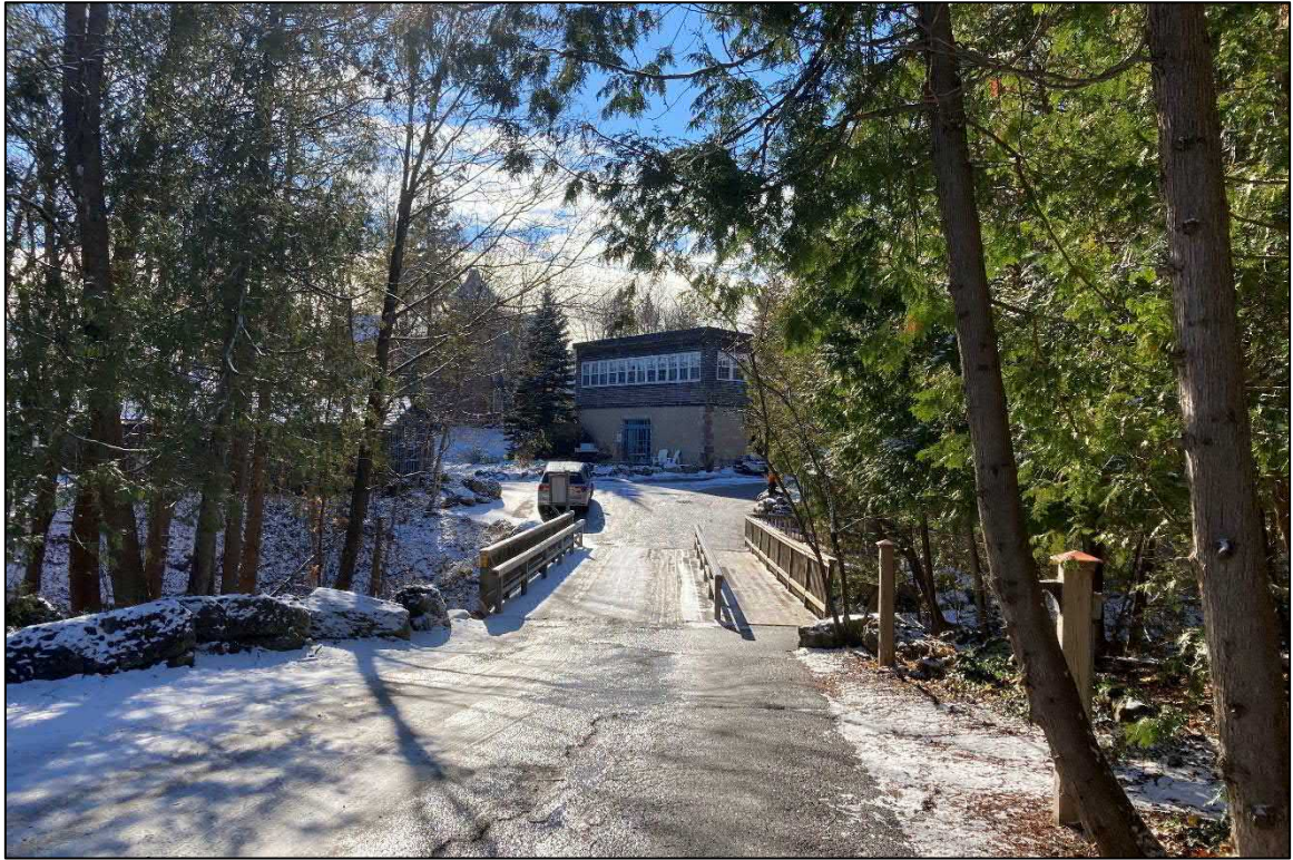
Photograph 5: View of bridge over Shaw's Creek
