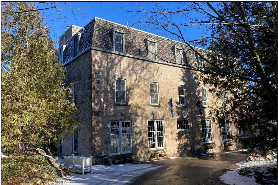
Photograph 8: West façade of the Mill
