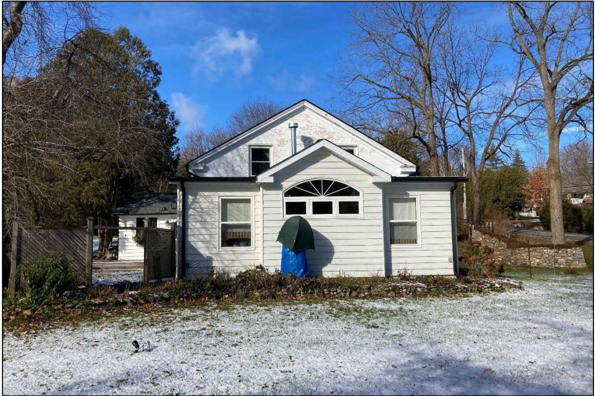
Photograph 29: South façade of 19876 Main Street
