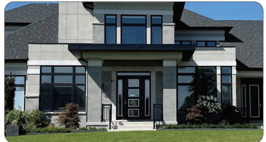
Large covered front entry features are encouraged
