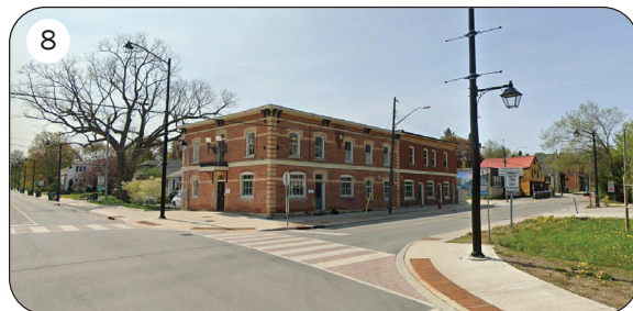
View around the intersection of Main Street and Queen Street W.
