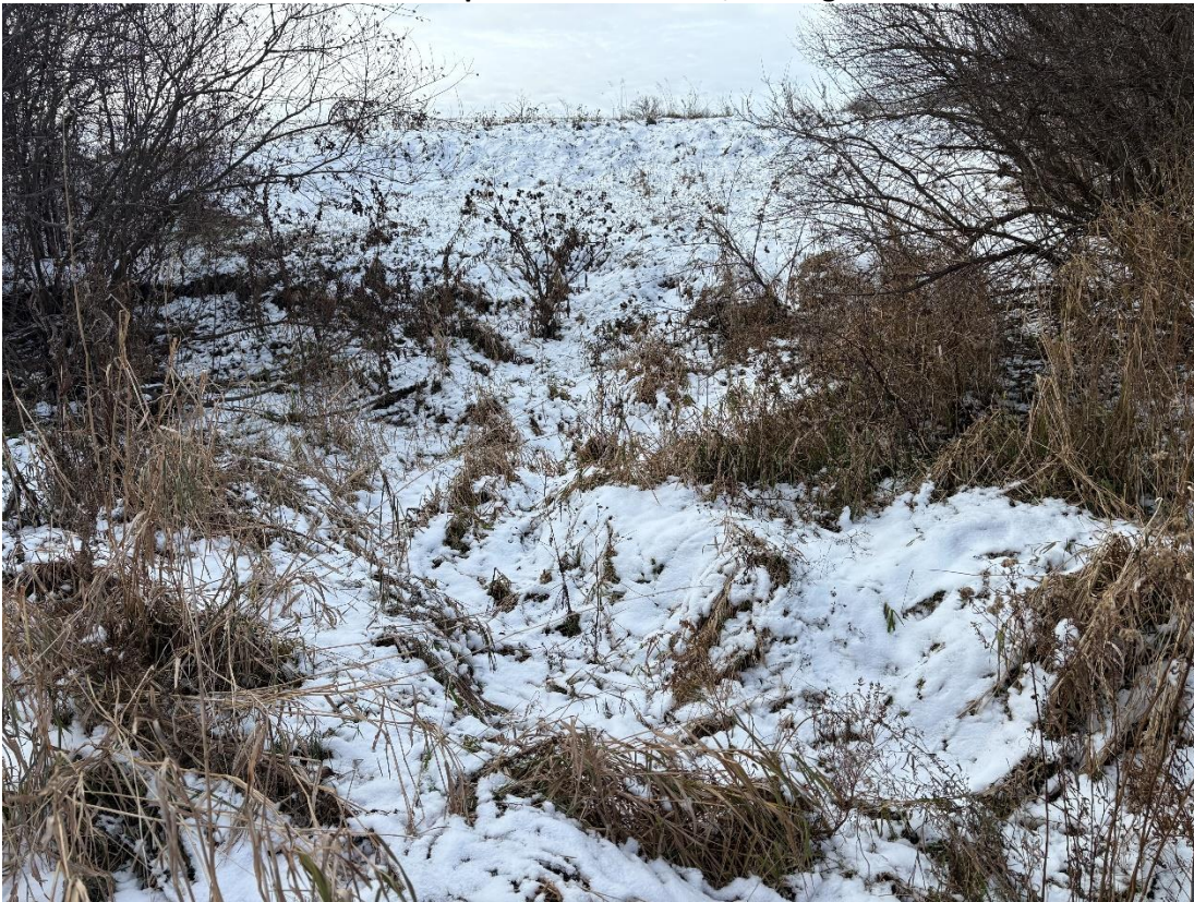
Photo 4: Slope Near Section 4-4, looking East
