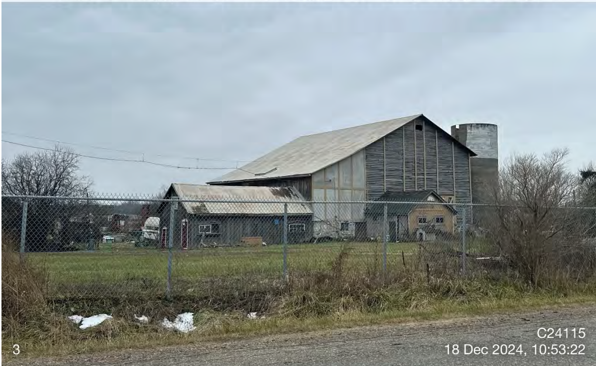
Photo 8: Operation #9 – Unoccupied livestock facility, former dairy operation.
