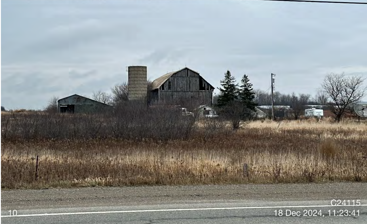
Photo 9: Operation #12 – Remnant farm with uncapped silo and bank barn in poor condition, missing boards in loft.
