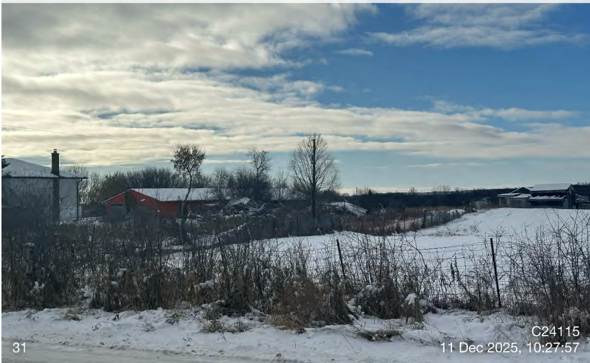
Photo 14: Operation #31 – Remnant farm, agricultural structures demolished, garage and residence remaining.
