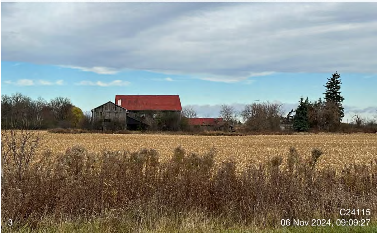
Photo 2: Operation #3 – Remnant farm, wooden bank barn in poor condition.
