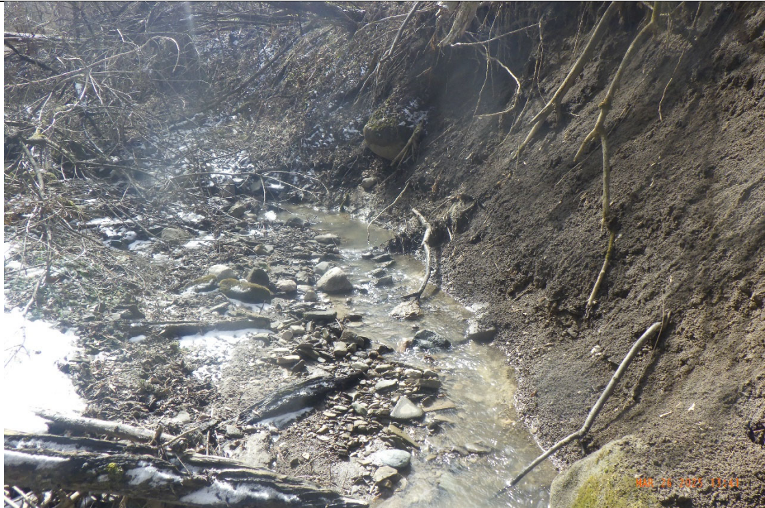
Exposed clay was noted throughout the channel, increasing in frequency upstream. Channel bed morphology was primarily comprised of riffles, with few deep pools. Measured riffle lengths were between 8.40 and 11.20 m.
