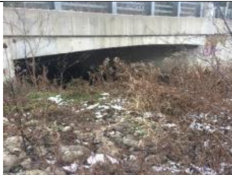
Downstream Culvert Face
