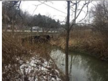
Downstream Bridge Face
