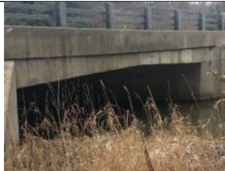
Downstream Bridge Face
