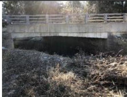
Upstream Bridge Face
