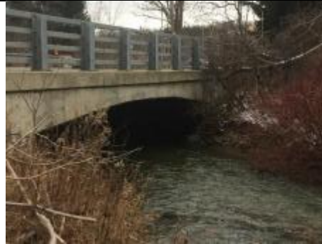
Upstream Bridge Face
