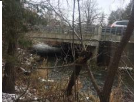
Upstream Culvert Face
