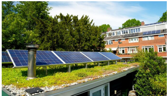
Rooftop solar panels and green roof integration
