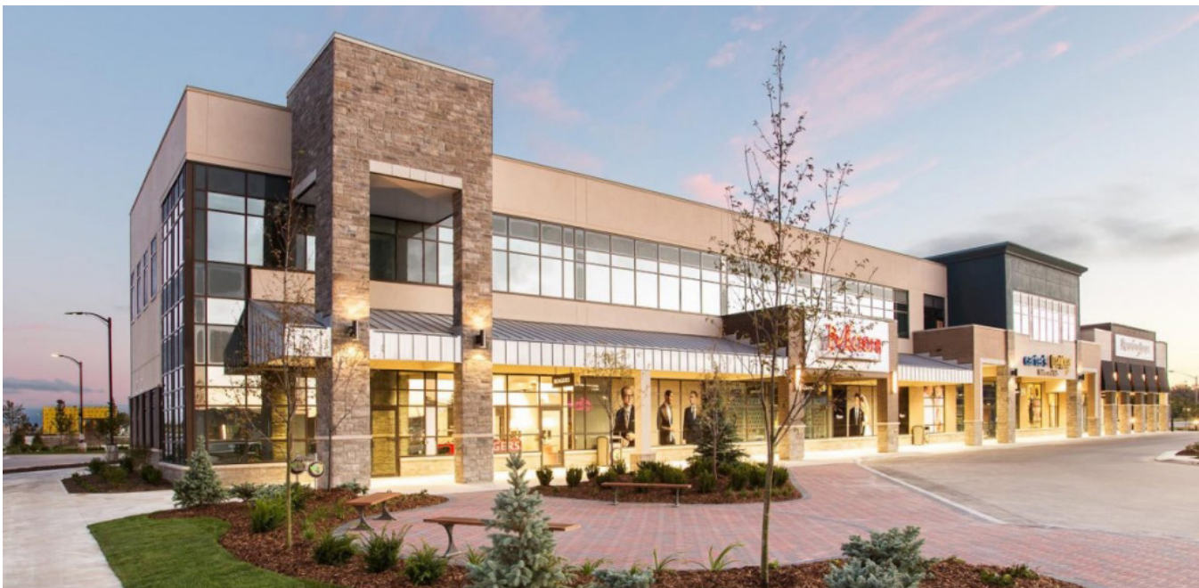
Commercial built form with active storefronts, articulated façades and landscaped open space
