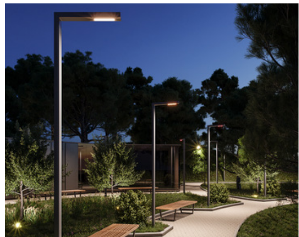
Down-directed pedestrian lighting along trails and open spaces
