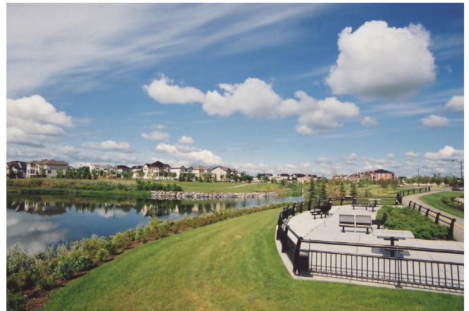
Integrated walkway and viewing area along stormwater pond
