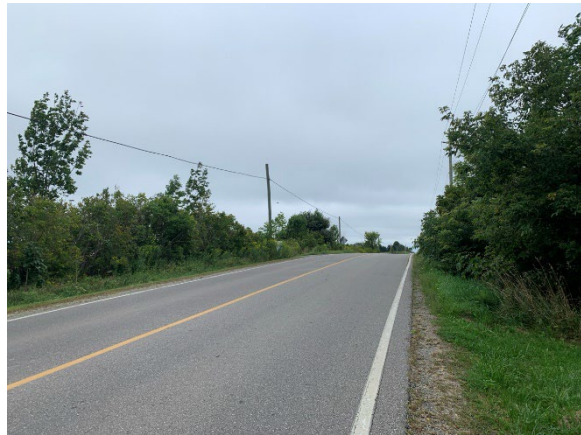
Photo 2: Mount Hope Road, looking south
