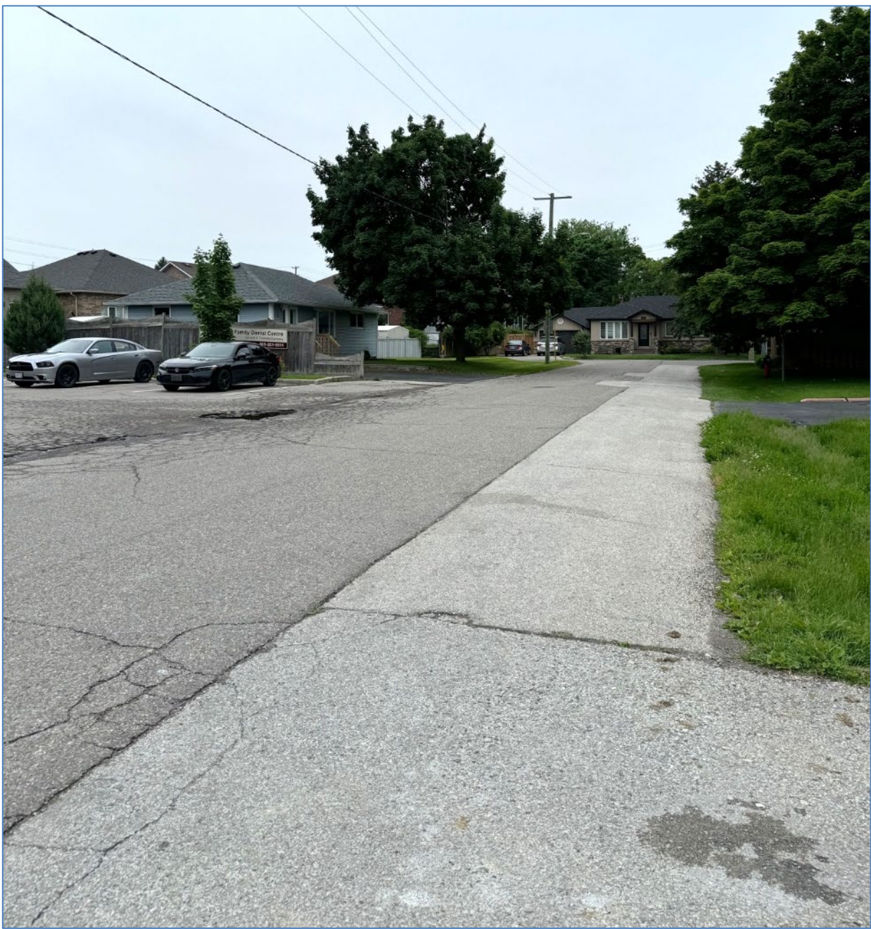
Shore Street at Site Access – Looking West
