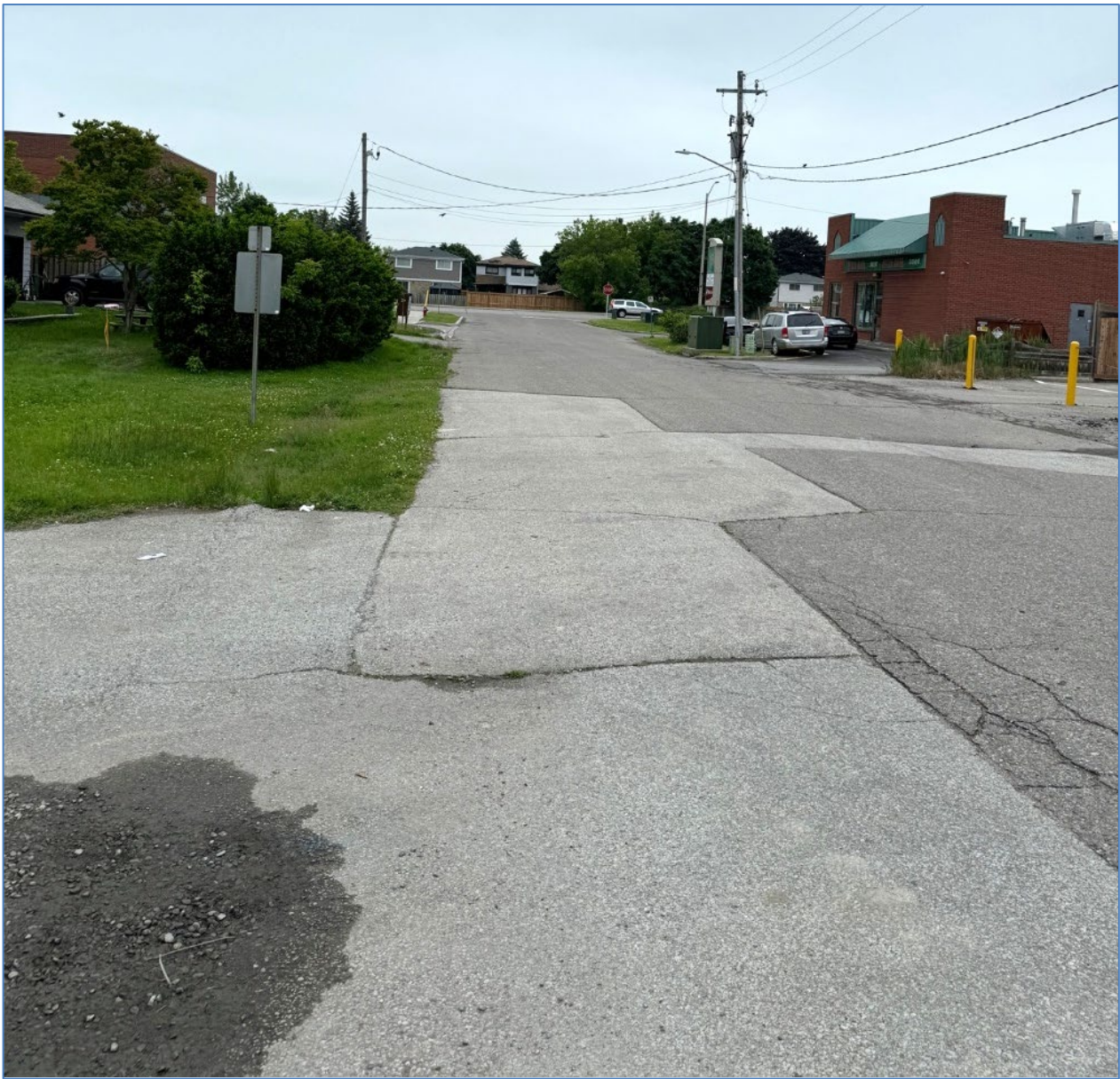
Shore Street at Site Access – Looking East
