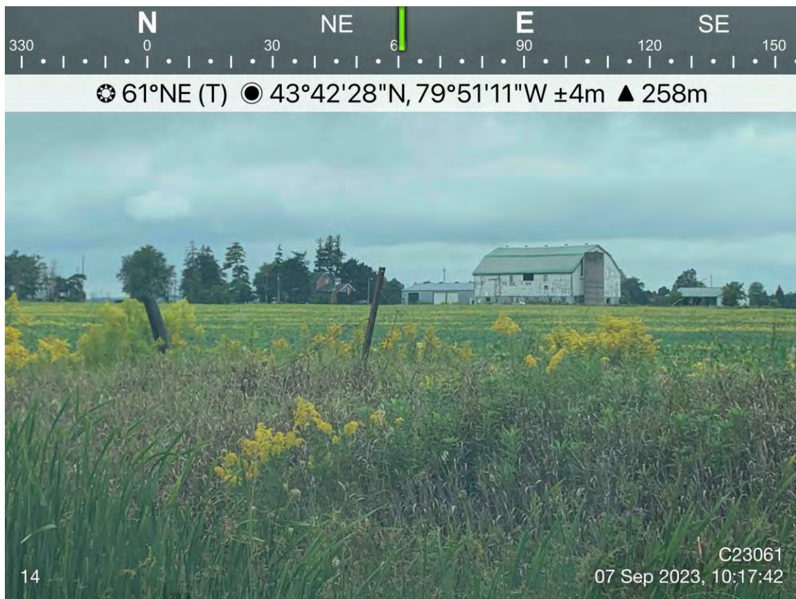
Photo 10: Operation #14 - Remnant farm showing uncapped cement silo, implement shed, and barn in poor condition.
