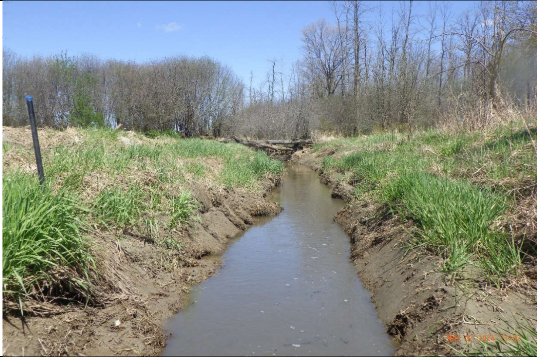
One localized area in the downstream portion of the reach showed evidence of recent dredging (sloped bare banks).
