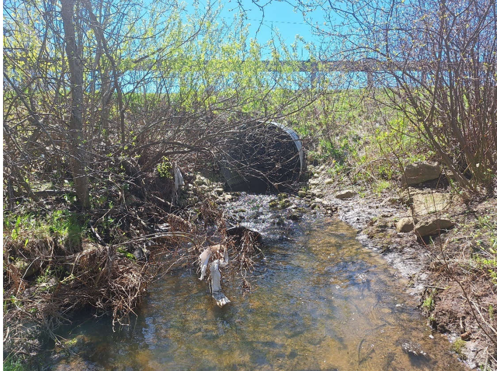
The reach was run-dominant with a lack of riffle pool morphology. One artificial riffle was identified at the culvert at Creditview Road.
