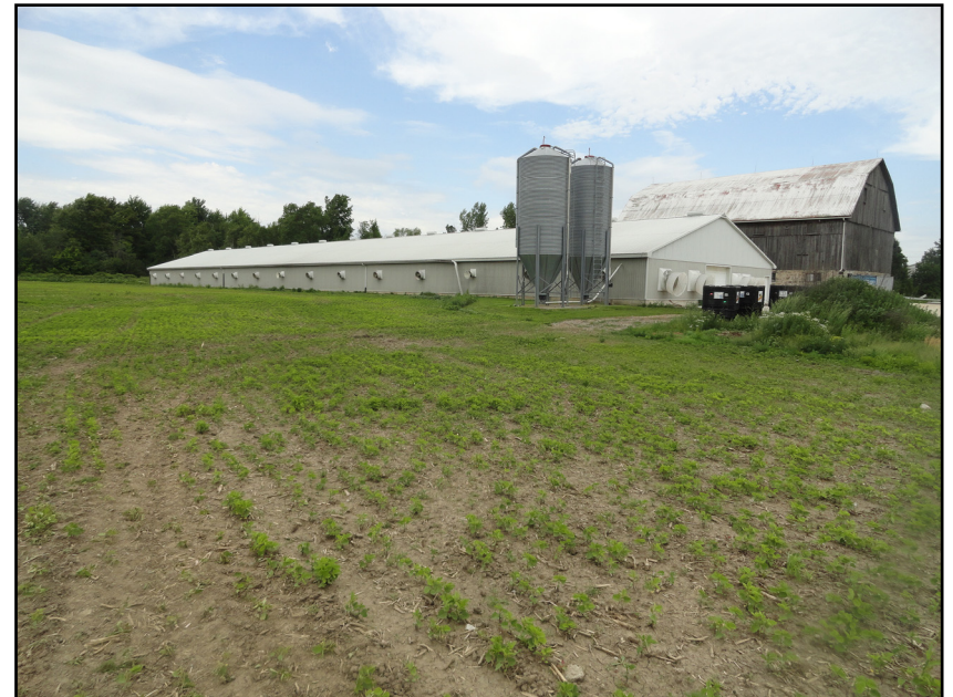
Photograph 32. Agricultural Buildings (IAGM1)
