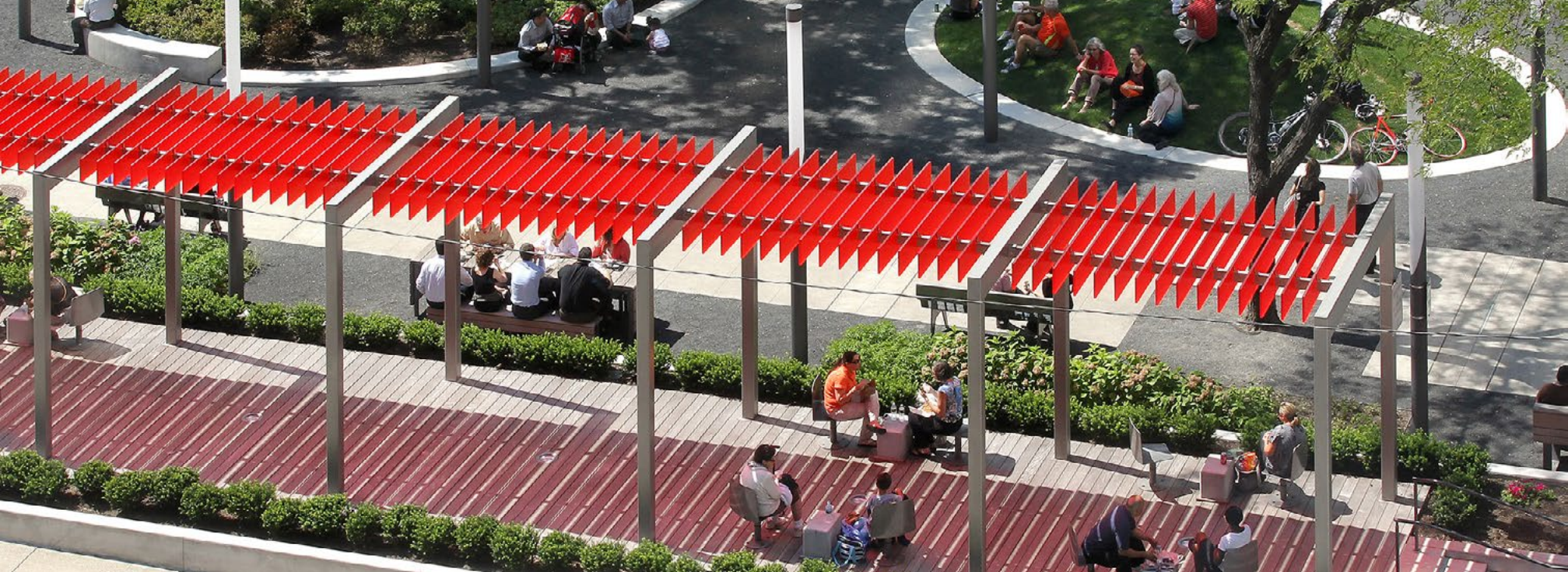
Example of a shade structure that is designed to be a focal element of the park
