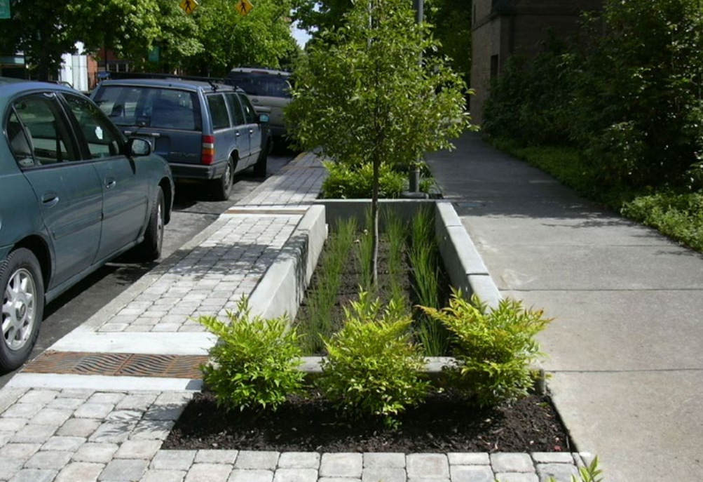
Street level stormwater retention
