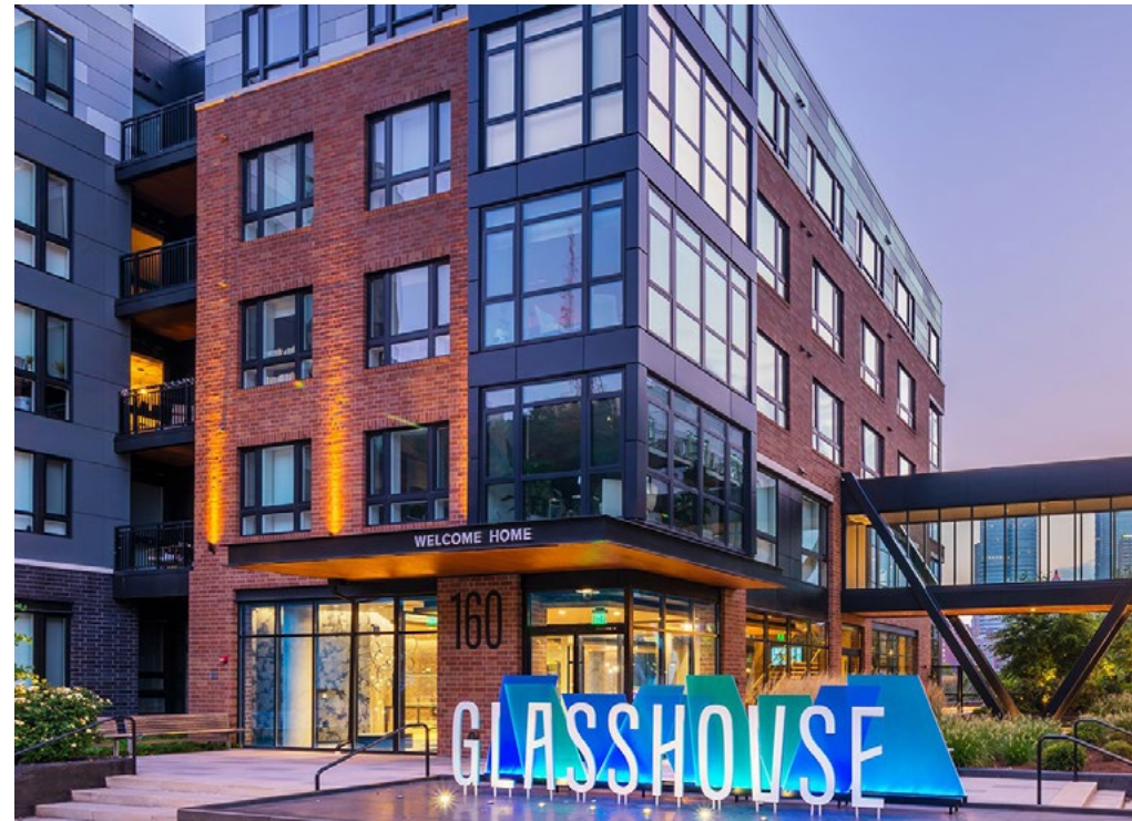
Examples of mid-rise buildings
