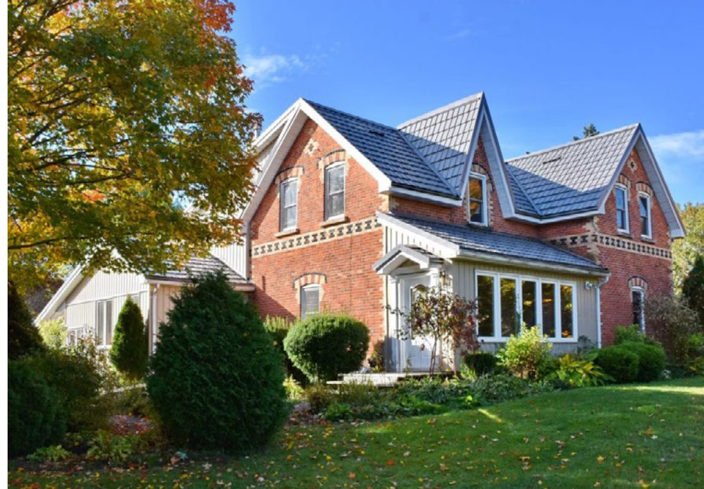
Gothic Revival Style with steeply pitched front gables
