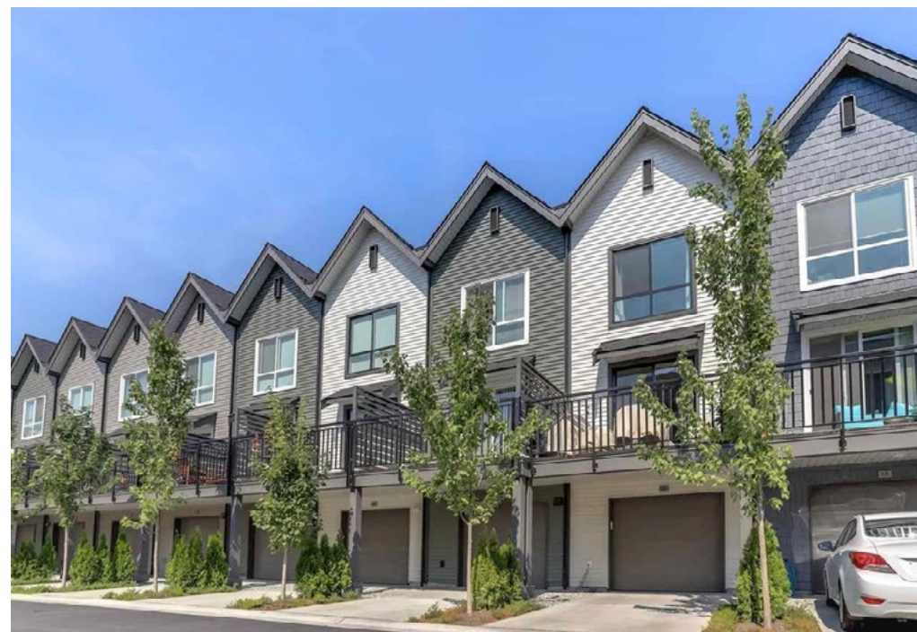
Outdoor amenities for lane-based townhouses may include conventional rear yards with detached garages or raised terraces/ balconies with integrated garages.
