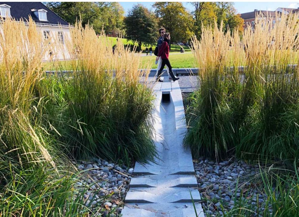
Lot level stormwater retention
