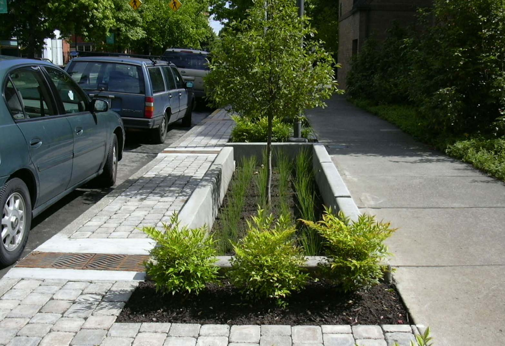
Street level stormwater retention
