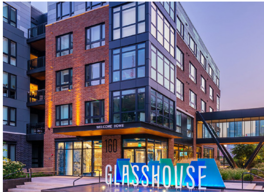
Examples of mid-rise buildings
