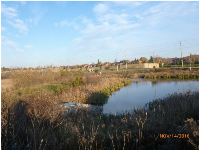
Figure 3.3 Outlet Structure – Looking Southwest
