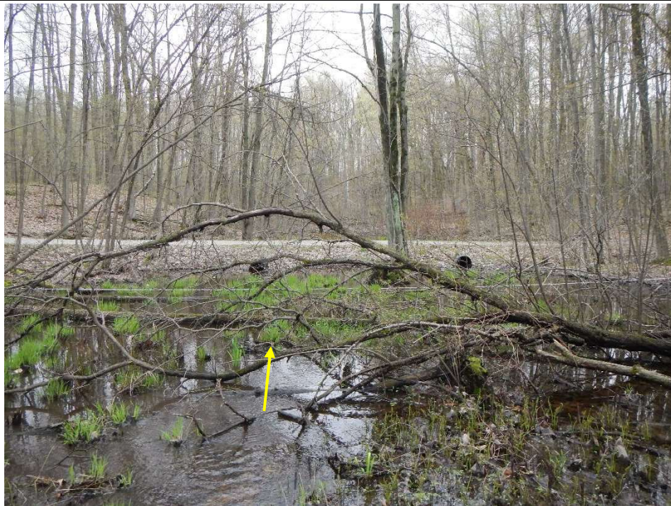
Photo taken facing downstream towards tail crossing, near the downstream extent of the detailed assessment.
