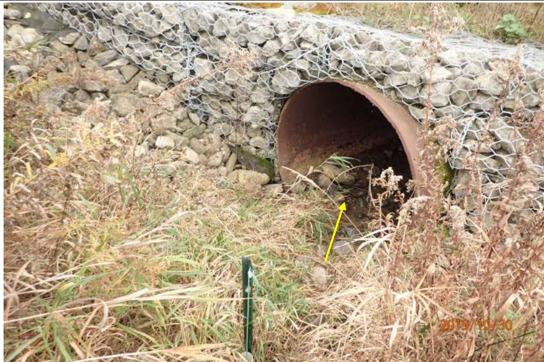
Photo taken facing downstream showing baseline conditions.
