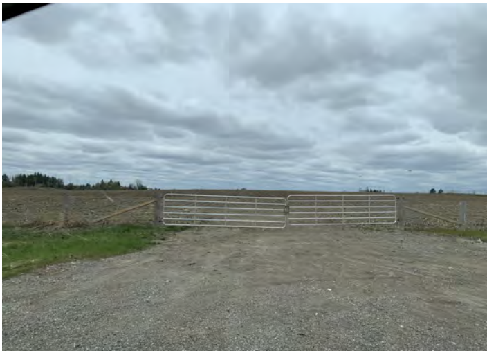
PHOTO 1: View of the front entrance of the property located at 12414 Kennedy Road in Caledon, ON
